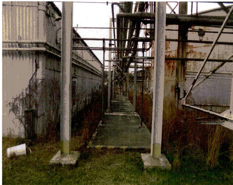
Figure 4: Building 483-3D Ancillary Cable Trench and Pipe/Conduit Bridge
