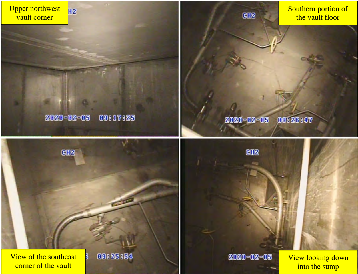
Figure 2.4-2: Views of the FDB-5 Vault Interior
