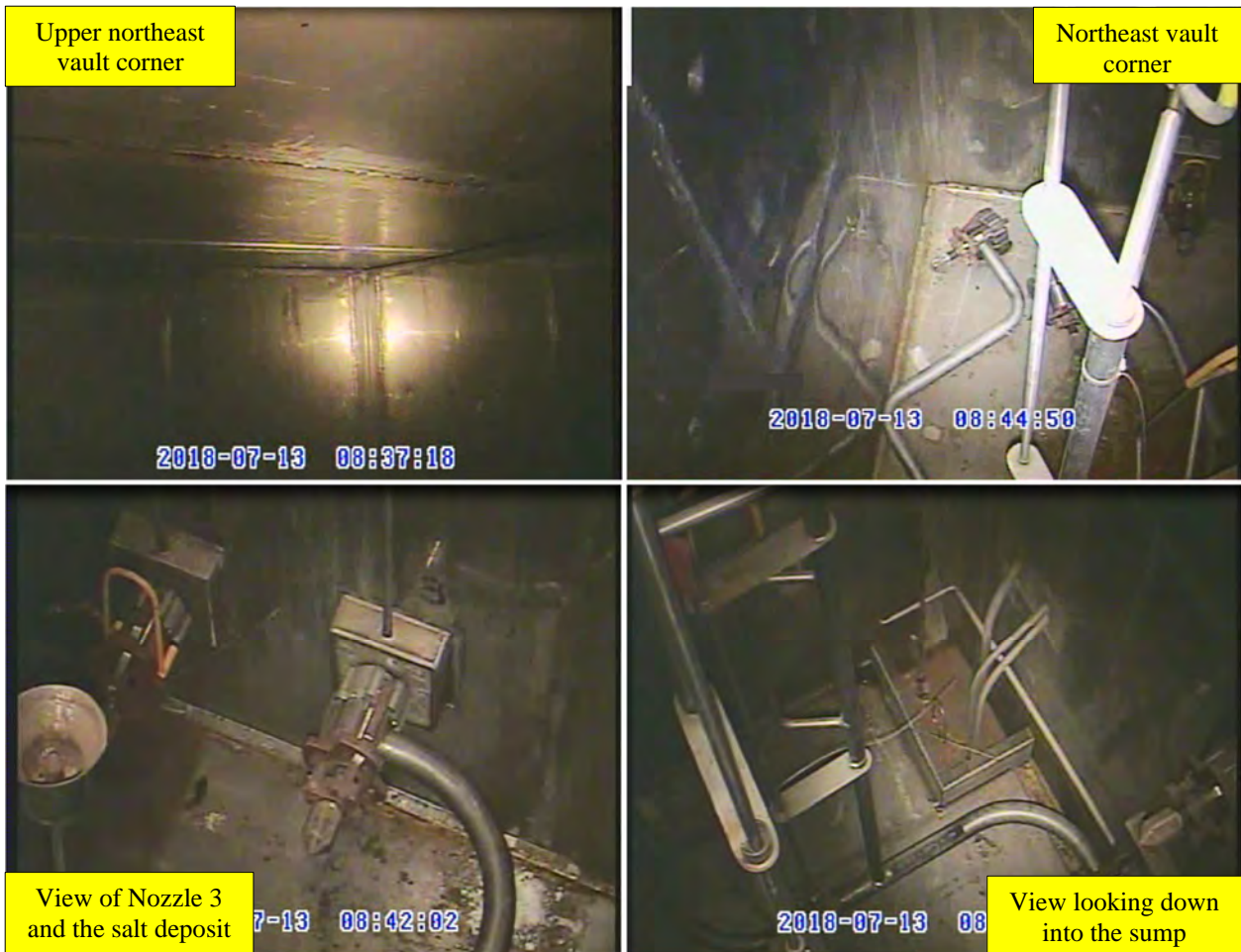
Figure 9.0-2: Views of the FDB-6 Vault Interior
