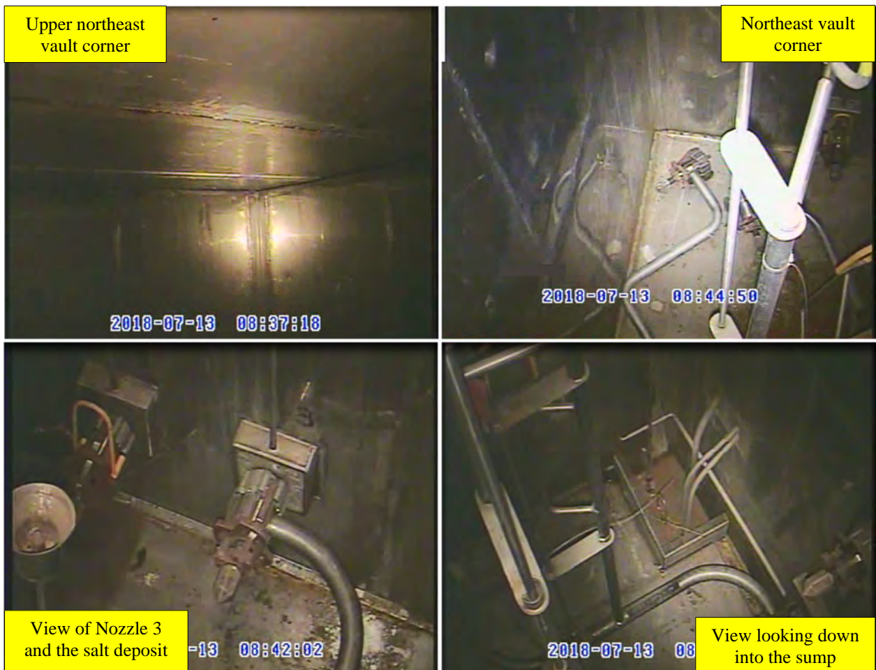
Figure 2.8-1: Views of the FDB-6 Vault Interior
