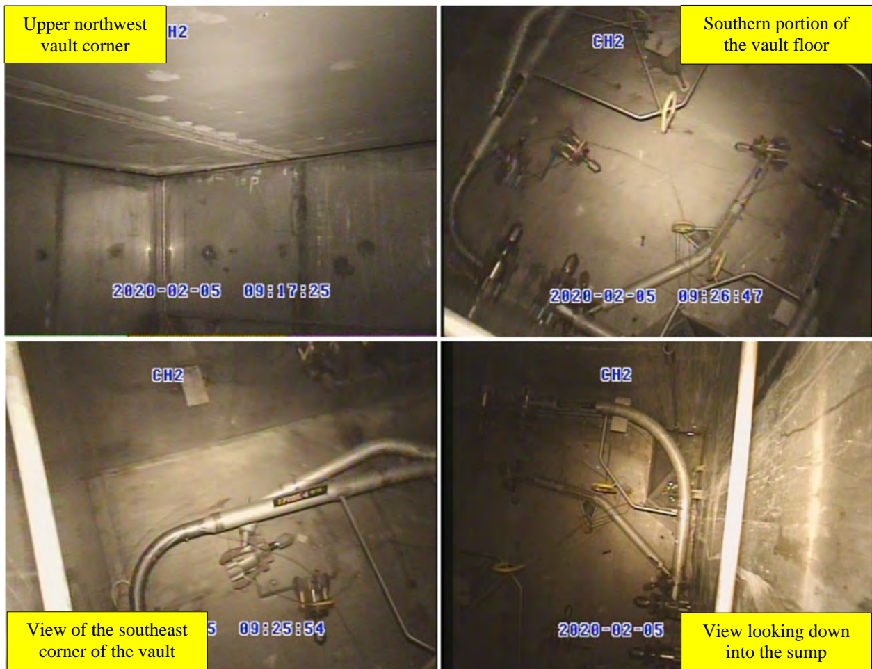
Figure 9.0-1: Views of the FDB-5 Vault Interior
