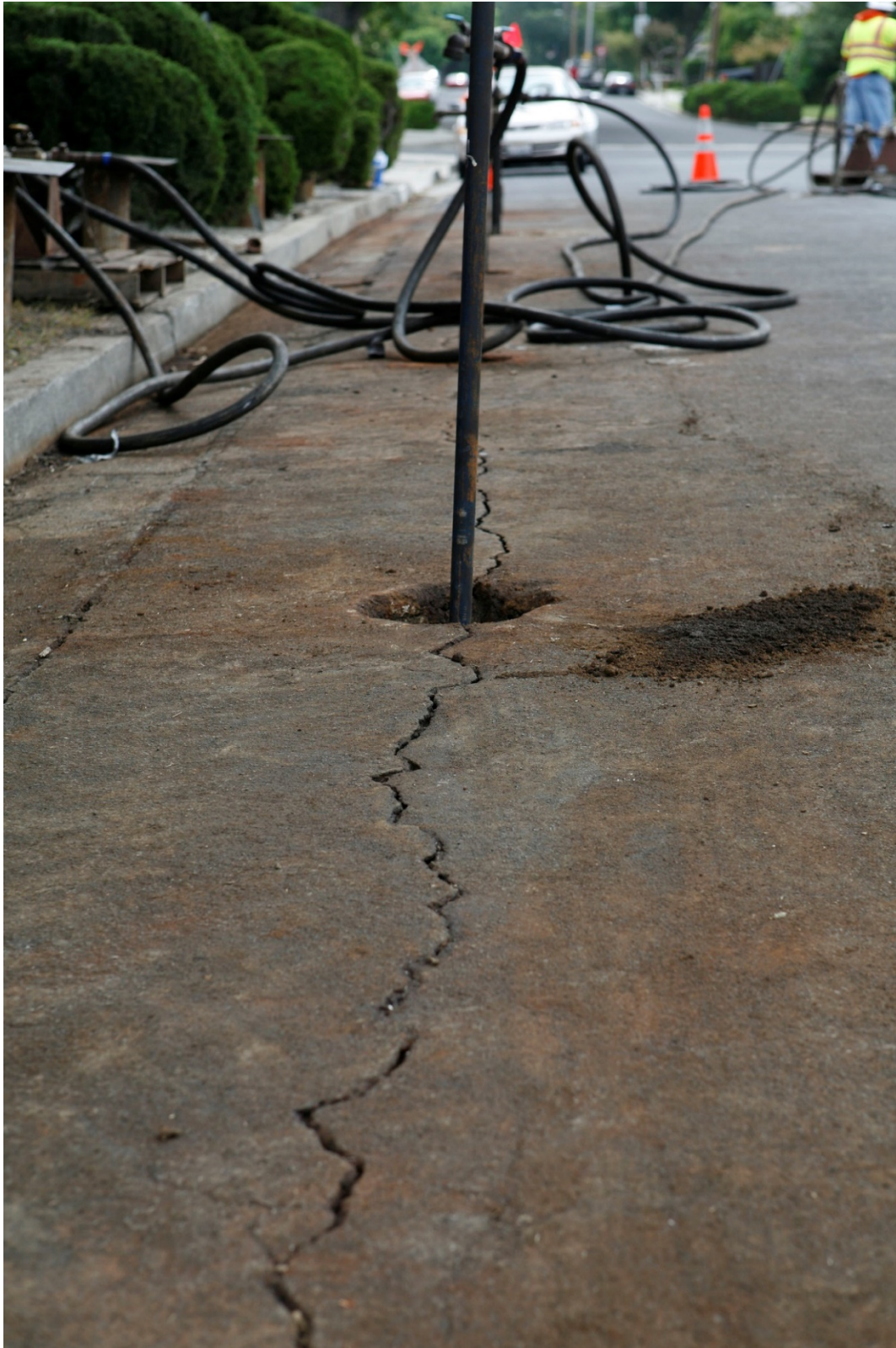
Figure 15. Demonstration of Fracture Along Alignment of PRB
