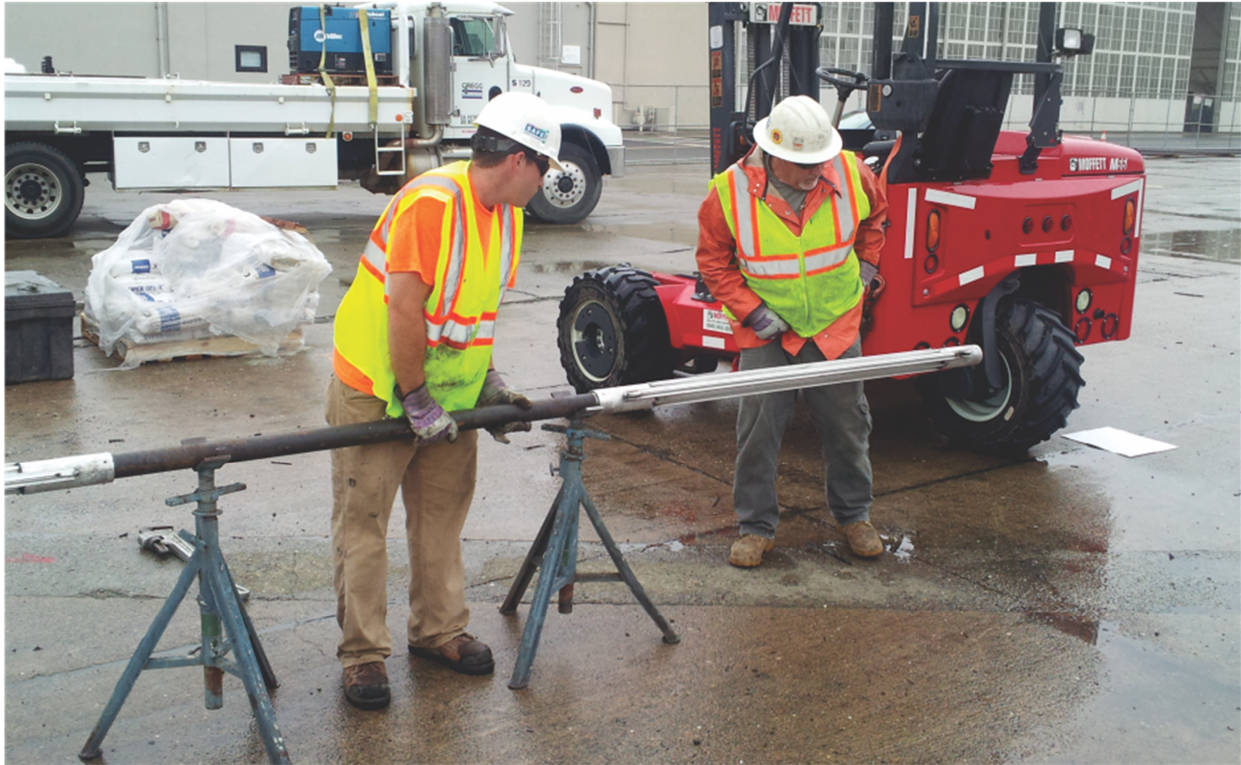
Figure 13. Preparing Expansion Casing System for Installation
