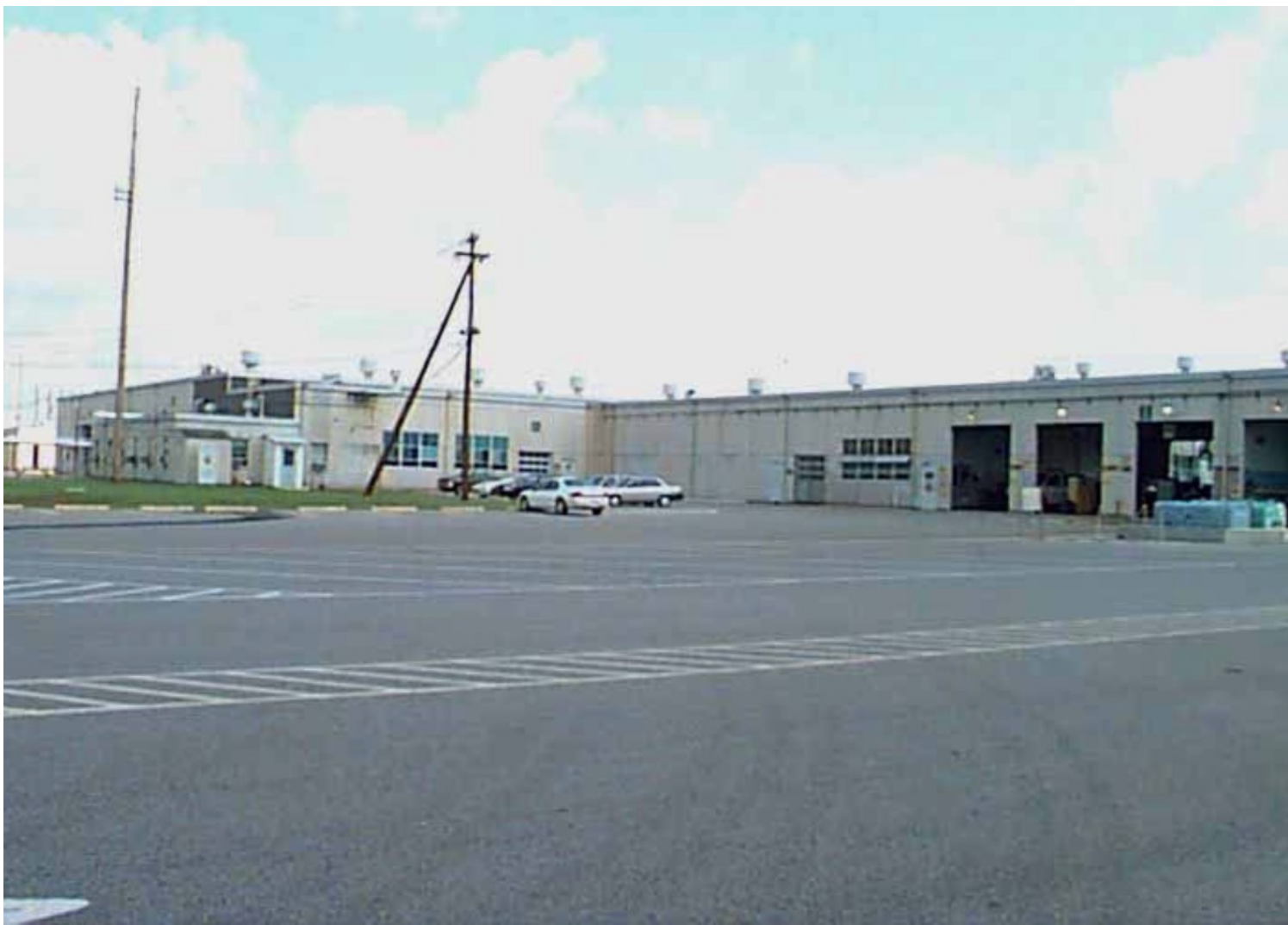
Figure 8. Building 716-A, Before Decommissioning
