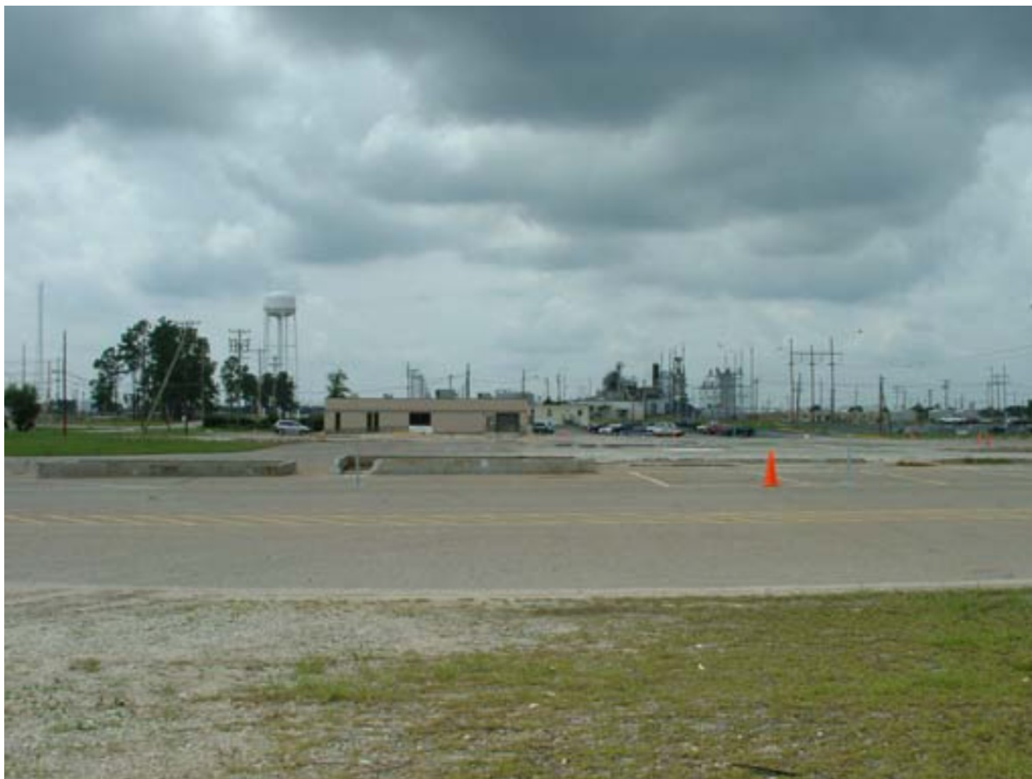
Figure 9. Building 716-A Remnant Slab, After Decommissioning
