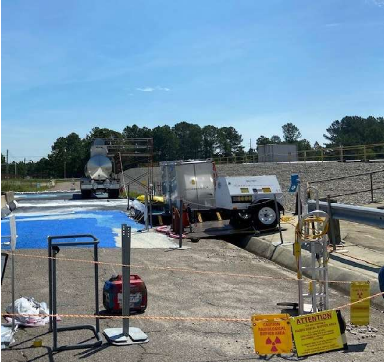
Above: Tuff tanks and area coated on 7/5/22 to fix contamination (coating colors have no specific meaning, facility used the colors that were available). Photo taken 7/7/22.
