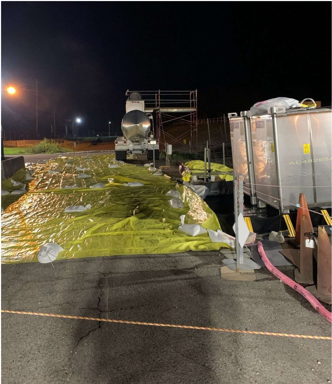
Above: Paved spill area tarped. Photo taken in the early morning hours of 7/5/22.
