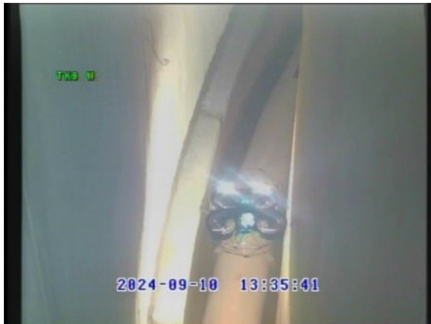
Figure 4 - Tank 9H Annulus Drone Inspection
