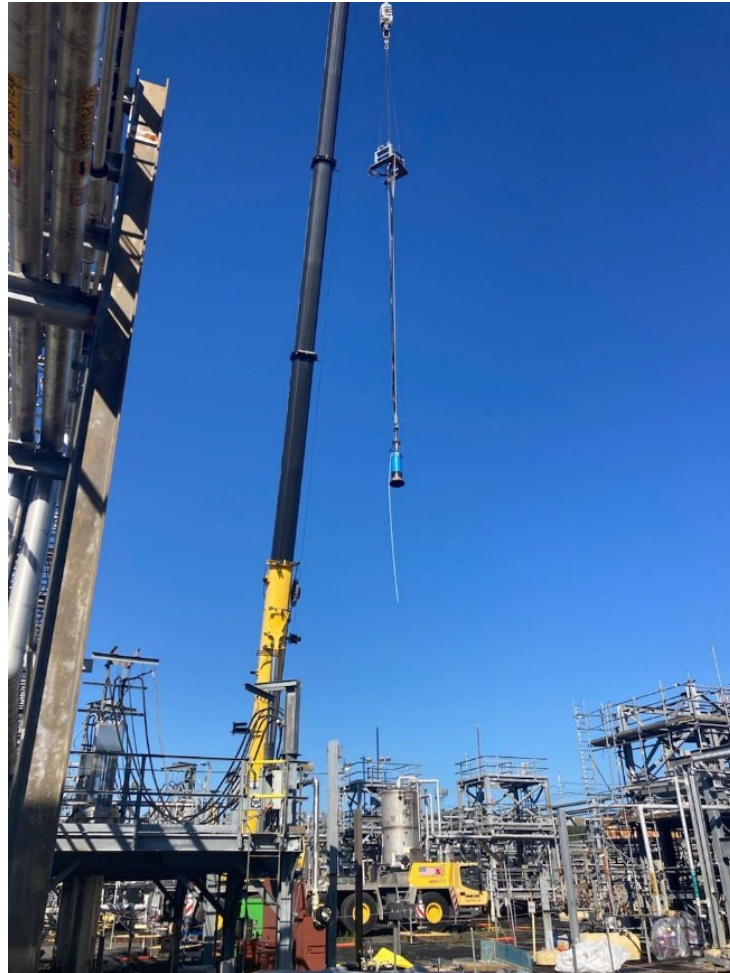
Figure 2 - Tank 4F Dewatering Pump Installation
