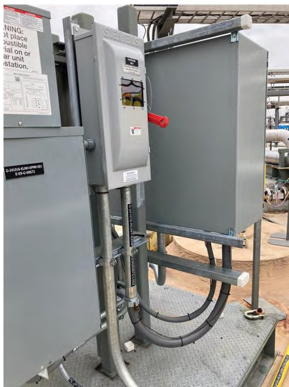
Figure 14 - Tank 31H Gas Release Mode Input Disconnect
