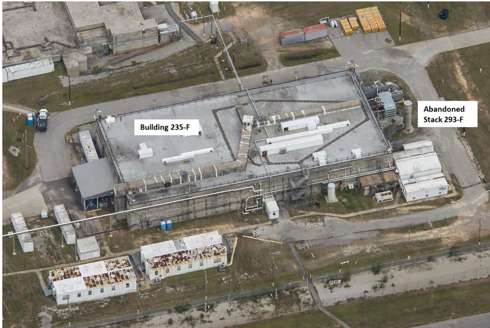
Figure 9. Photograph of Height Reduced Abandoned Capped Stack (293-F)
