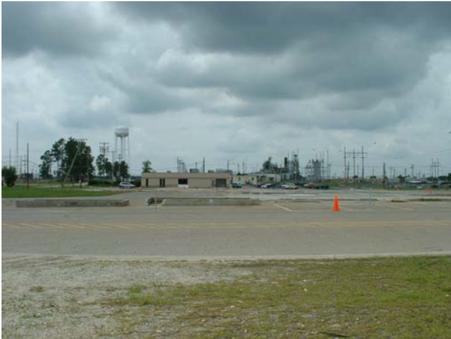
Figure 7. Building 716-A Slab, After Decommissioning
