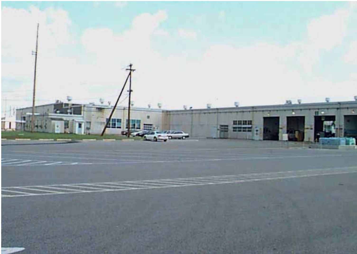
Figure 6. Building 716-A, Before Decommissioning
