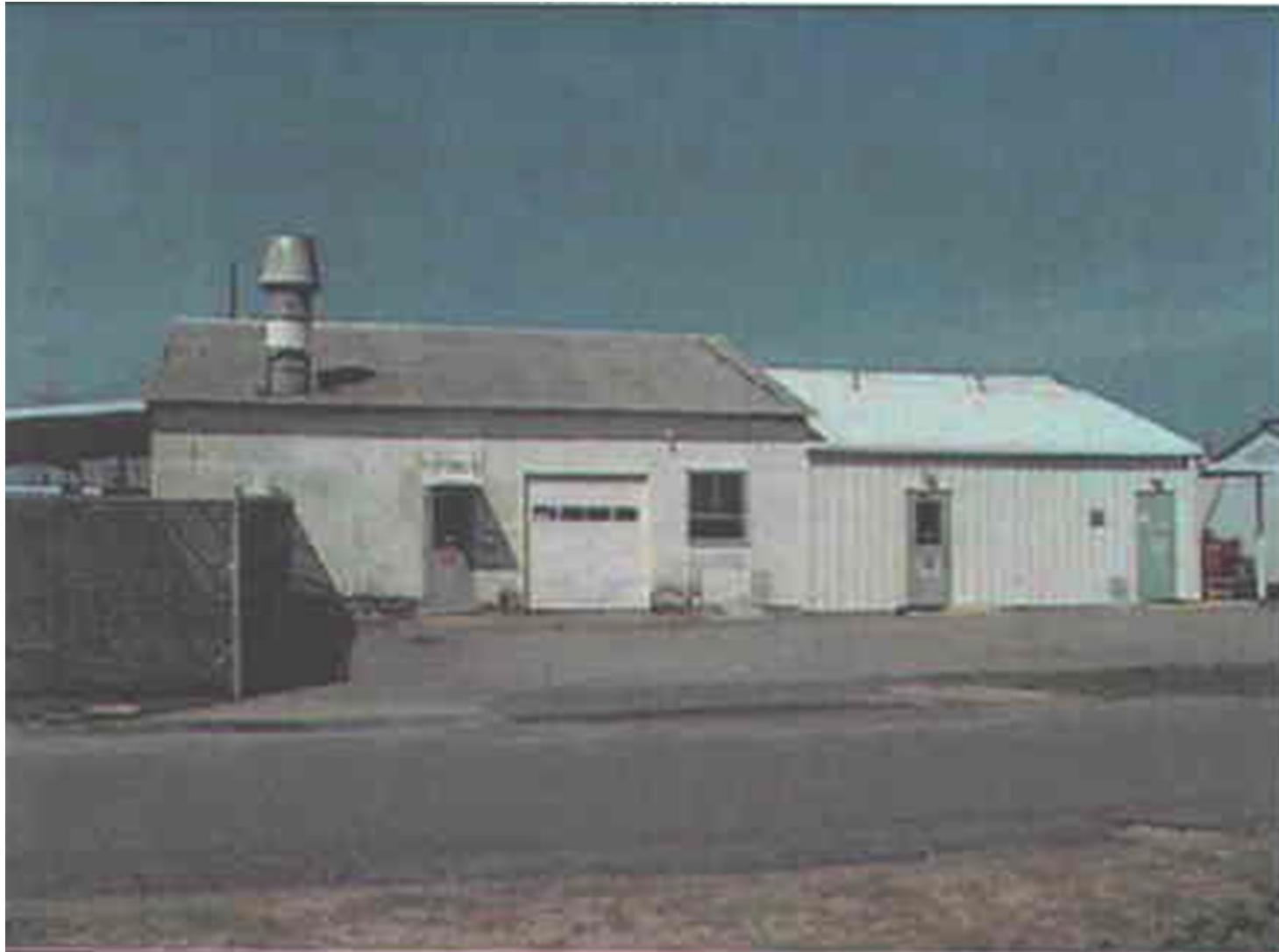
Figure 11. Building 725-A, Before Decommissioning
