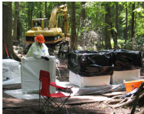
Photos of excavation in the lower subunit of LTR as a representation of Alternative 5 Excavation and Disposal of PTSM Sediment/Soil in EA1 and EA5
