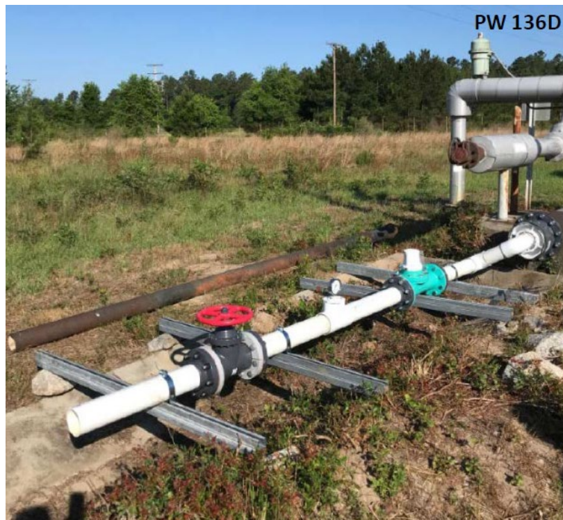
Figure 6. Production Well Flow Testing Setup
