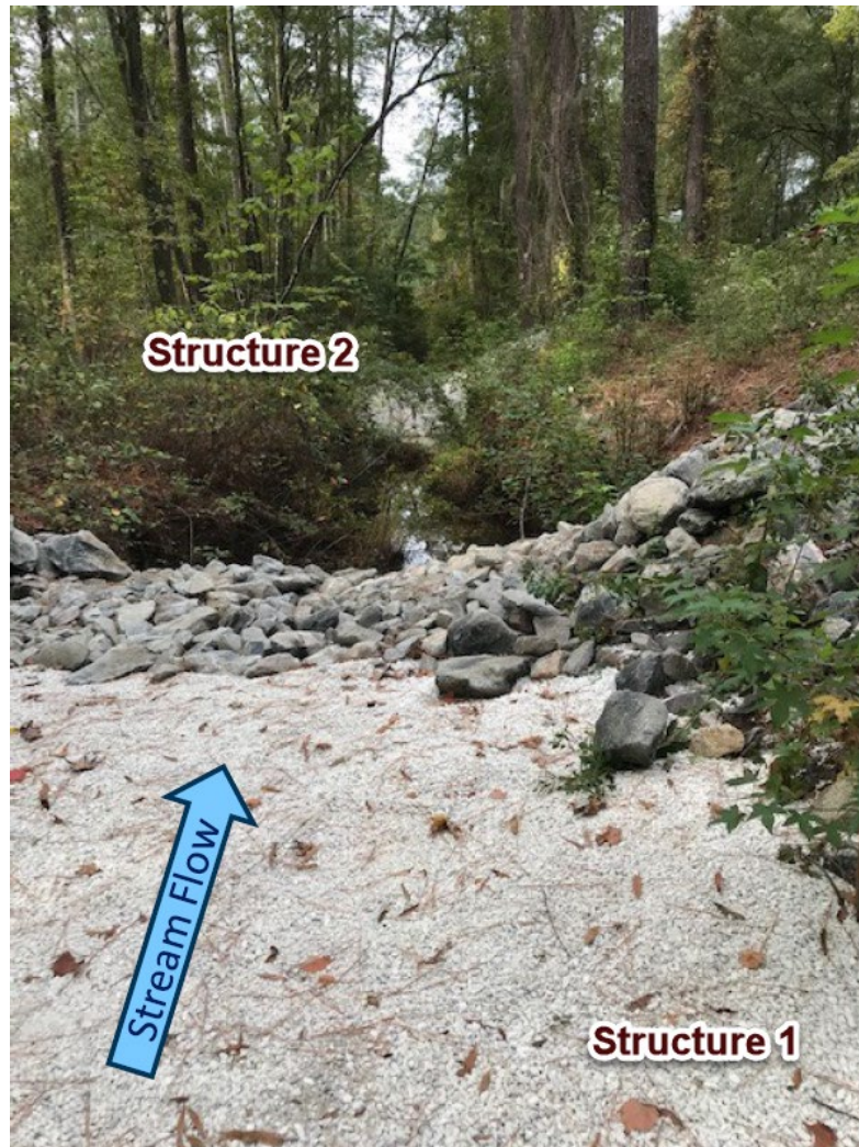
Figure 13. D-Area Effluent Discharge Canal \text{CaCO}_3 Reactive Structures
