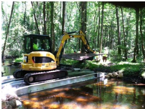
Photos of excavation in the lower subunit of LTR as a representation of Alternative 5 Excavation and Disposal of PTSM Sediment/Soil in EA1 and EA5
