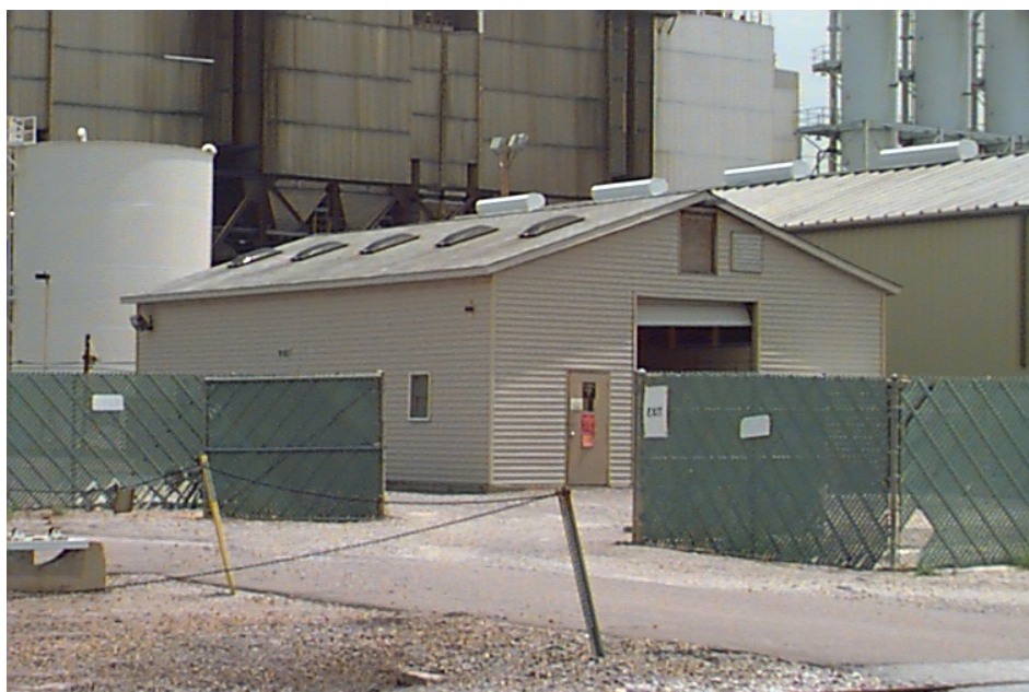
Figure 1. Building 710-16D, Storage Building
