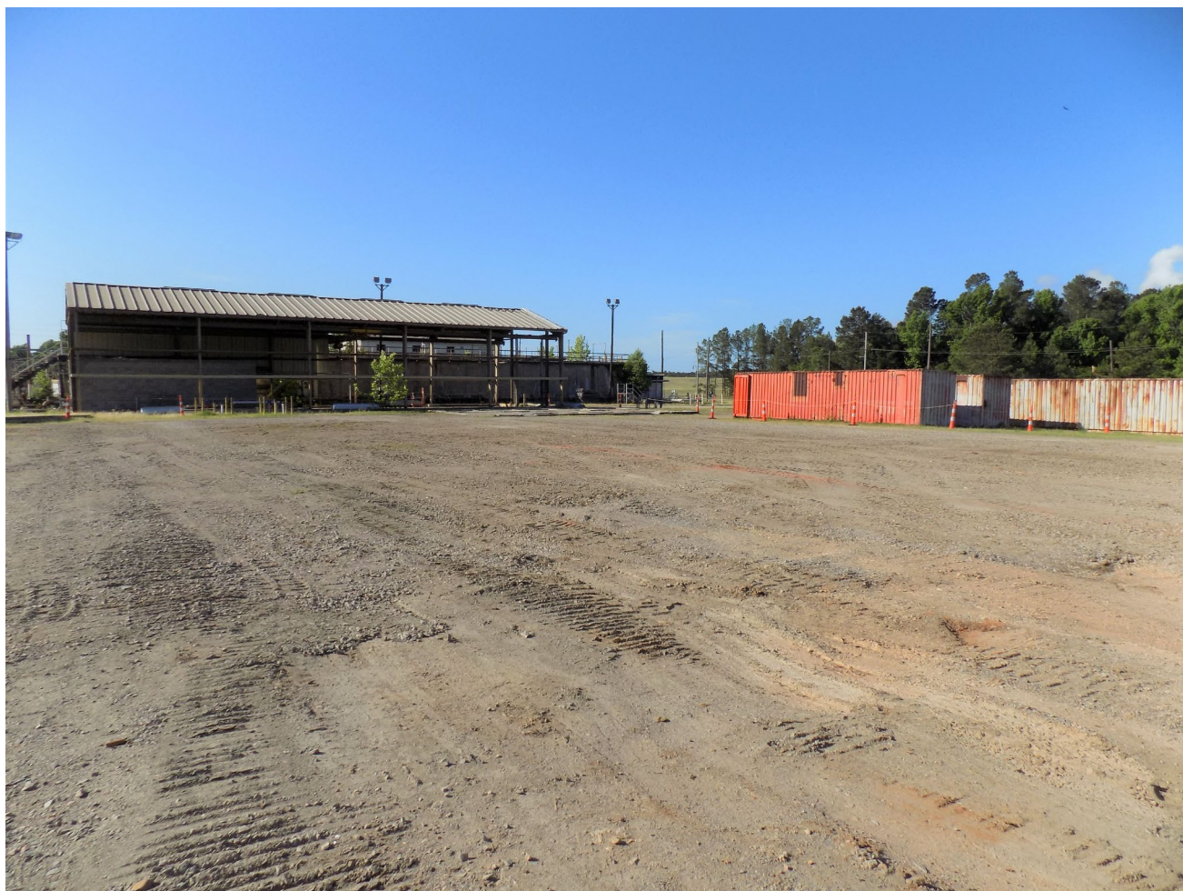
Figure A-2. Building 704-7D (Looking Southwest) After Decommissioning
