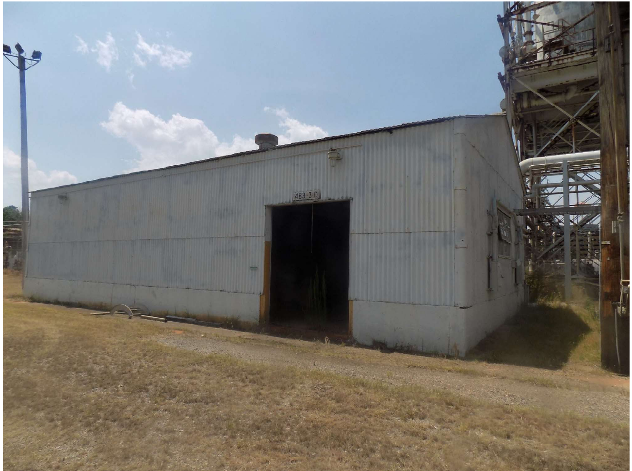
Figure 1: Building 483-3D (Looking Northwest) Before Decommissioning
