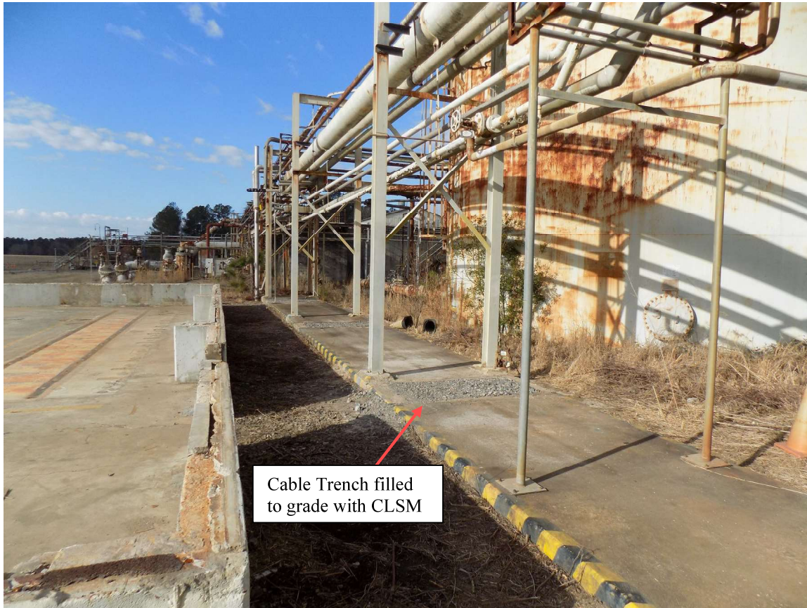
Figure 3: Exterior North Cable Trench (Looking Northwest) After Decommissioning
