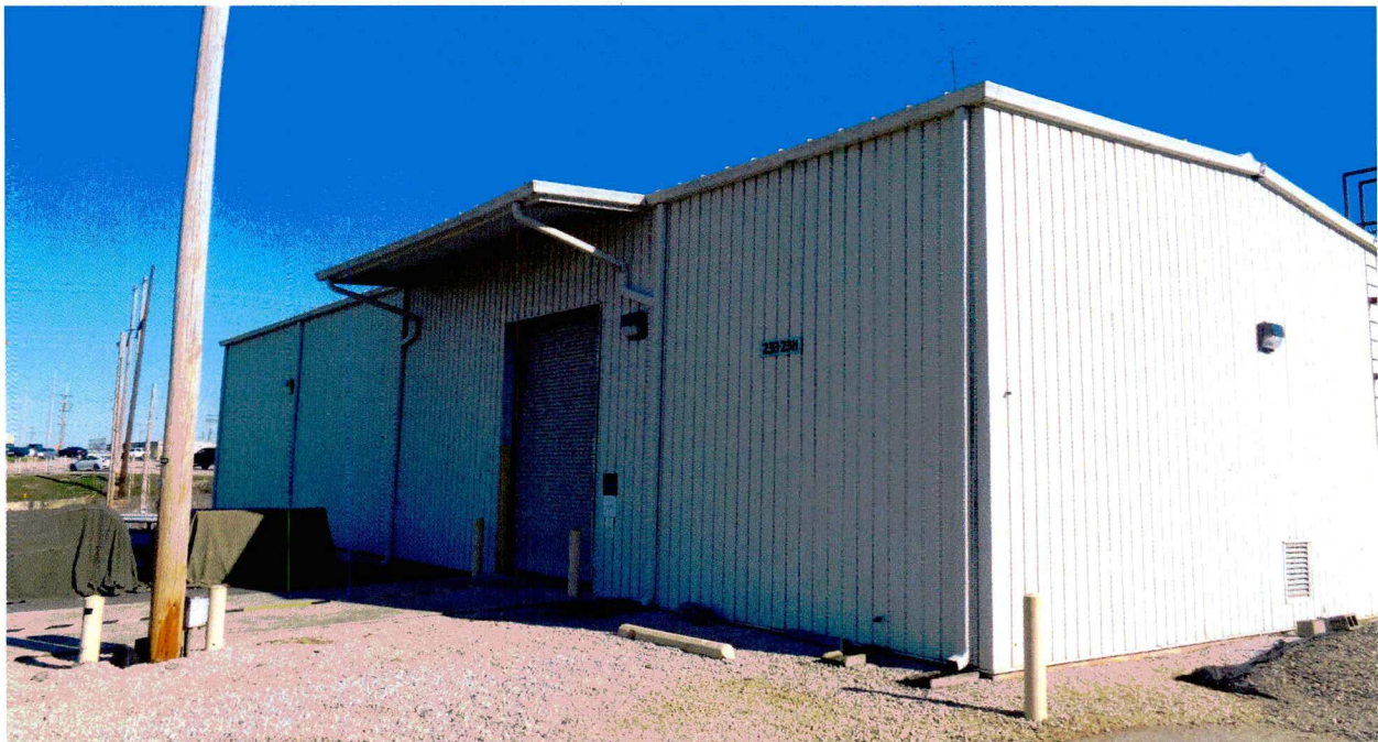
Figure 2. Building 233-23H Looking Southeast
