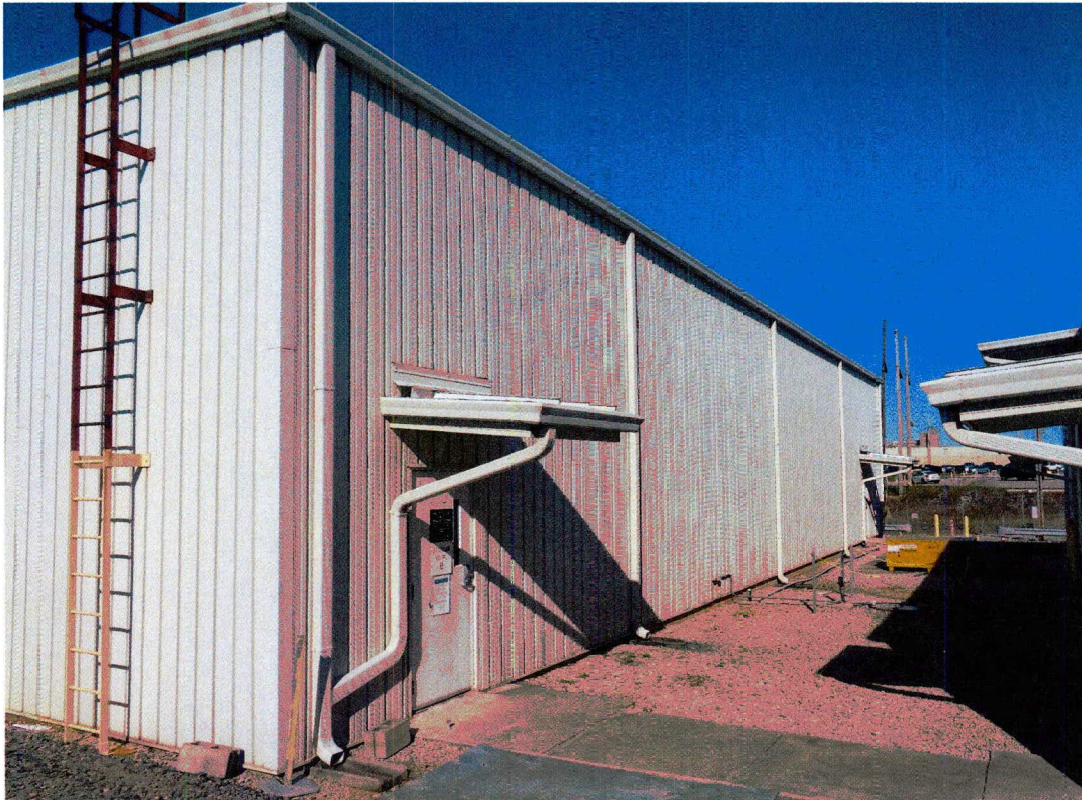
Figure 3: Building 233-23H Looking Northeast
