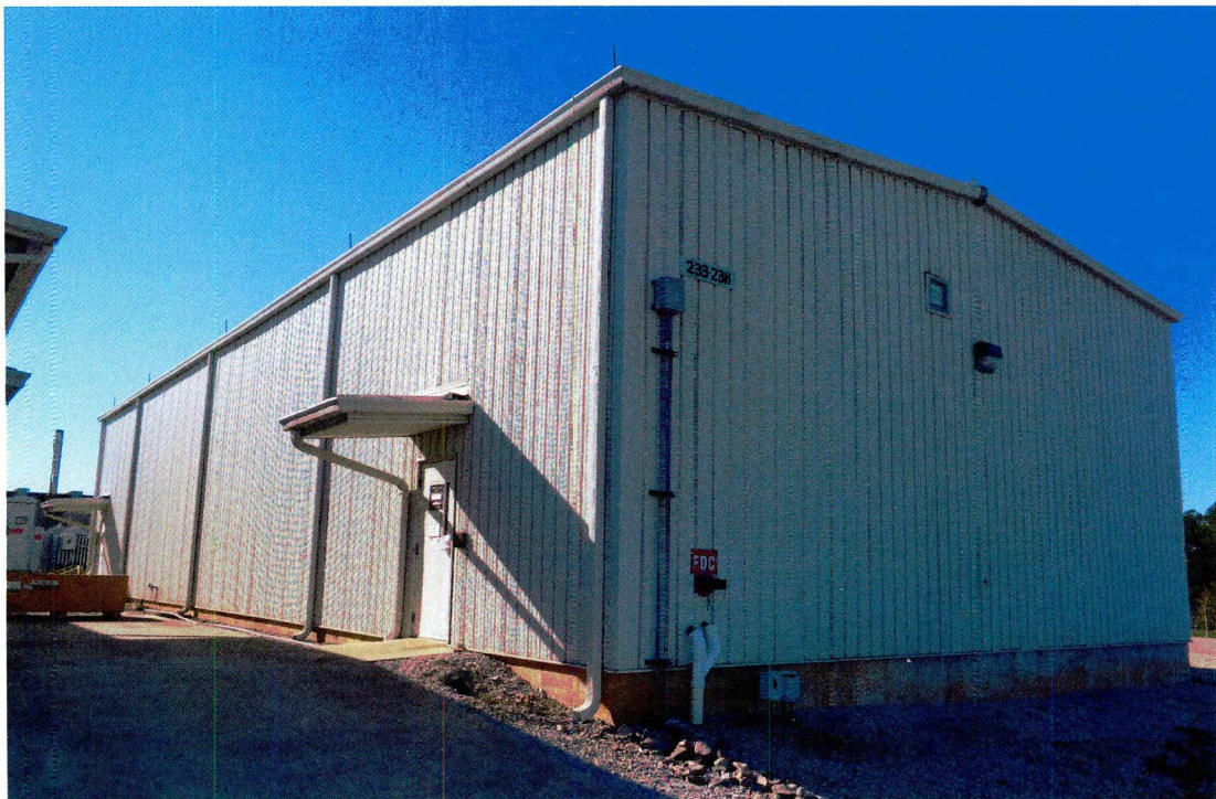
Figure 4. Building 233-23H Looking Northwest
