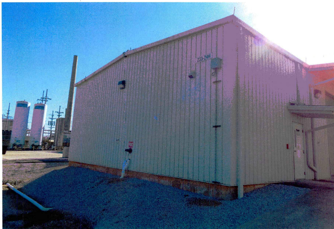
Figure 8: 233-24 H Looking Southwest
