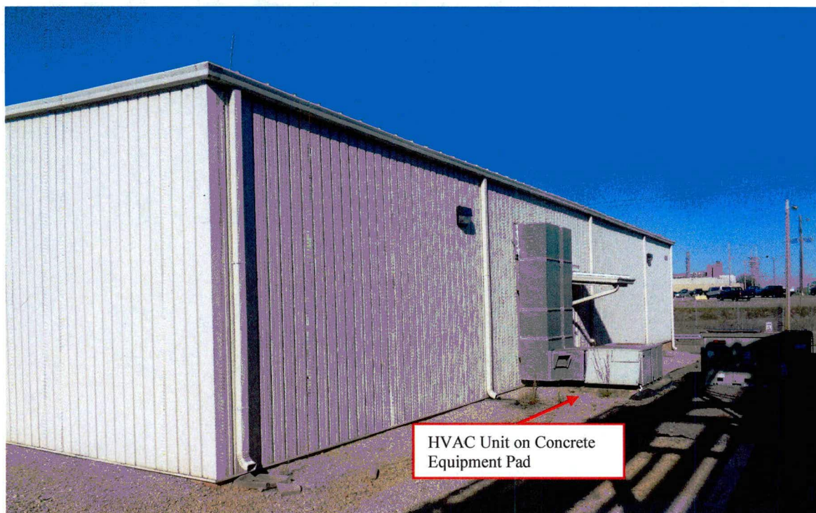
Figure 7: 233-24 H Looking Northeast
