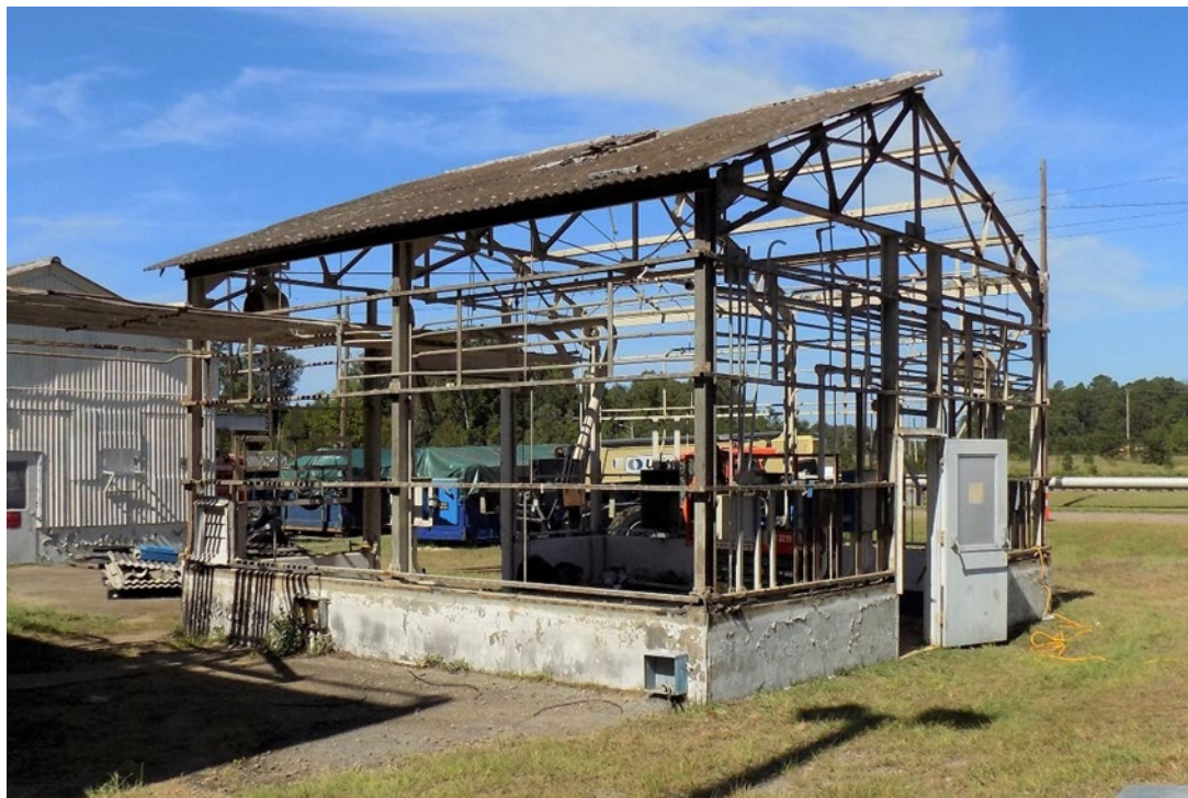
Figure A-2. Building 482-2D (Looking Northwest) After Asbestos Abatement
