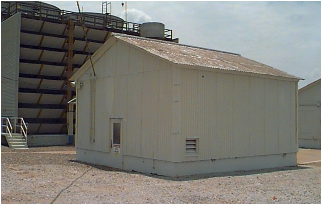
Figure A-1. Building 482-2D (Looking Southwest) Before Asbestos Abatement
