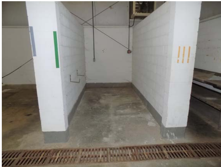
Figure 8. Building 483-7D Chemical Storage Area (Typical)
