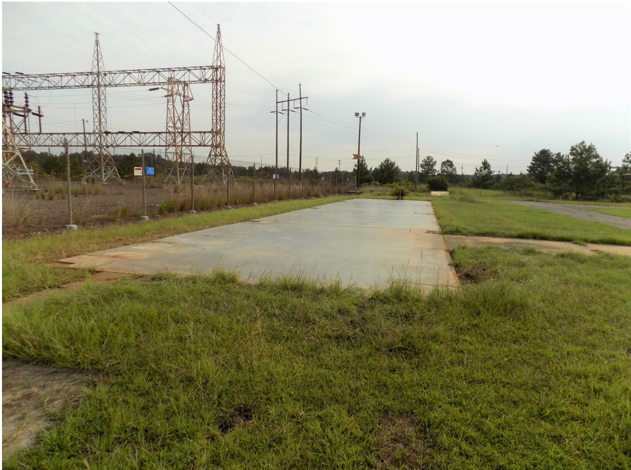
Figure 2: 484-15D (Looking East) After
