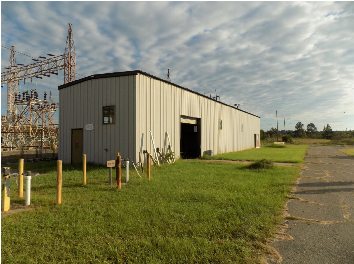
Figure 1: Building 484-15D (Looking East) Before
