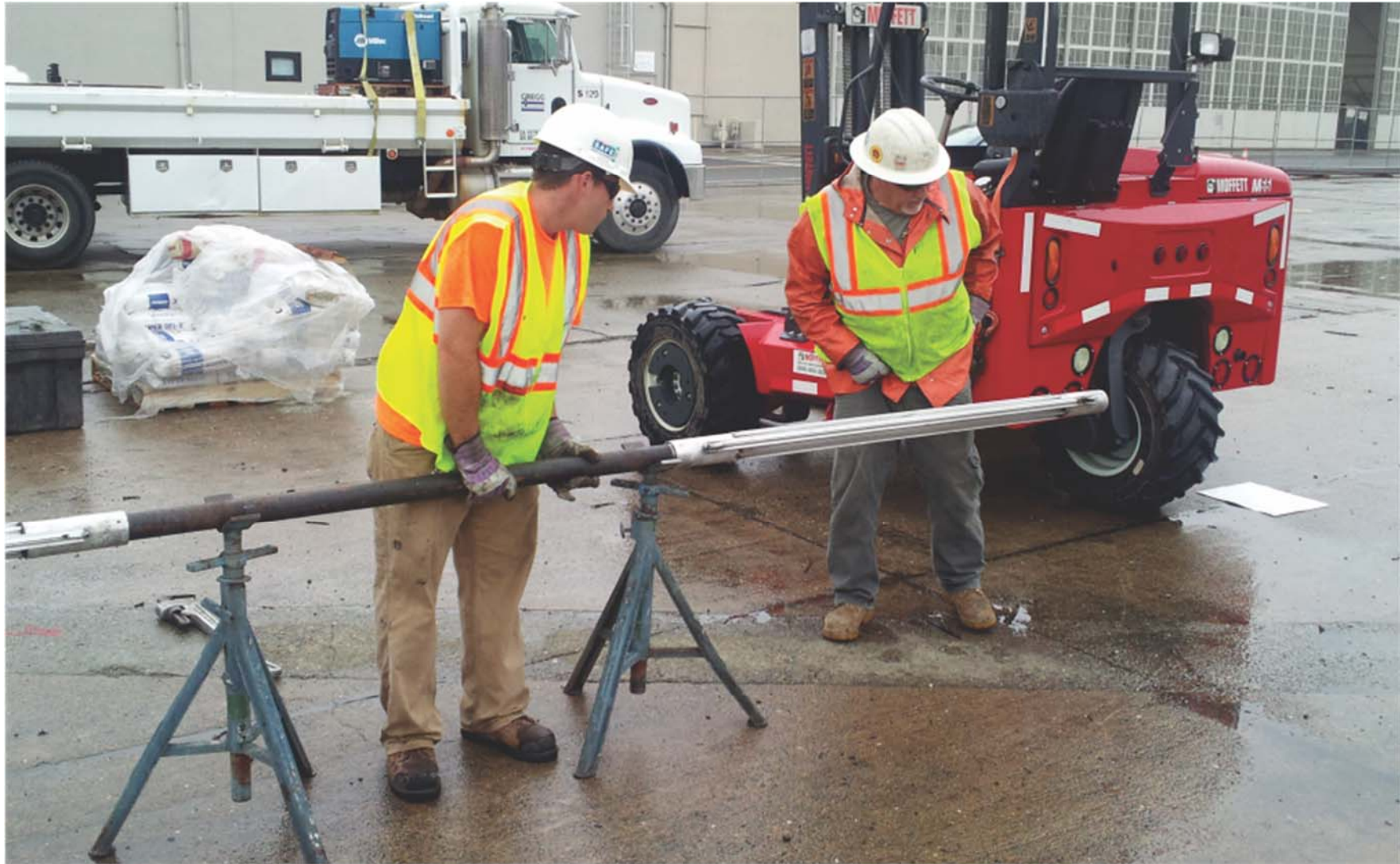
Figure 13. Preparing Expansion Casing System for Installation
