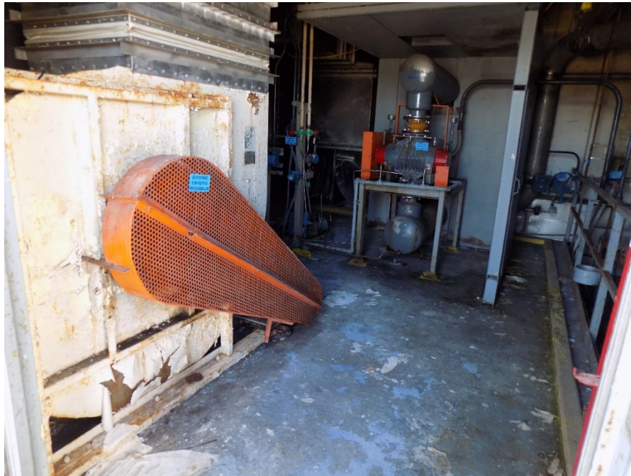
Photo 10: The above photo shows the general condition of the concrete and peeling paint on the third floor of A-Line in Room 302, Zone 5.3.2.
