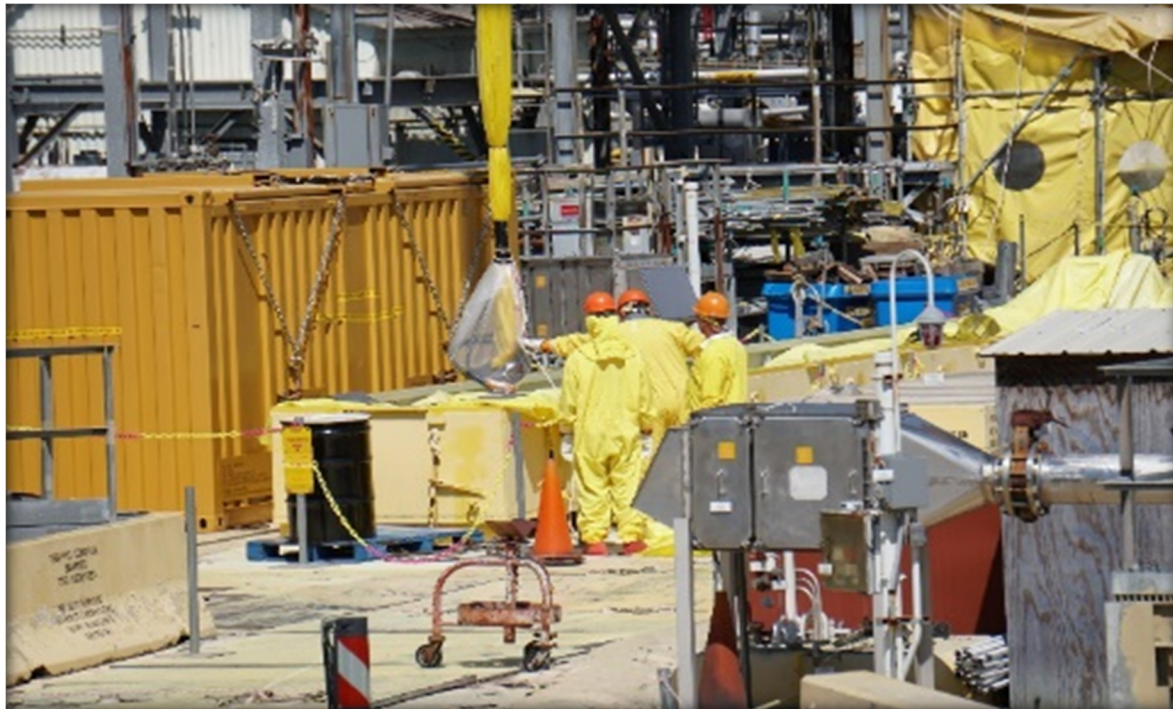
Figure 4: Riser Mining at Tank 3F Riser 5 to Support Transfer Pump Installation
