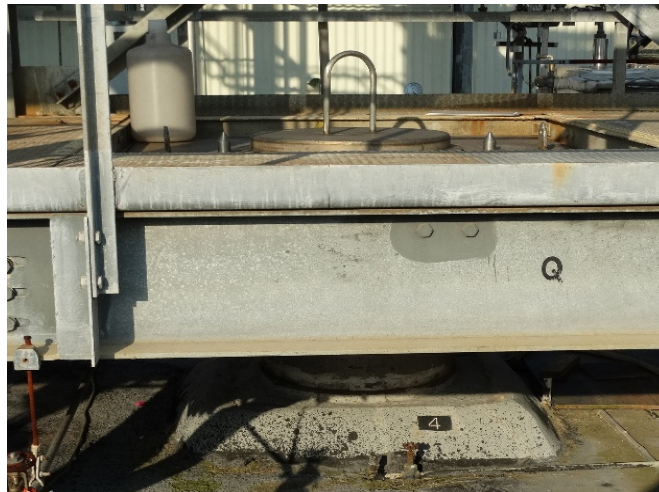
Figure 5: Tank 9H Riser 4 D&R Before (With Spray Chamber)
