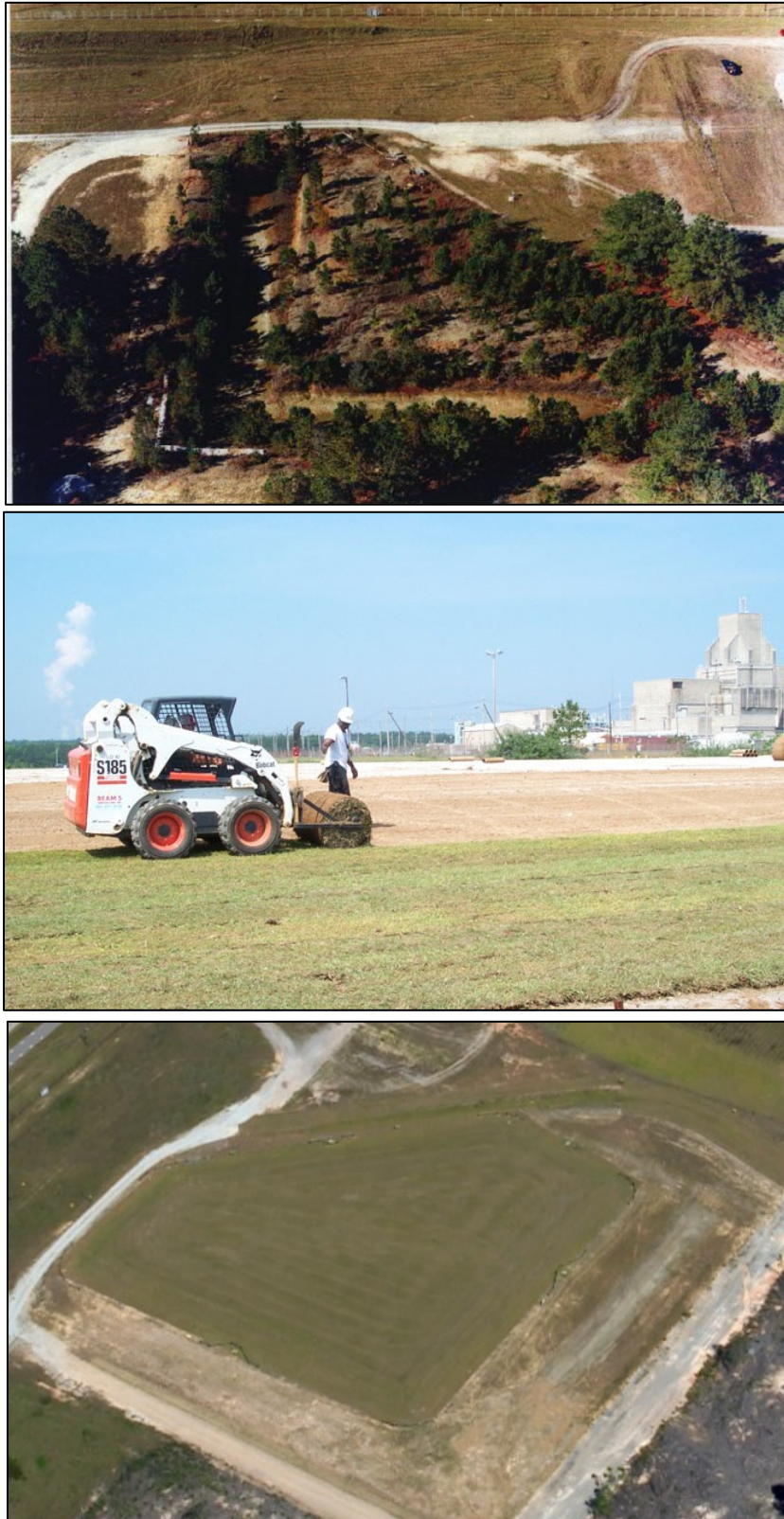
Figure M-4. Before, During, and After Remedial Action at LRSB OU
