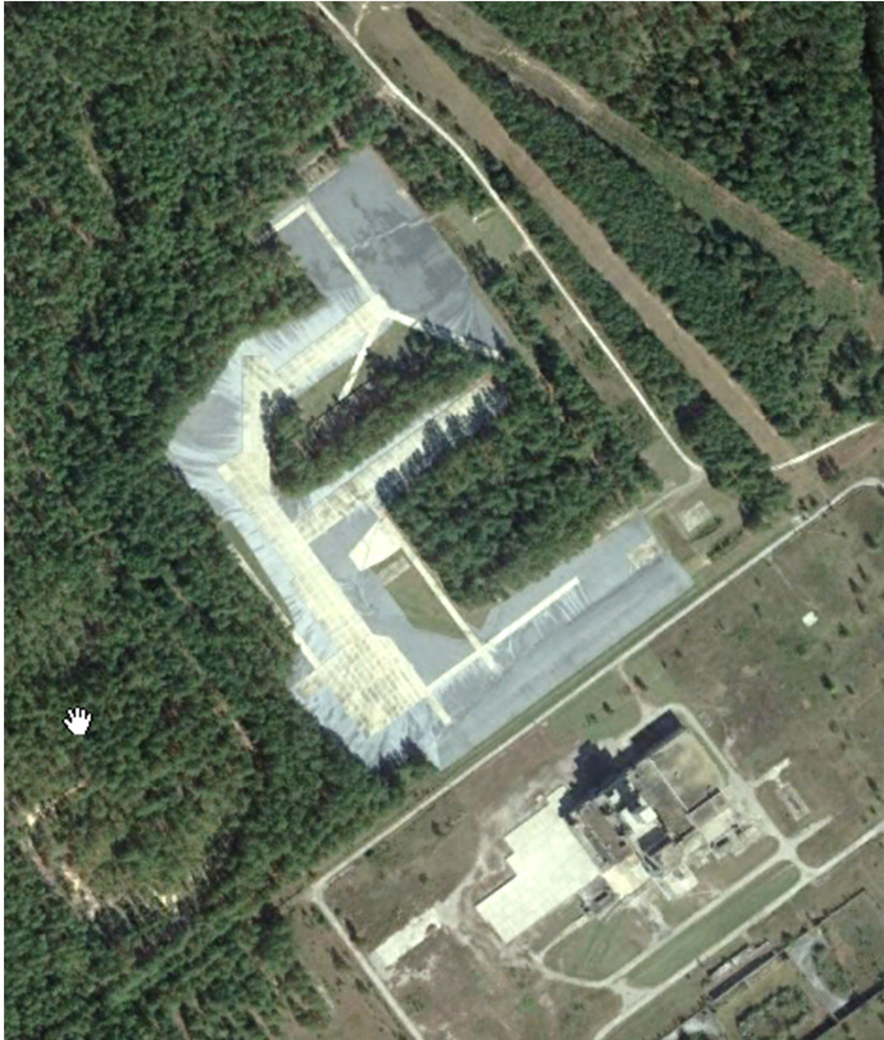
Figure H-4. Current Aerial Photo of the R-Reactor Seepage Basins OU (2017)
