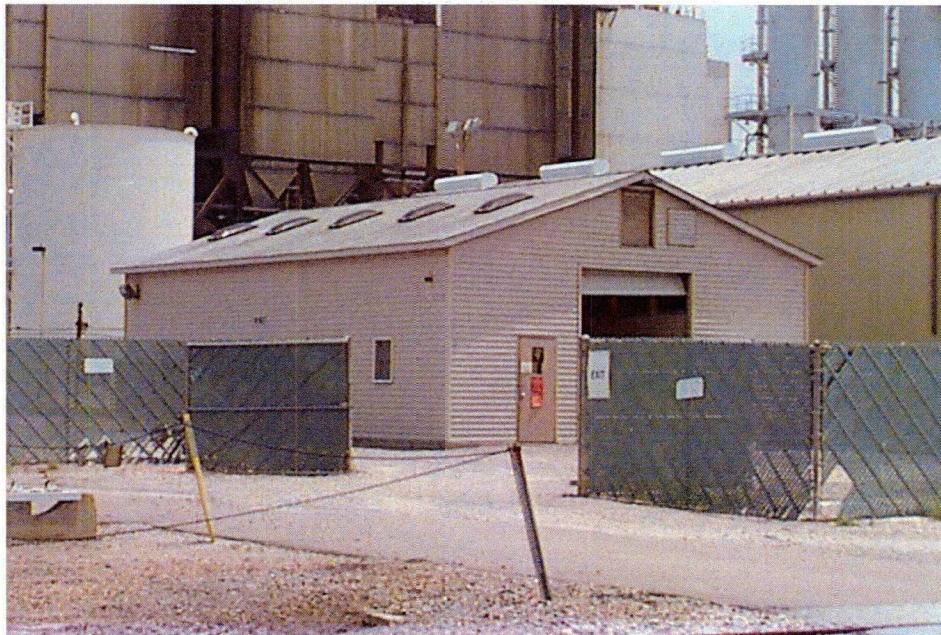
Figure 1. Building 710-16D, Storage Building
