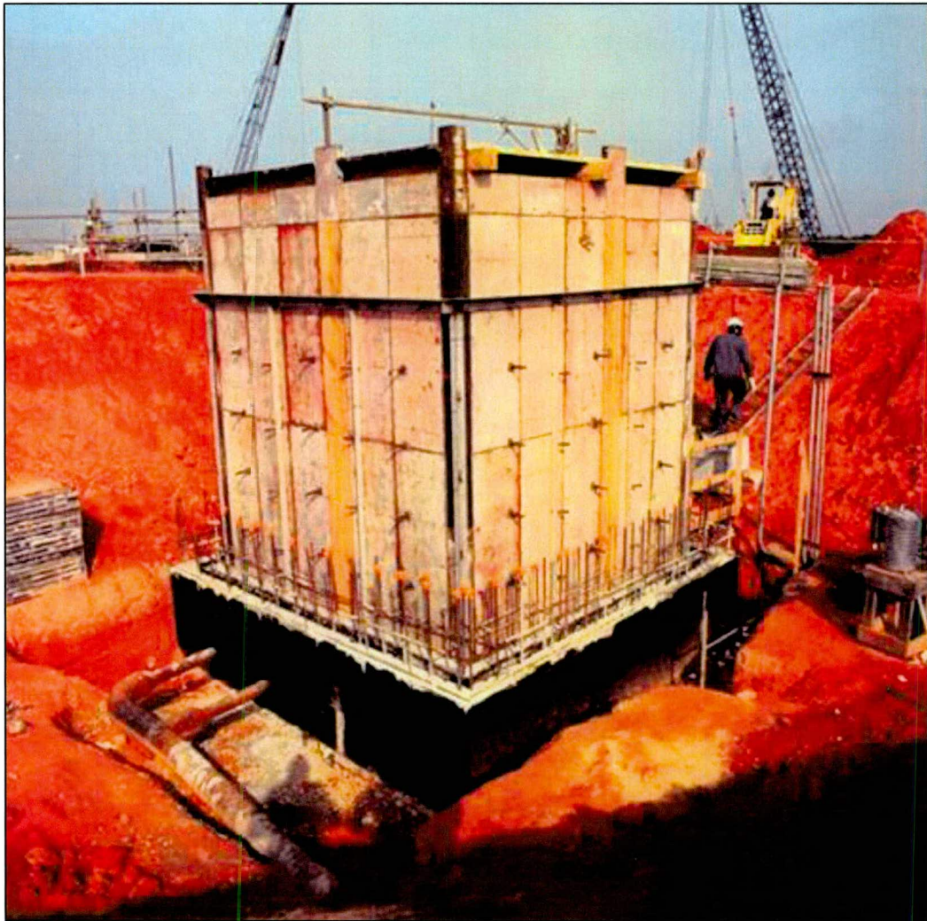
Figure 6: FDB-5 Early Construction Phase
