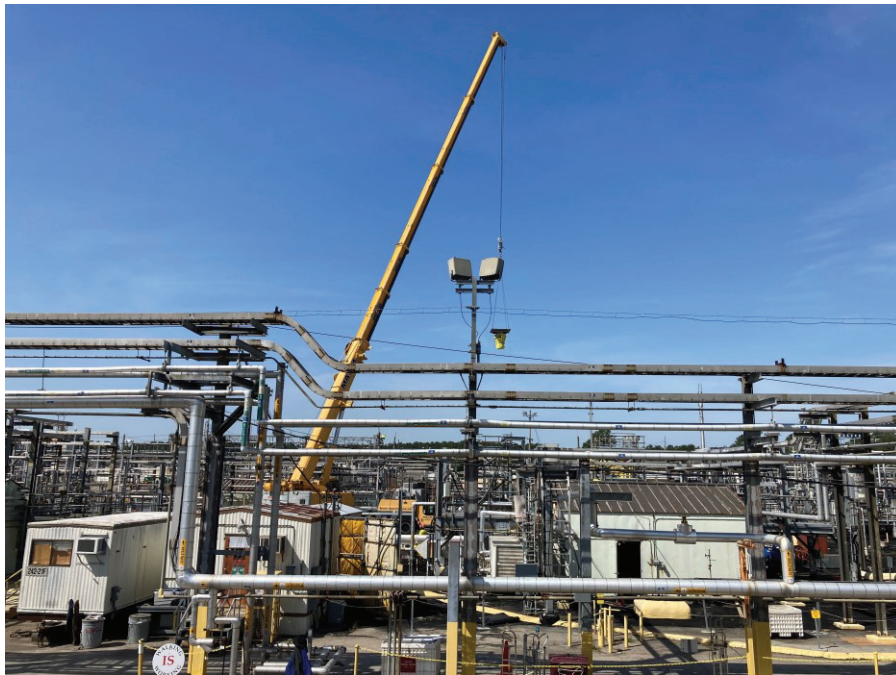
Figure 5: Tank 3F Riser Spray Chamber Disassembly & Removal
