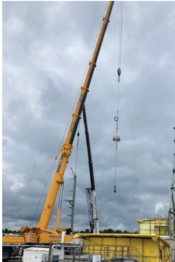
Figure 9: Installation of Tank 35H Riser C1 Submersible Transfer Pump (STP)
