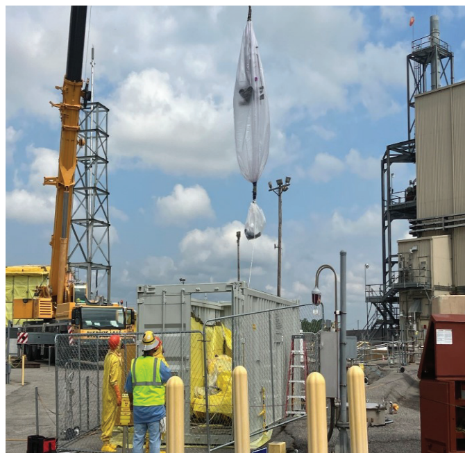
Figure 7: Tank 31H Draw Off Valve Removal
