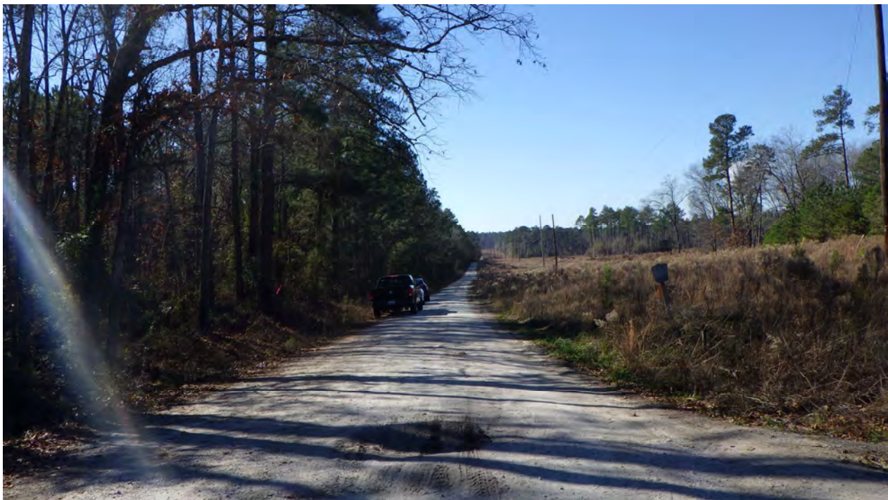
N: Westerly Overview of the Access & Utility Easement
