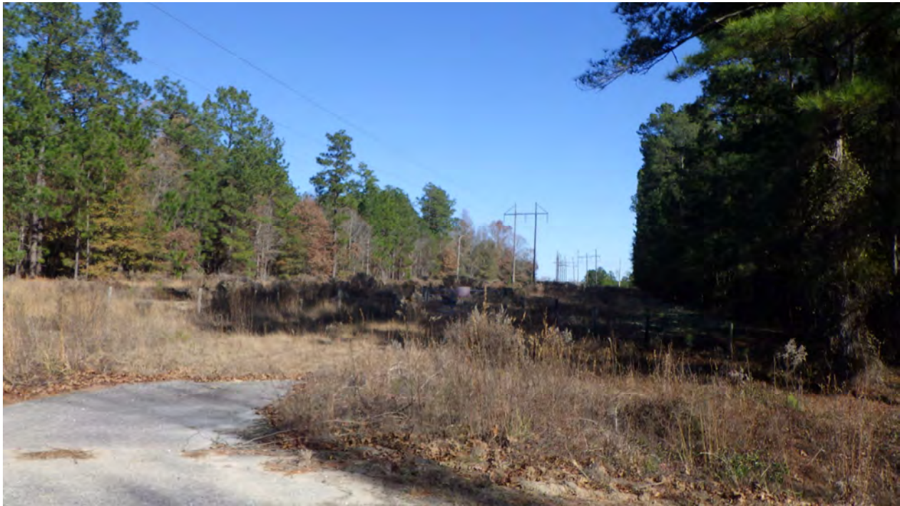
R: View Looking East Toward the Power Substation at the SRS, as Seen From SC Highway 125
