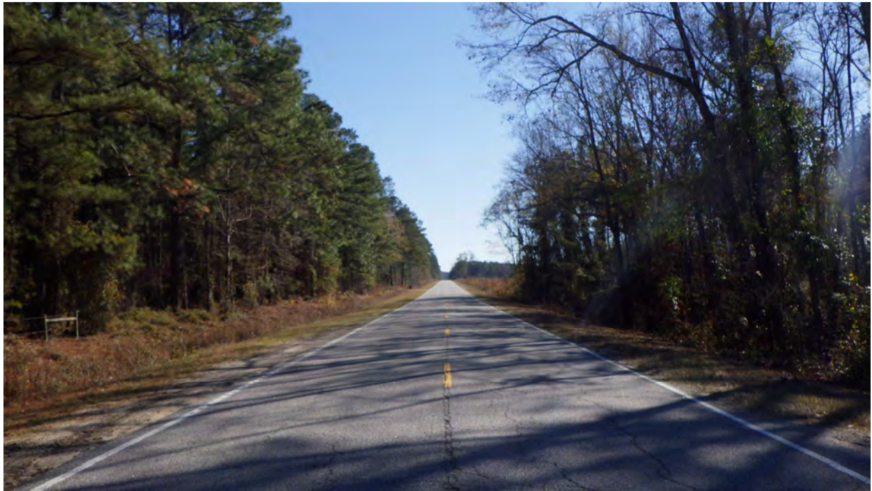
S: View Looking South-Southeast Along SC Highway 125
