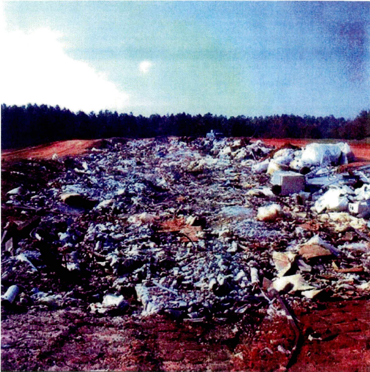
Figure C-3. Photo of CSBRP OU Before Remediation Activities (April 1985)
