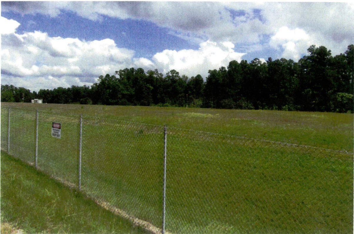
Figure E-3. Current On-Unit Photographs of the Cover System of the FHWMF OU (2016)
