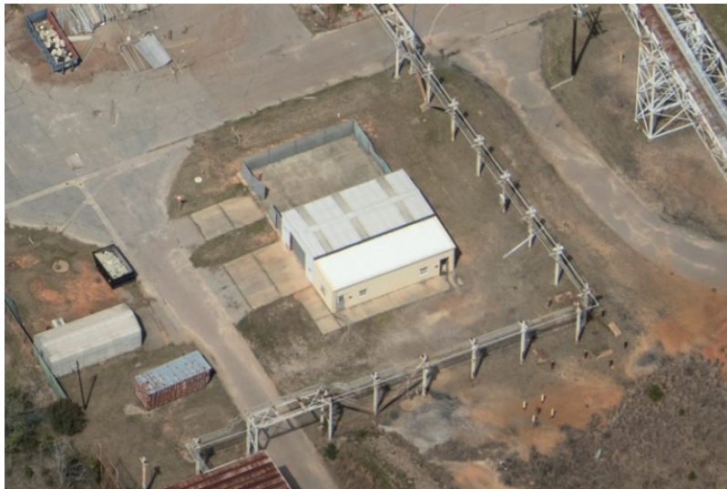
Figure 6. Aerial View of 484-12D Laydown Yard
