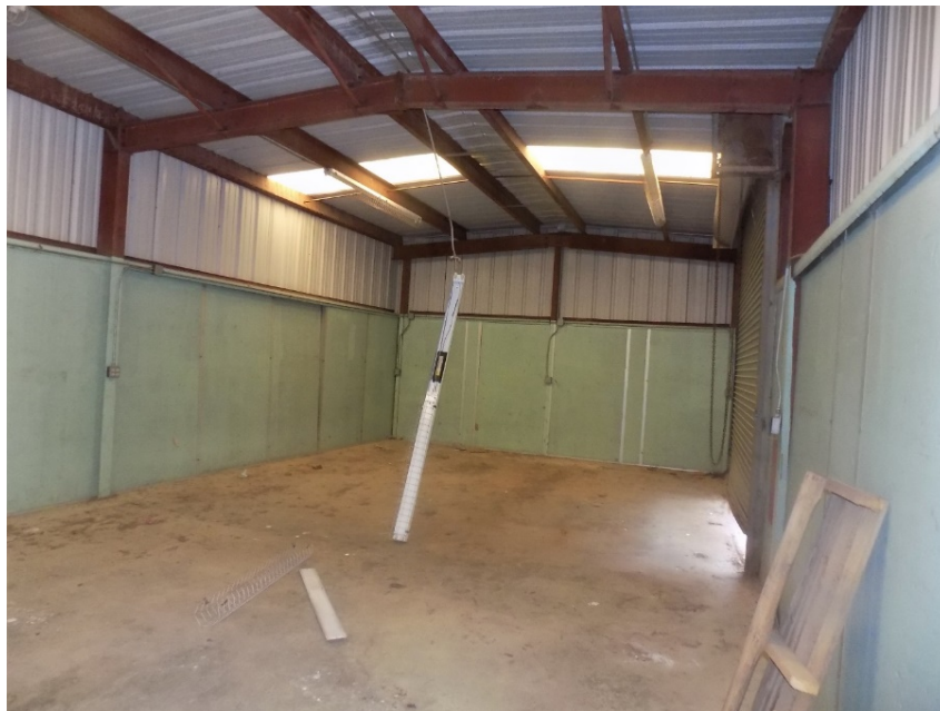
Figure 8. Interior View of Building 484-7D
