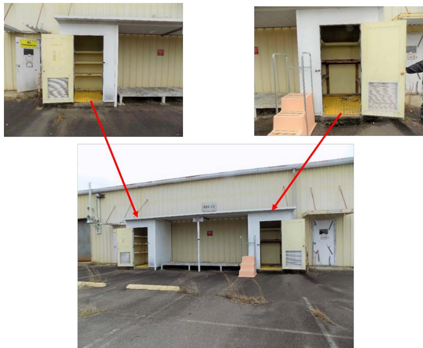
Figure 2. Interior and Exterior Views of 484-4D Storage Buildings
