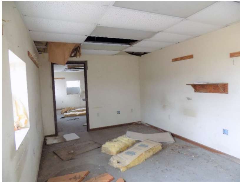
Figure 4. Office Area of 484-12D
