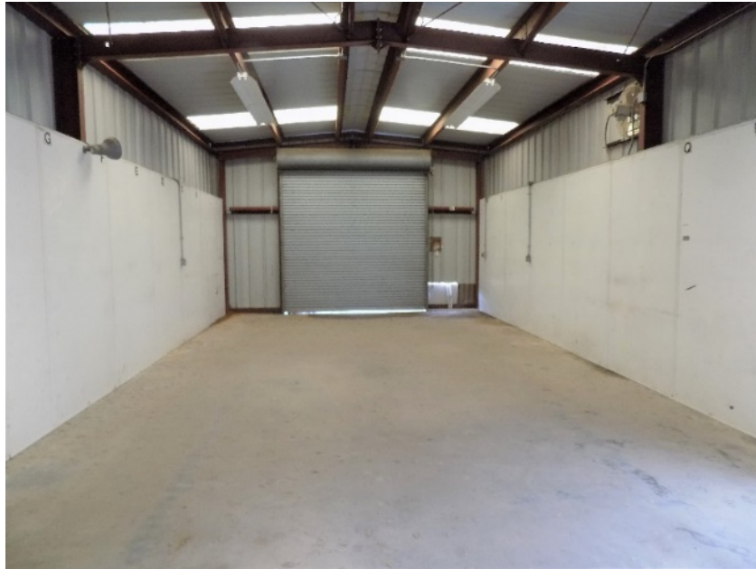
Figure 5. Garage Area of 484-12D
