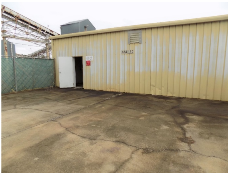
Figure 7. Ground View of 484-12D Laydown Yard
