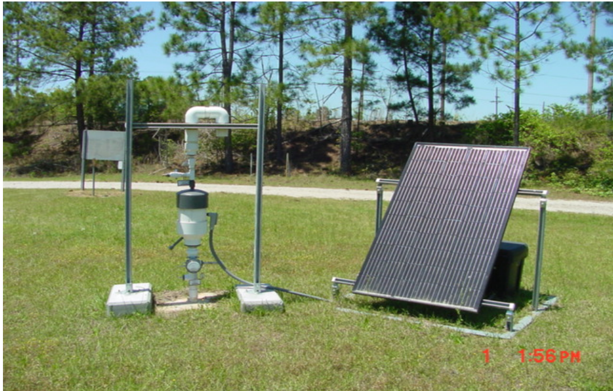
Figure 4. Typical Passive SVE Well
