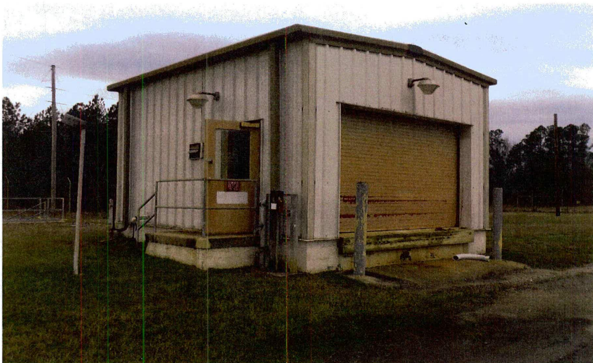
Figure 4. Building 607-14D, Chemical Feed Building
