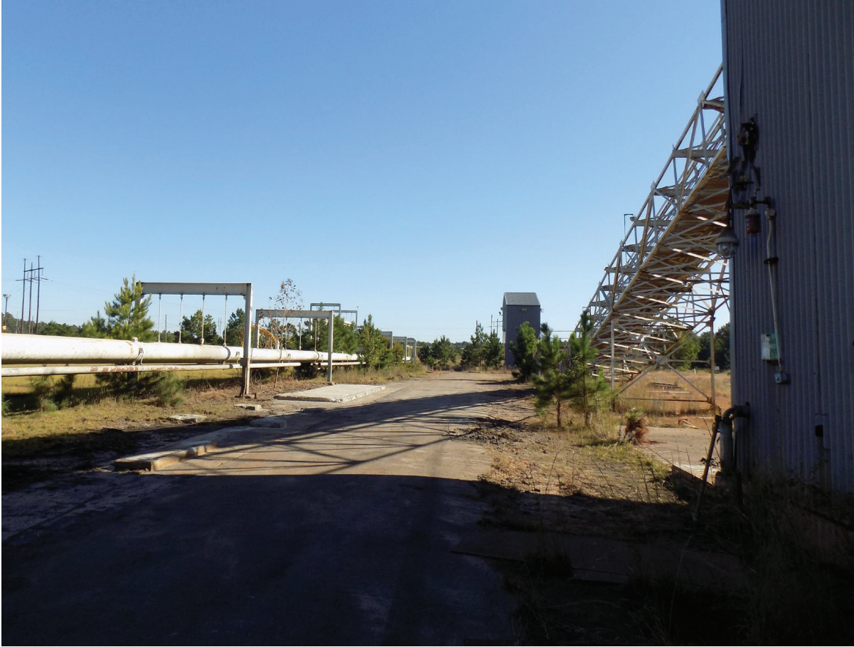
Figure 2: Building 484-9D (Looking East) After Decommissioning
