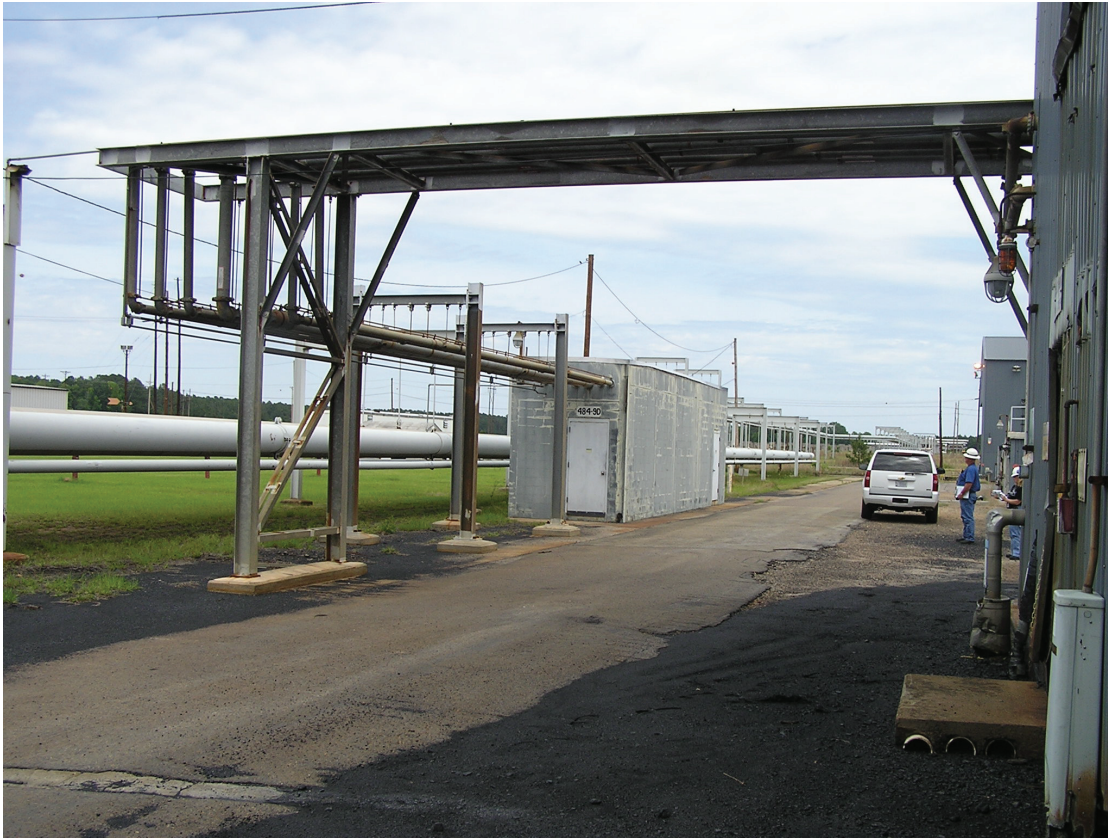
Figure 1: Building 484-9D (Looking East) Before Decommissioning
