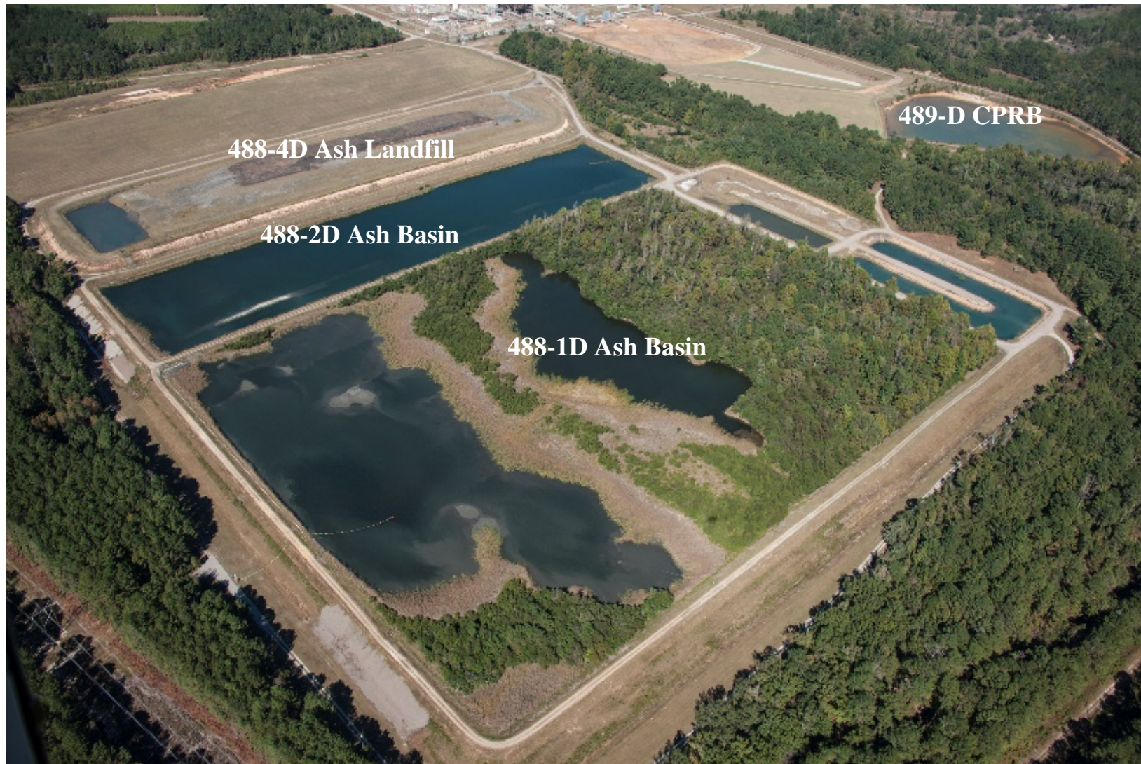
Figure 6. D-Area Project in October 2013 (Pre-Removal Actions)
