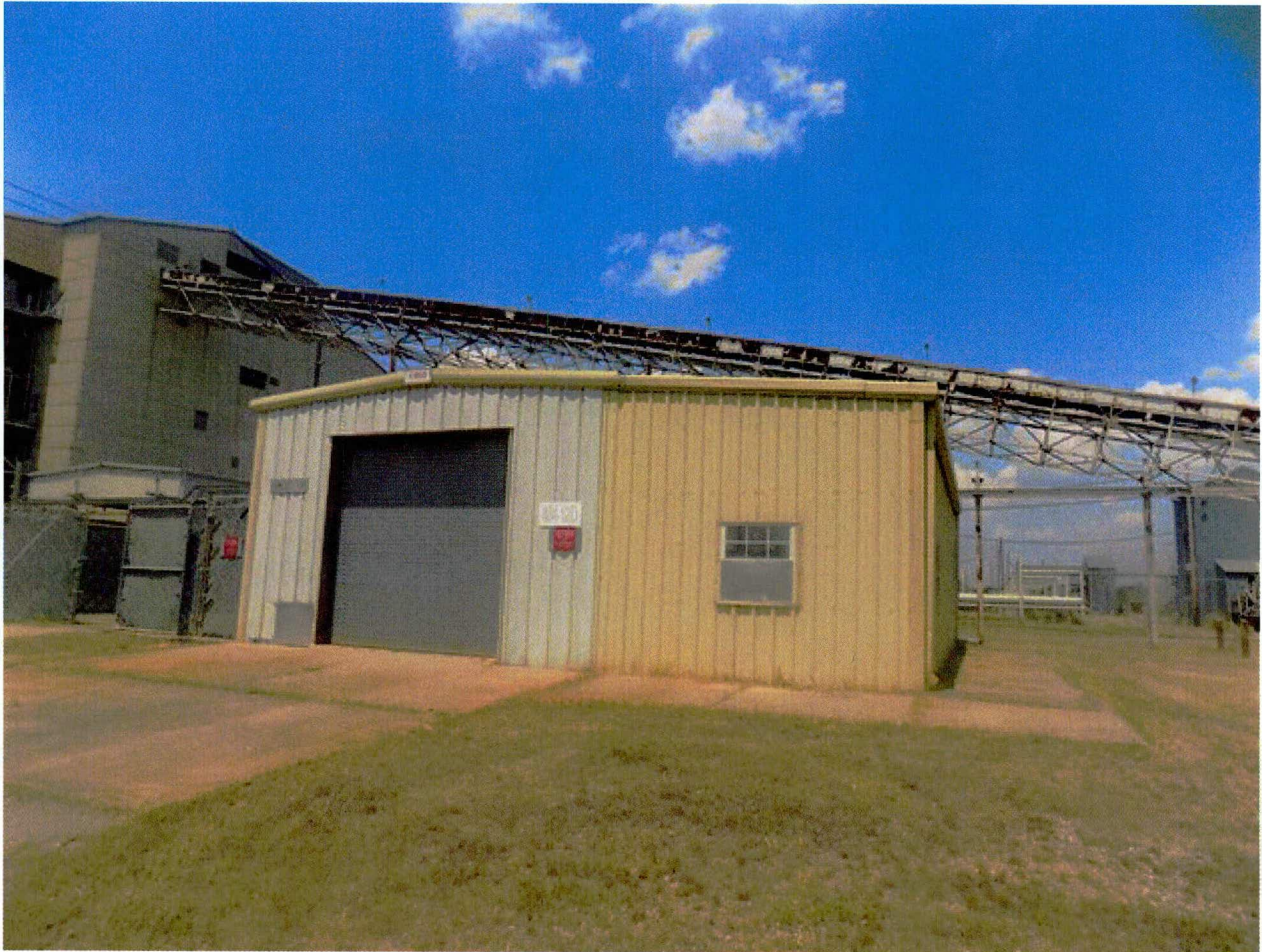
Figure A-1. Building 484-12D (Looking East) Before
