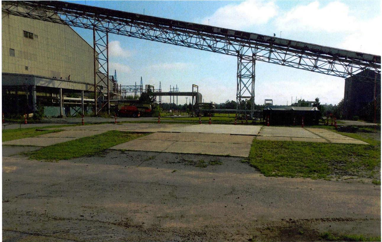
Figure A-2. Building 484-12D (Looking East) After
