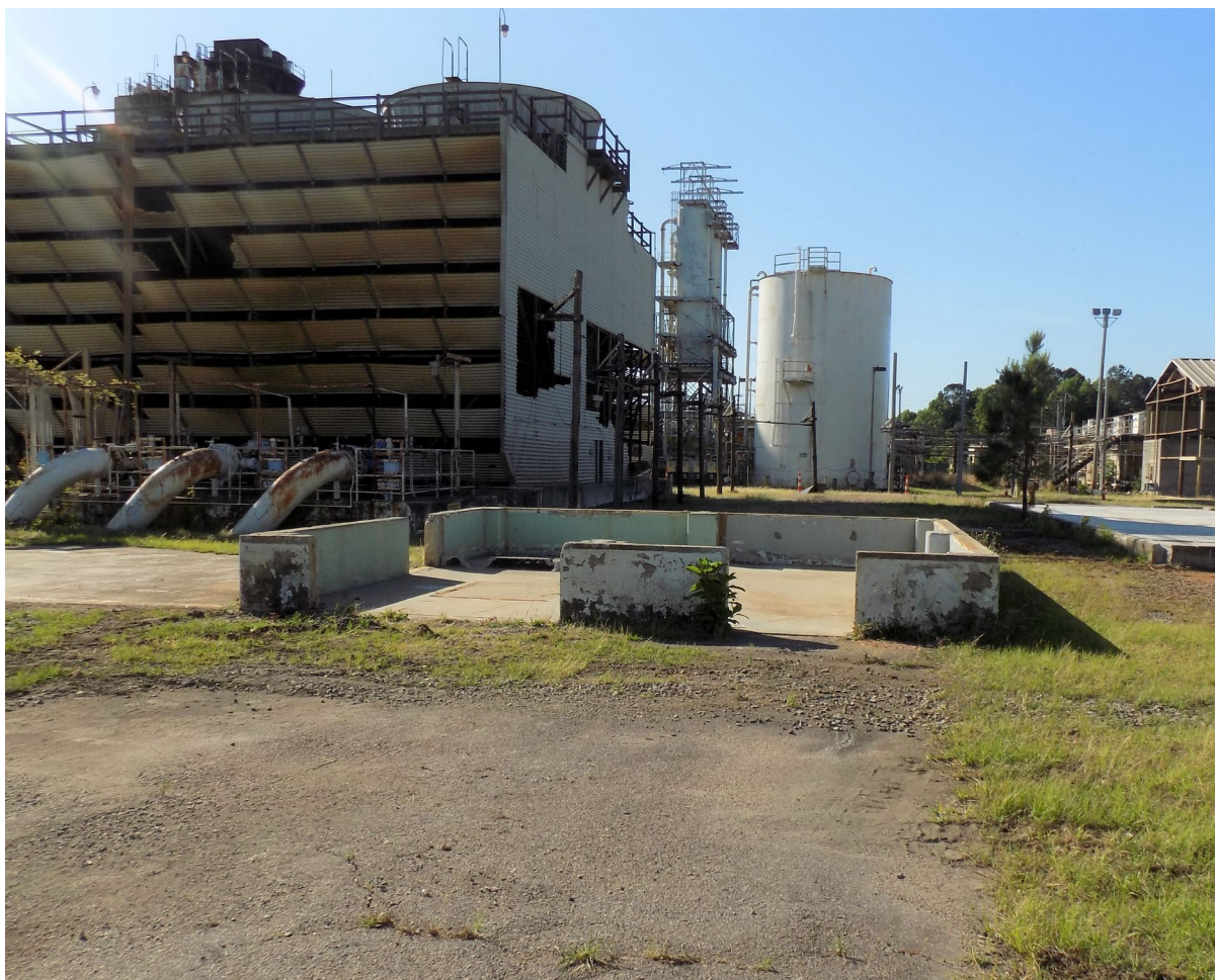
Figure A-3. Building 480-3D (Looking South) After Decommissioning
