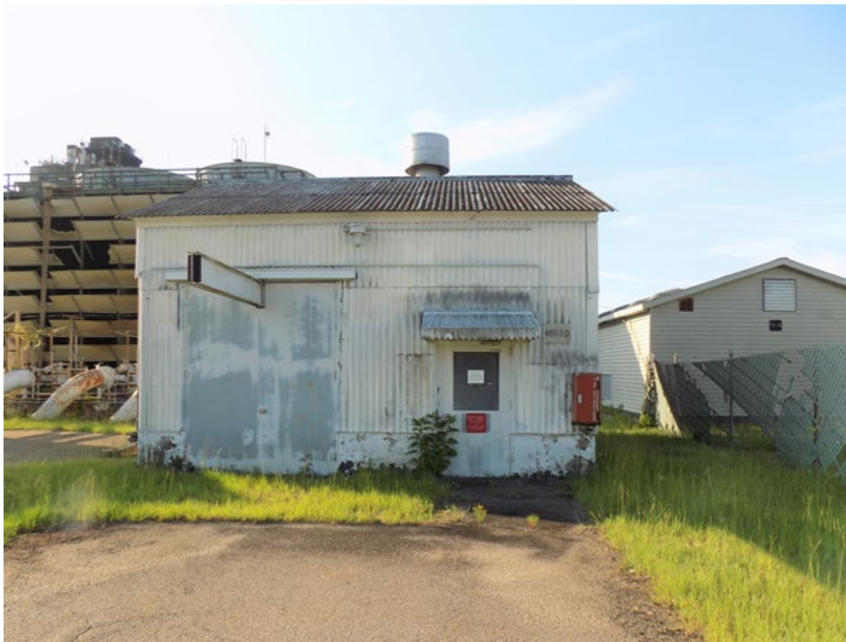
Figure A-1. Building 480-3D (Looking South) Before Asbestos Abatement
