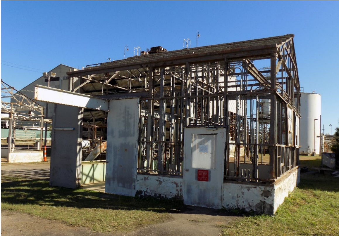
Figure A-2. Building 480-3D (Looking South) After Asbestos Abatement
