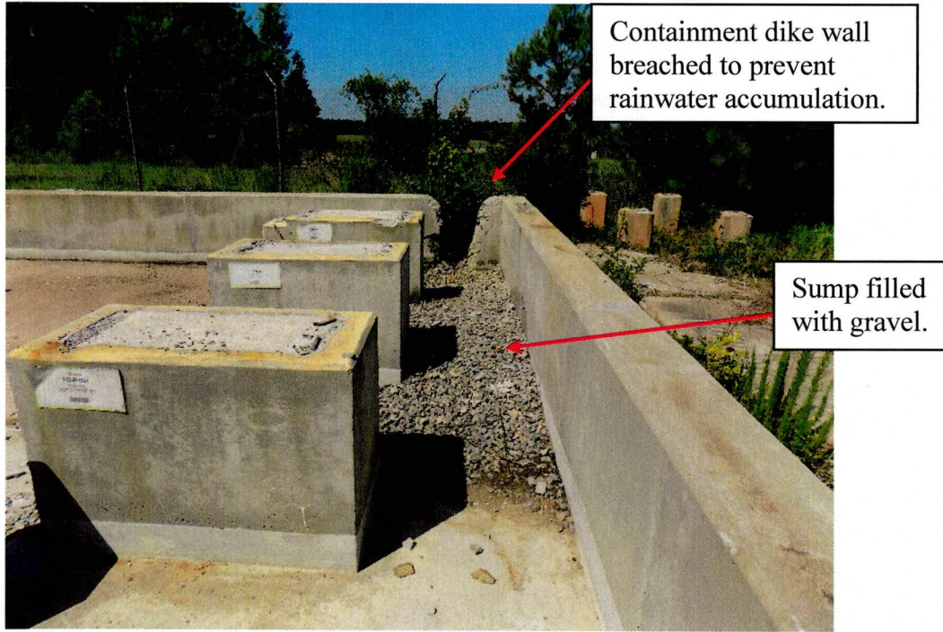
Figure 6. Building 454-D Slab and Sump (Looking West) After Final Decommissioning
