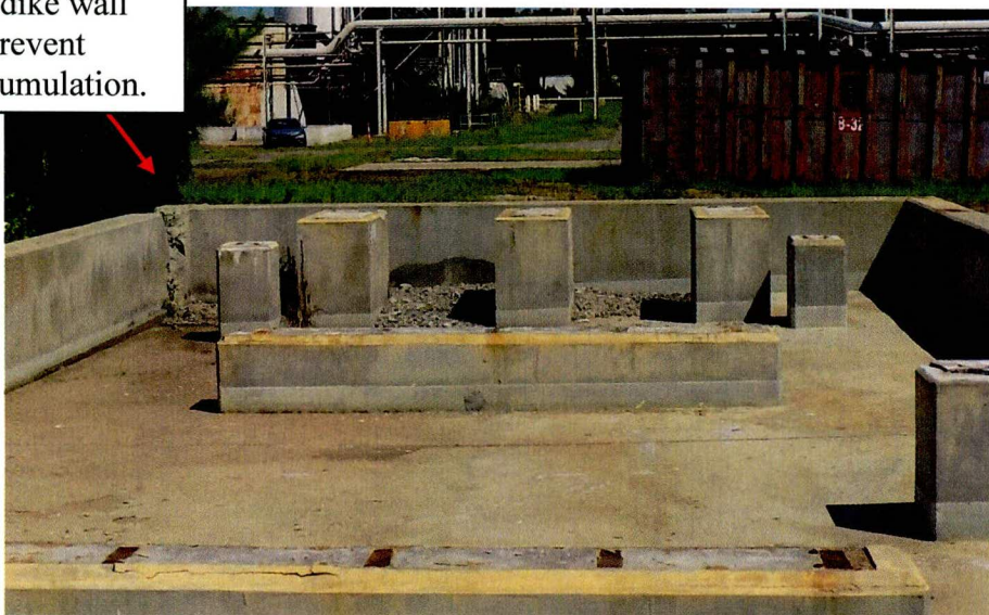
Figure 3. Building 454-D Slab (Looking North) After Final Decommissioning
