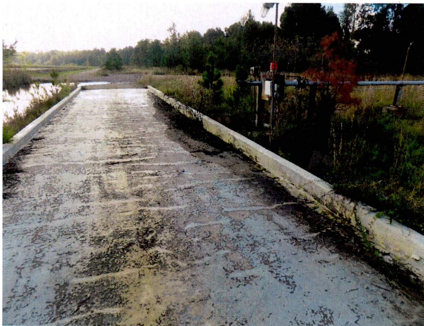
Figure 10. Building 454-1D (Looking South) Before
