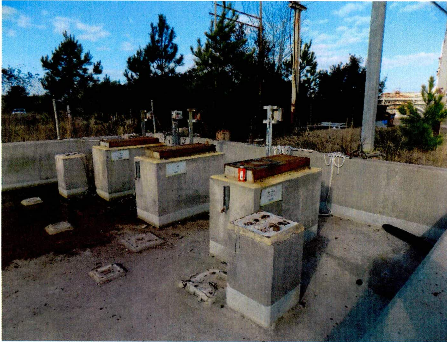
Figure 2. Building 454-D Slab (Looking Northwest) After Partial Decommissioning by CRO
