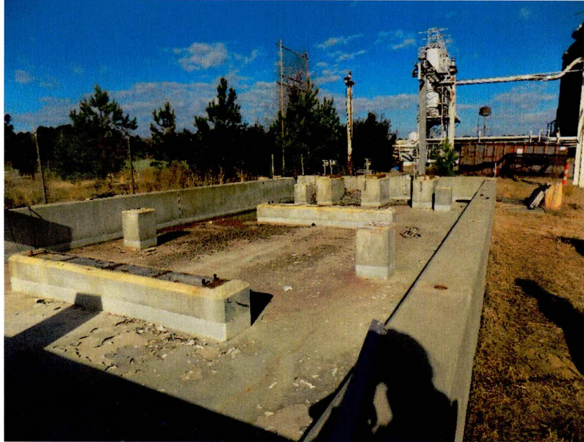
Figure 7. Building 454-D Slab (Looking Northwest) After Partial Decommissioning by CRO
