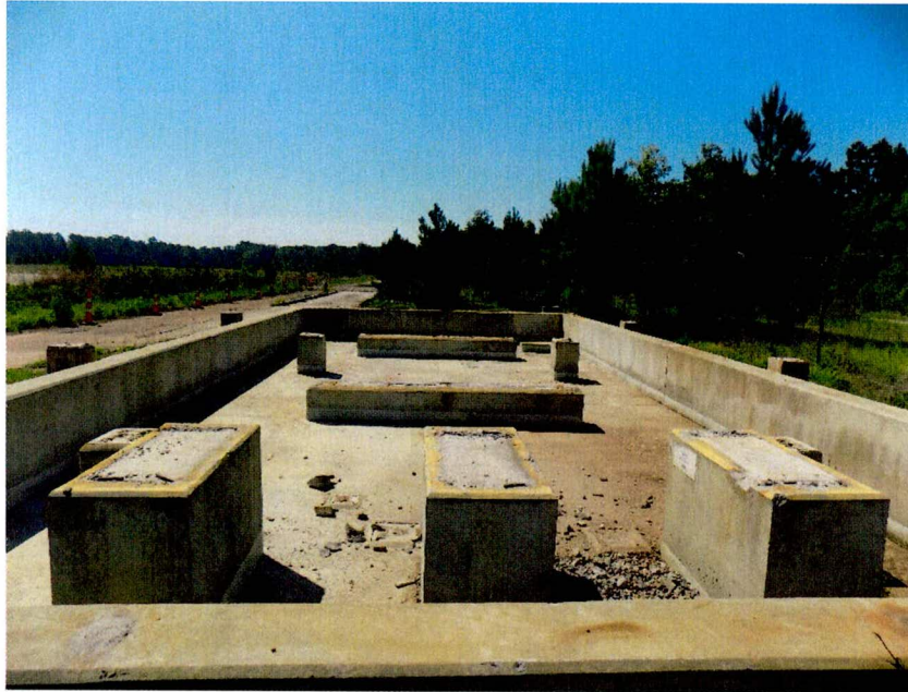
Figure 9. Building 454-D Slab (Looking South) After Final Decommissioning
