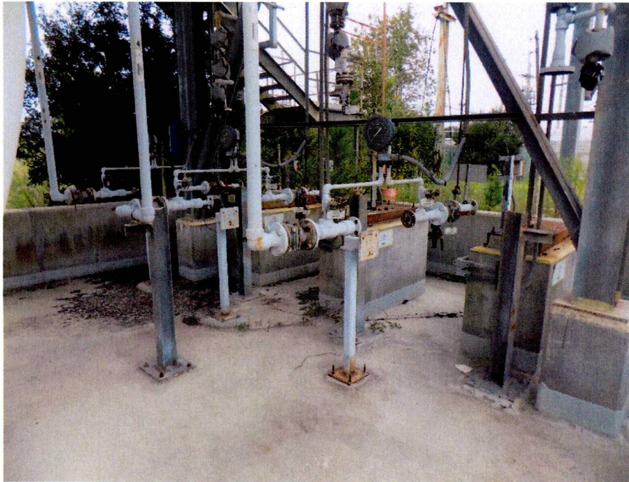
Figure 1. Building 454-D Slab (Looking Northwest) Before
