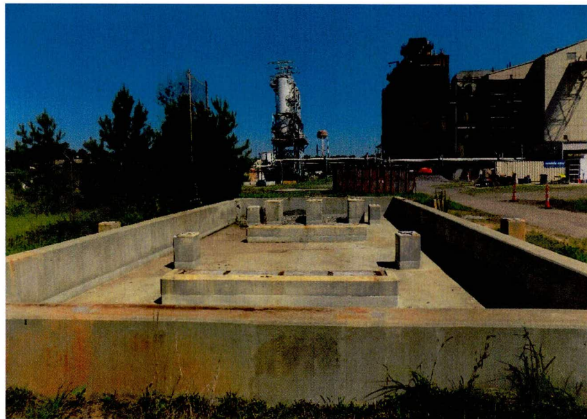
Figure 8. Building 454-D Slab (Looking North) After Final Decommissioning
