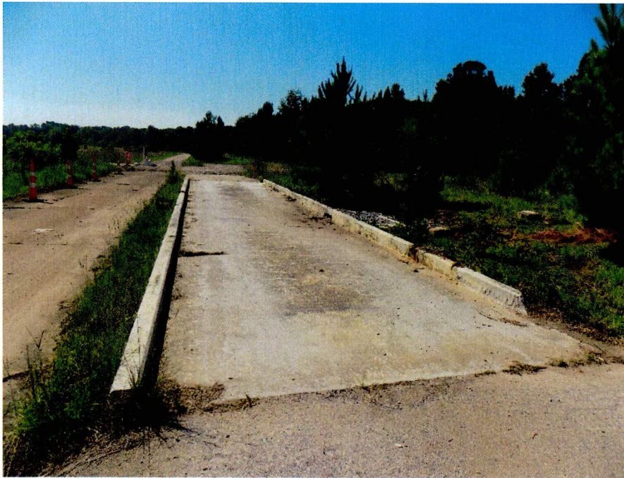
Figure 11. Building 454-1D (Looking South) After
