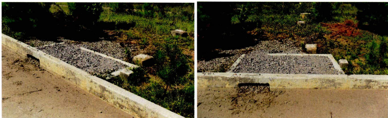
Figure 12. Building 454-1D Sump Filled with Gravel (Looking West) After
