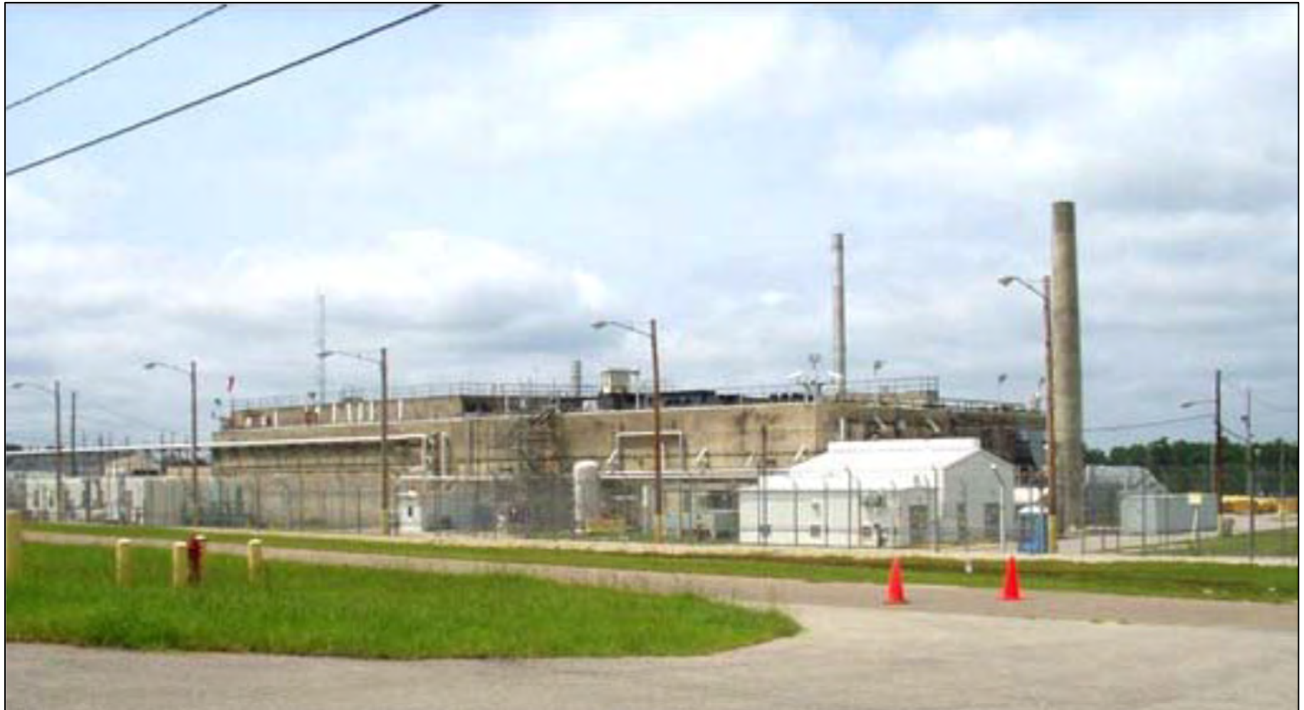
Figure 4. Historical Photograph of Building 235-F (Prior to 293-F Stack Reduction)
