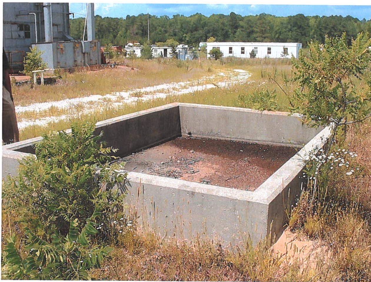
Figure 4 -Fuel Oil Tank Concrete Containment Dike (Looking East)
