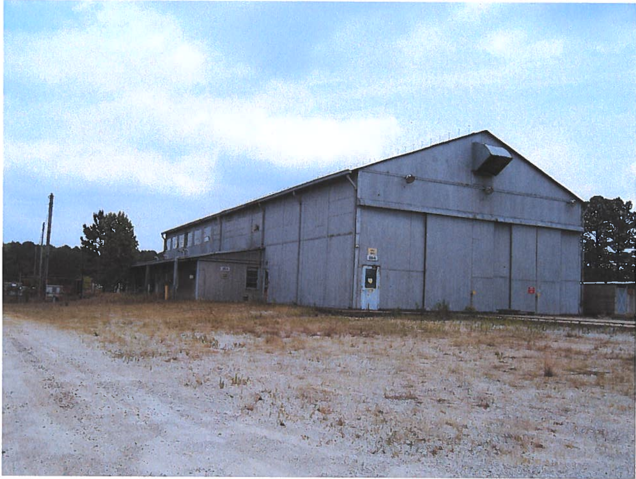
Figure 1 – Building 690-N, Process Heat Exchanger Repair Facility (Looking Southeast)
