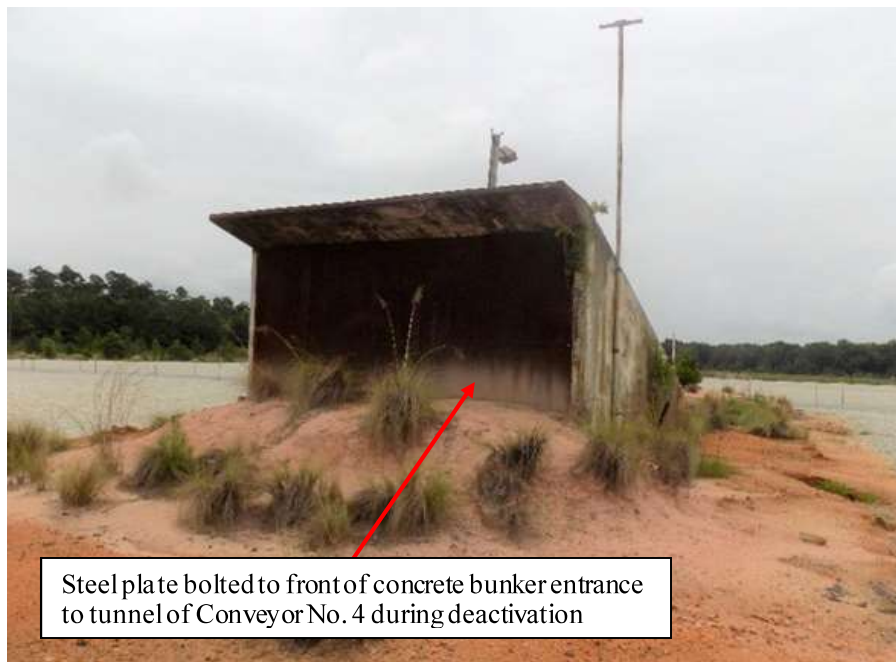
Figure 11. Concrete Bunker Entrance to Conveyor No. 4 Tunnel
