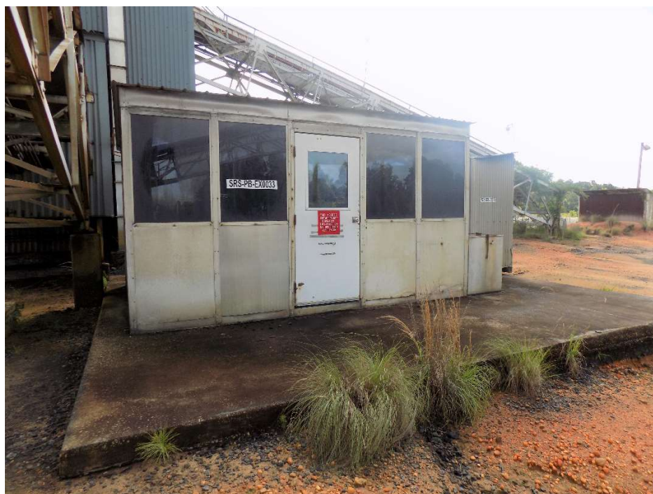
Figure 12. SRS-PB-EX0033 Coal Handling Breakroom Building for Crusher House
