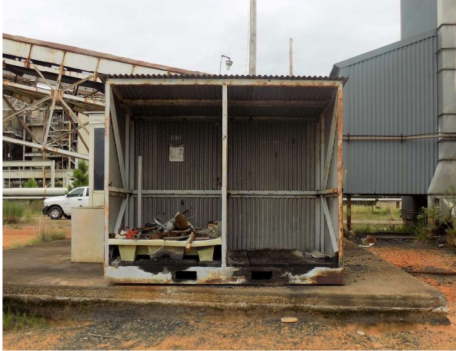
Figure 13. SRS-PB-EX0035 Storage Shed for Portable Equipment, Lube and Spare Parts
