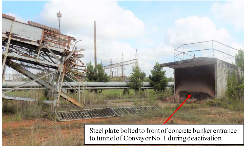
Figure 8. Conveyor No. 1 (cut) and Bunker Entrance to Conveyor No. 1 Tunnel
