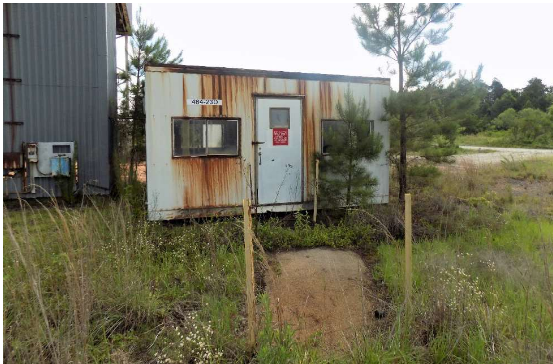
Figure 6. 484-23D Coal Handling Breakroom Building (aka SRS-PB-EX0032)
