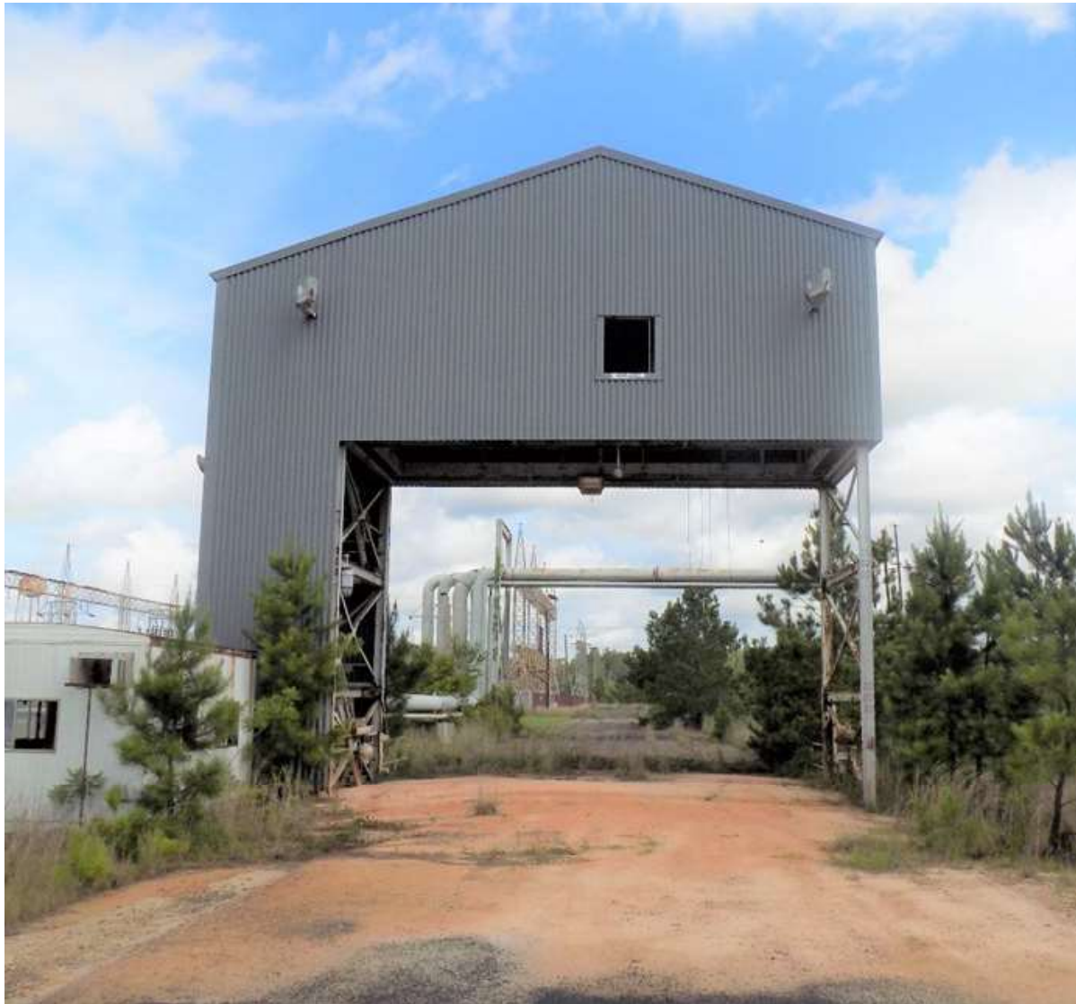
Figure 4. 484-24D Coal Handling Shaker House
