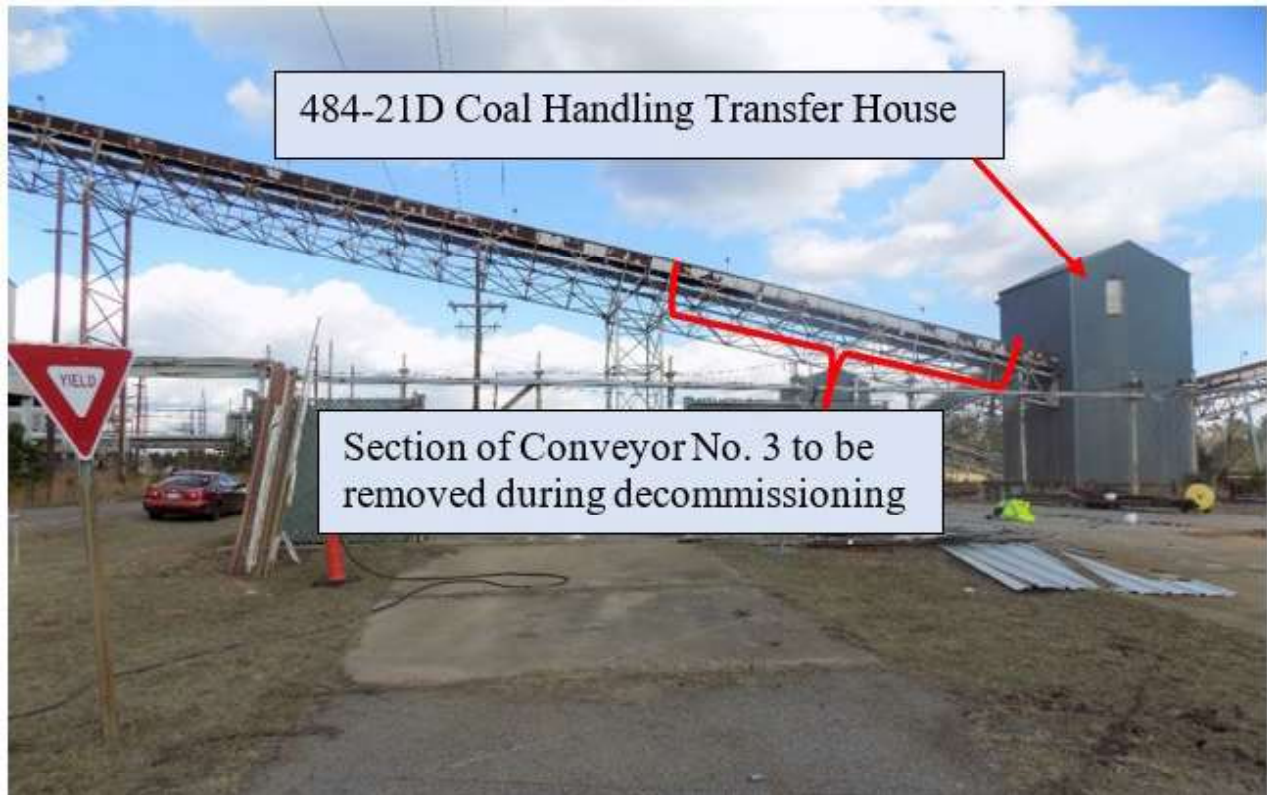
Figure 17. Section of Conveyor No. 3 to be Decommissioned as Part of This Project
