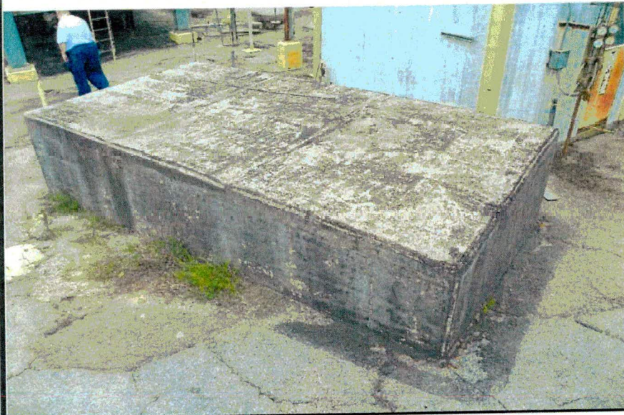
Tank 19, Underliner Sump Access Port
