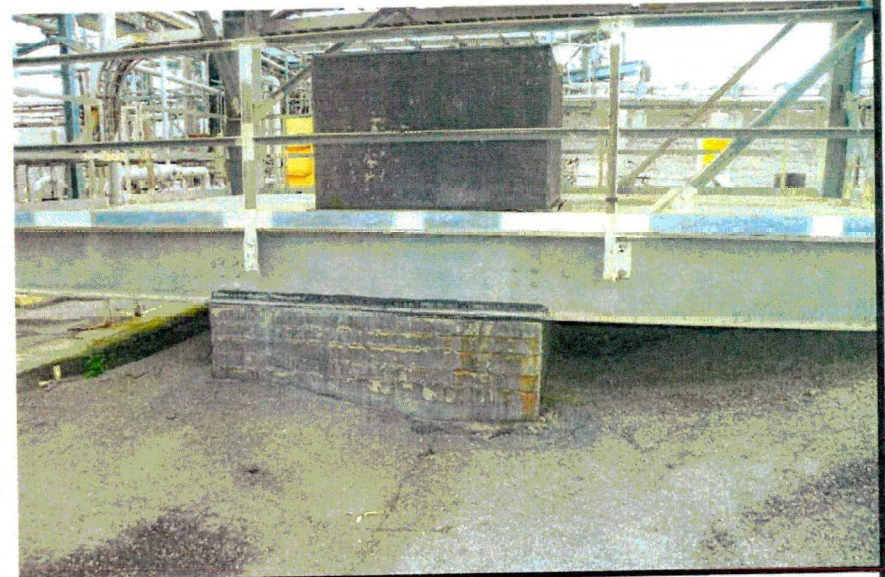
Tank 19, East Riser
