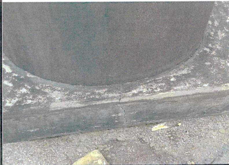
Tank 19, Northwest Riser (Crack on South Side)
