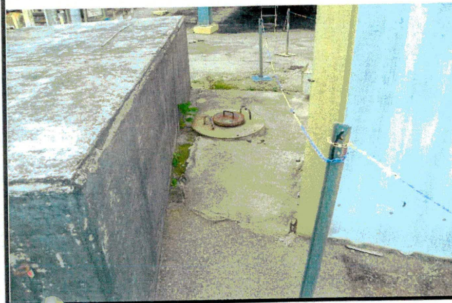
Tank 19, Underliner Sump Access Port
