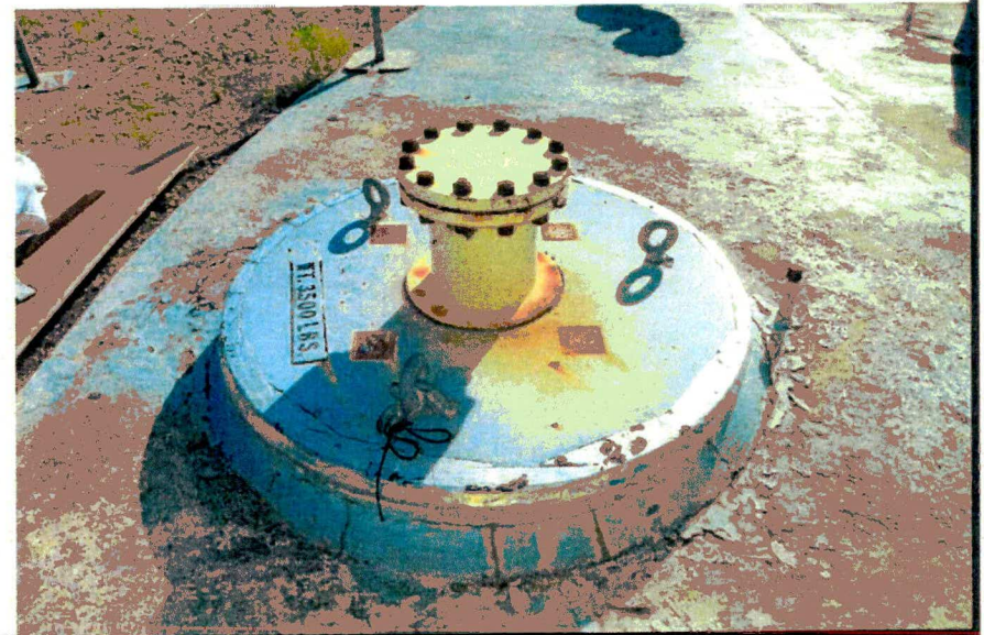
Tank 16, North Annulus Riser
