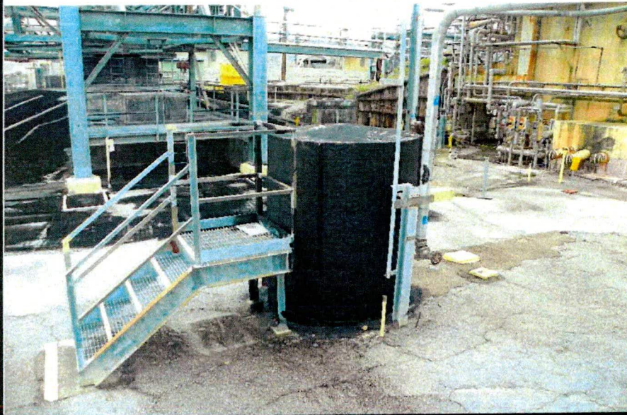
Tank 17, East Riser
