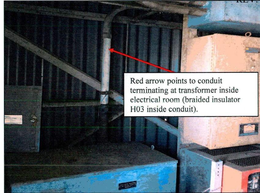
Photograph 5. View of transformer and conduit inside electrical room.
