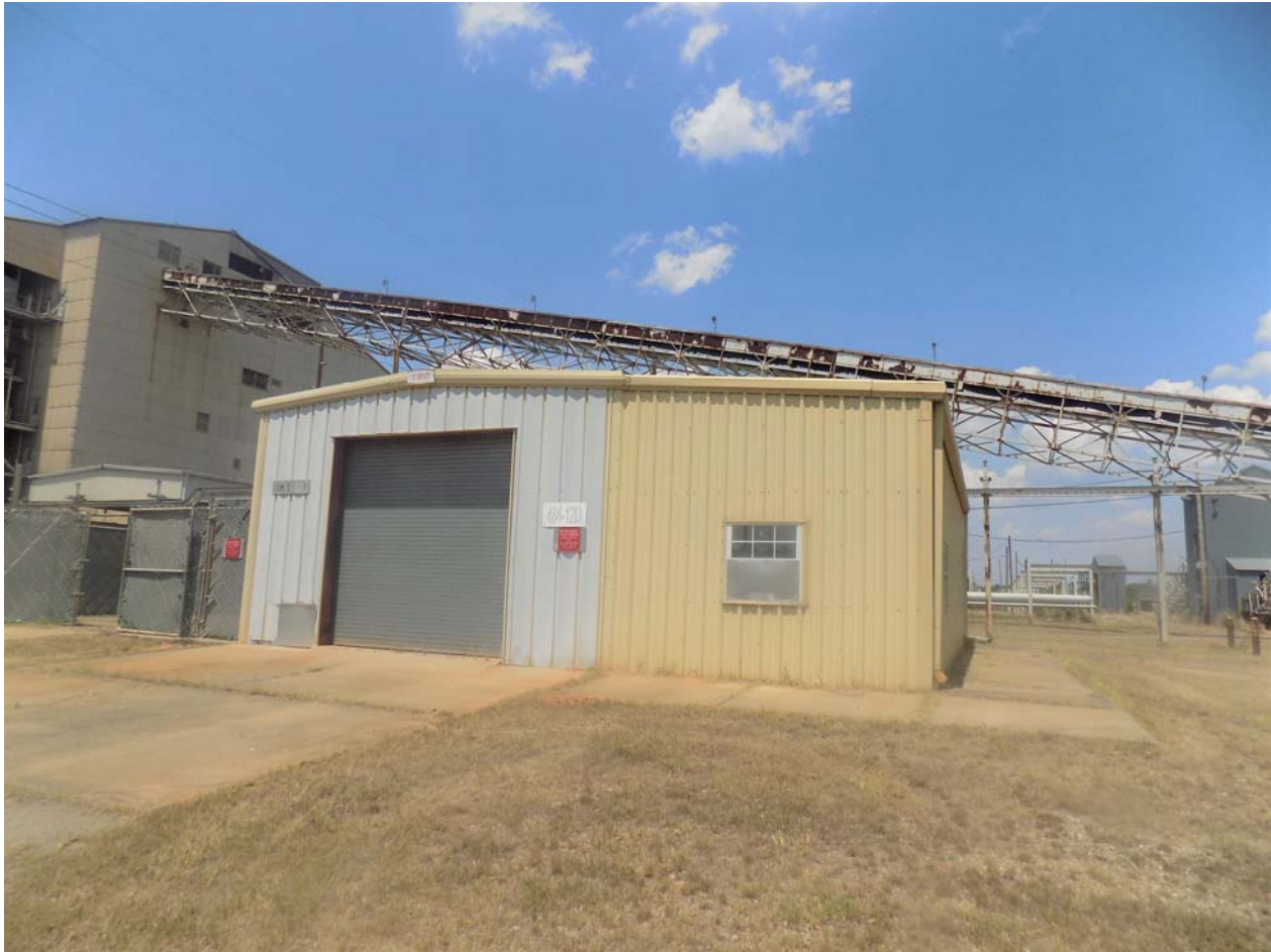
Figure 1. Building 484-12D, D-Area Storage Building
