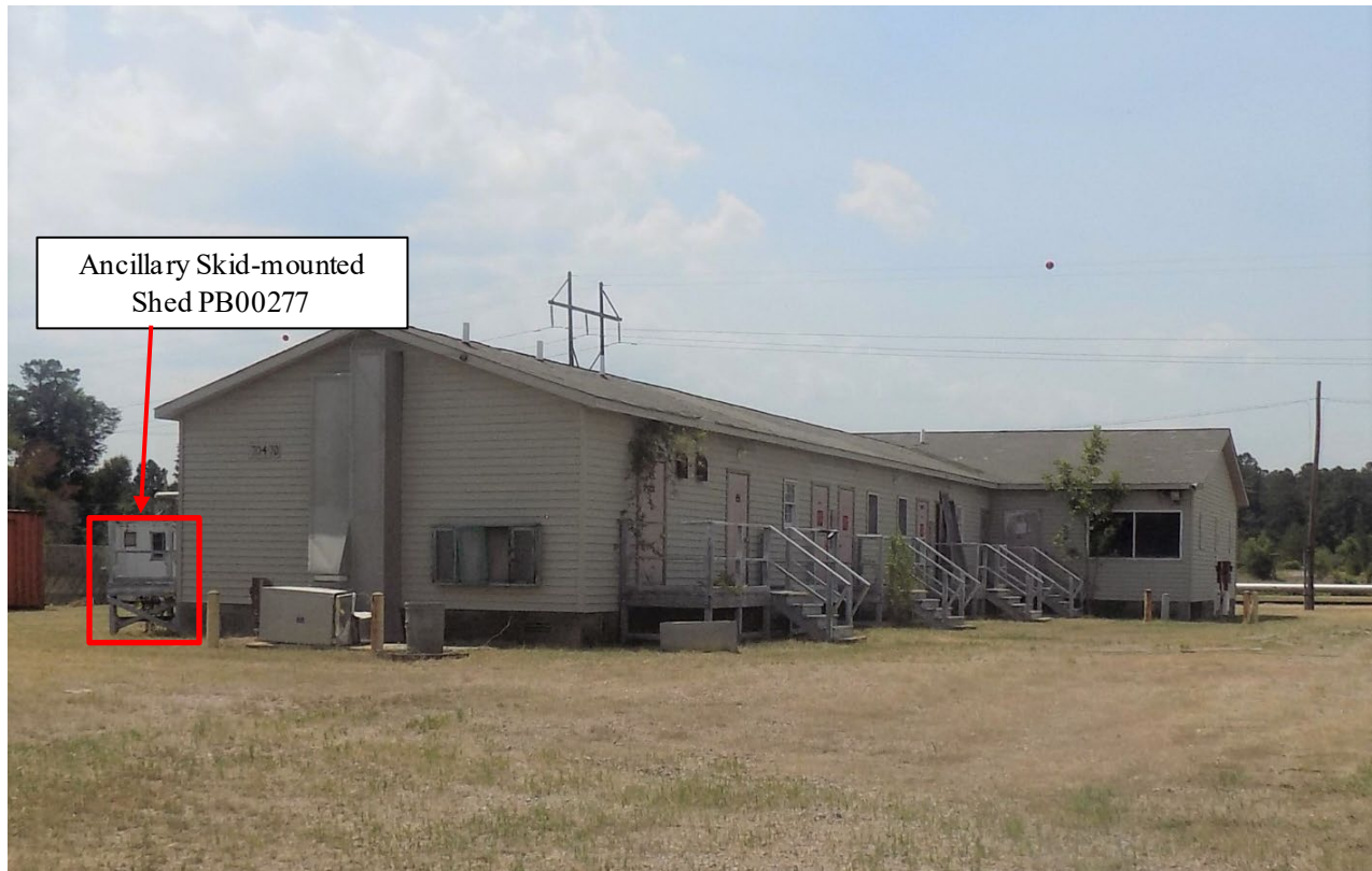
Figure 1. Building 704-7D (Looking Northwest) Before Decommissioning
