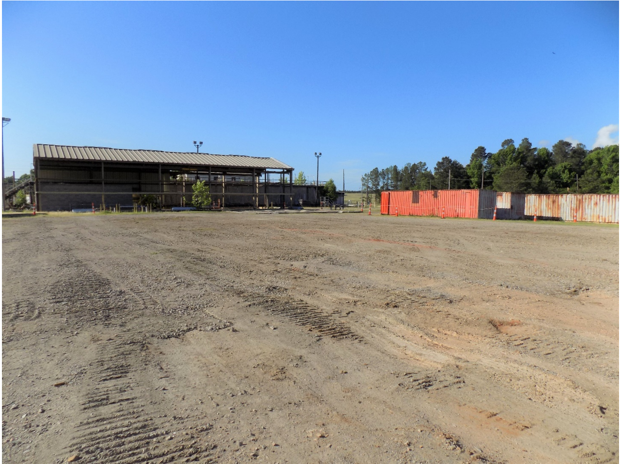
Figure 2. Building 704-7D (Looking Southwest) After Decommissioning
