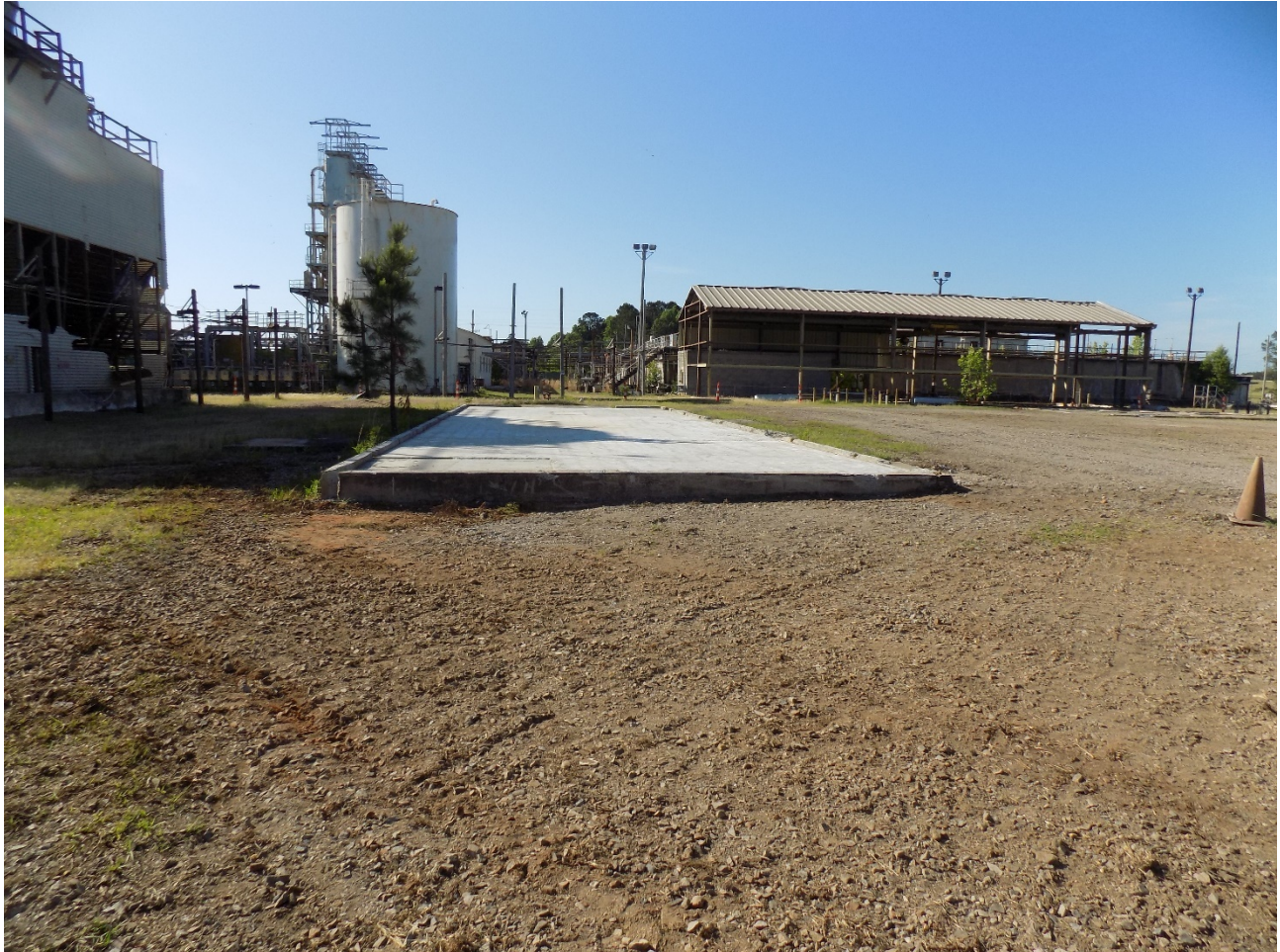
Figure 2. Building 717-3D (Looking South) After Decommissioning
