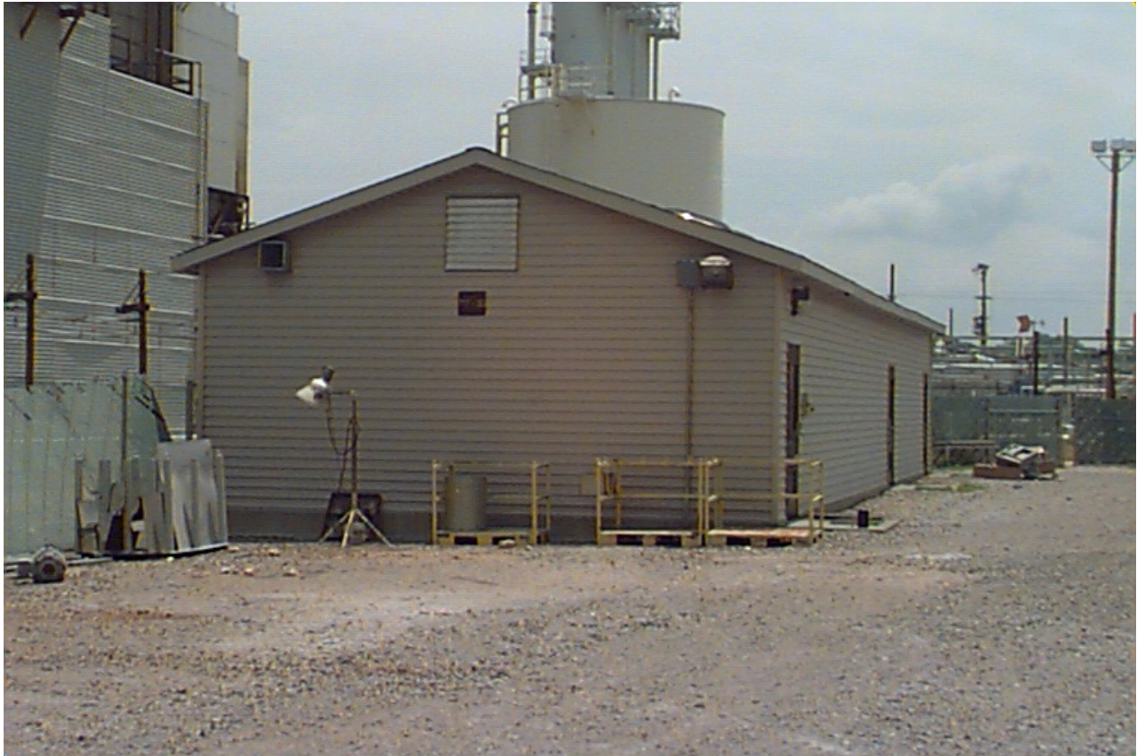
Figure 1. Building 717-3D (Looking South) Before Decommissioning
