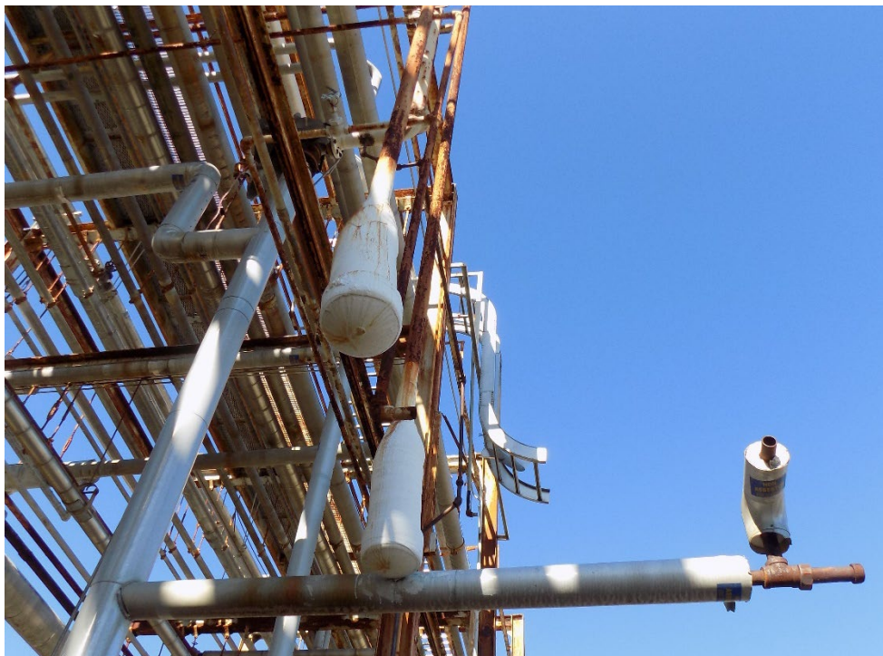
Photo 3 - Pipe Caps/Wraps Only
