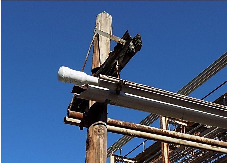
Photo 4 - Pipe Cap/Wrap Only
