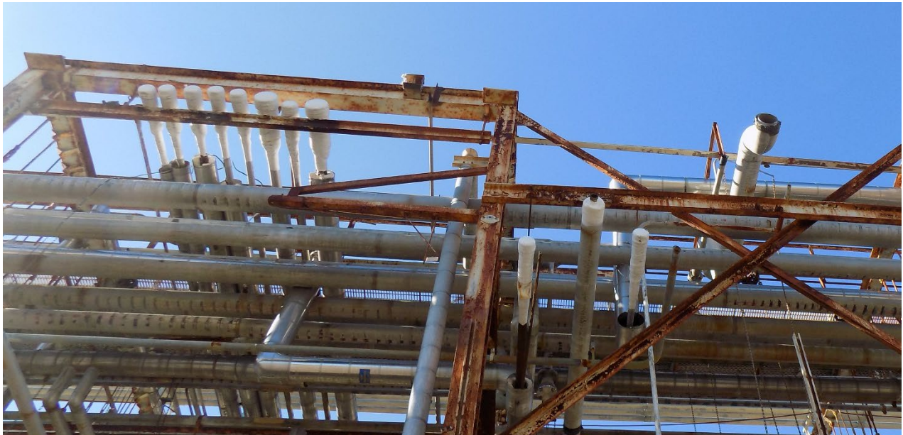
Photo 2 - Pipe Caps/Wraps Only
