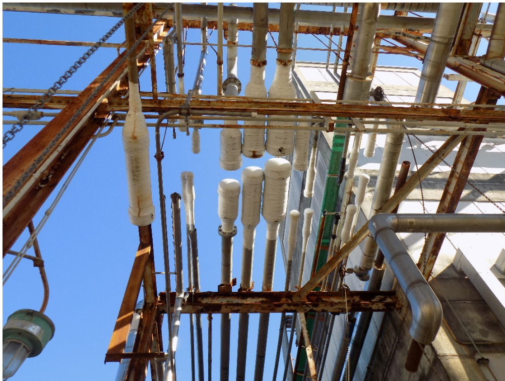
Photo 1 - Pipe Caps/Wraps Only
