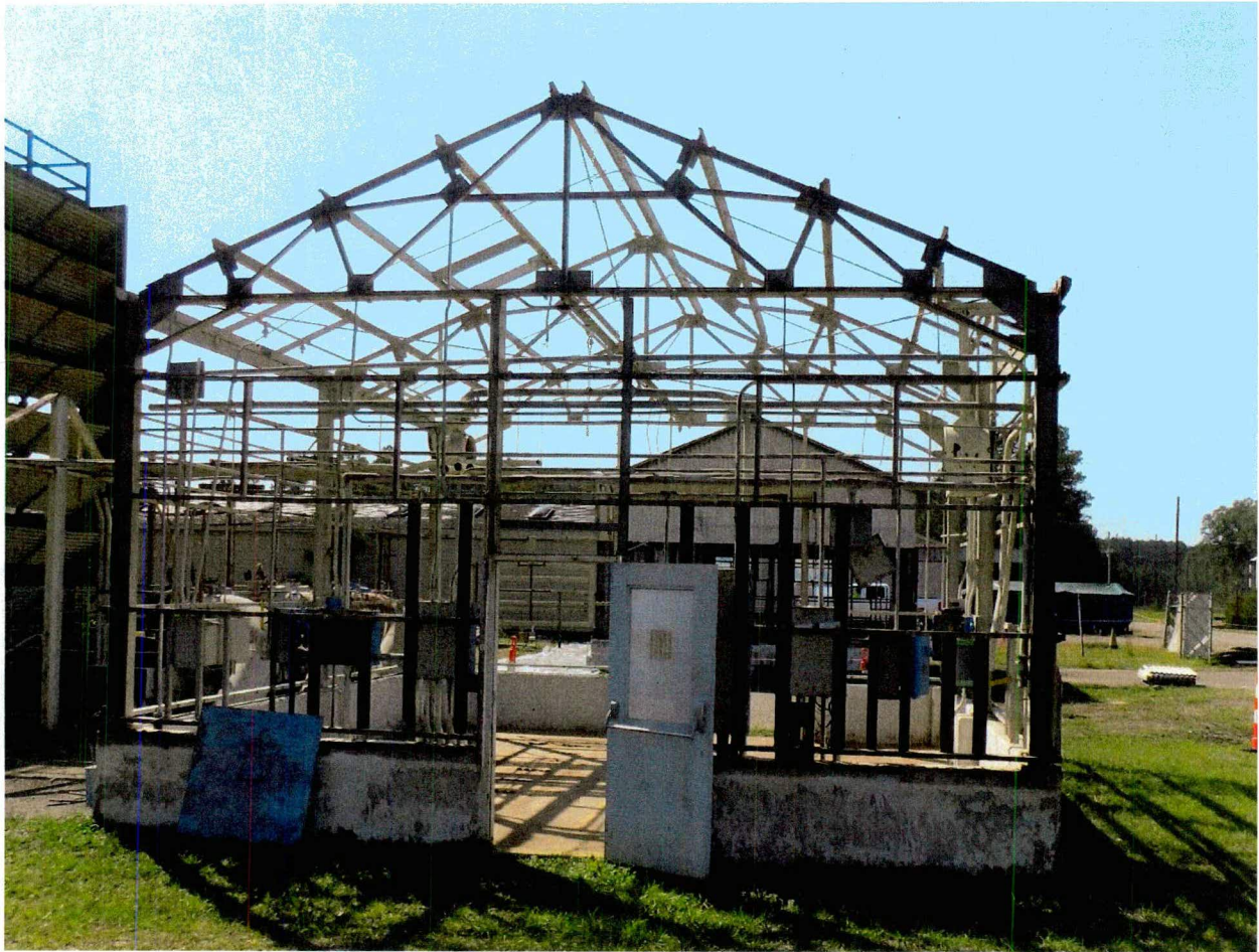
Figure 3: Photo of Building 482-2D Looking West (East Side of Building)
