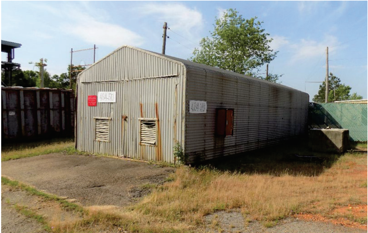
Figure 1: Building 484-5D (Looking Southwest) Before Decommissioning
