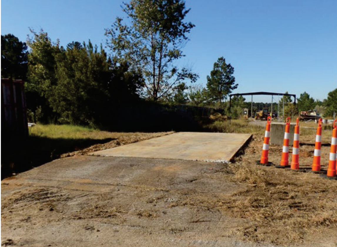
Figure 2: Building 484-5D (Looking West) After Decommissioning
