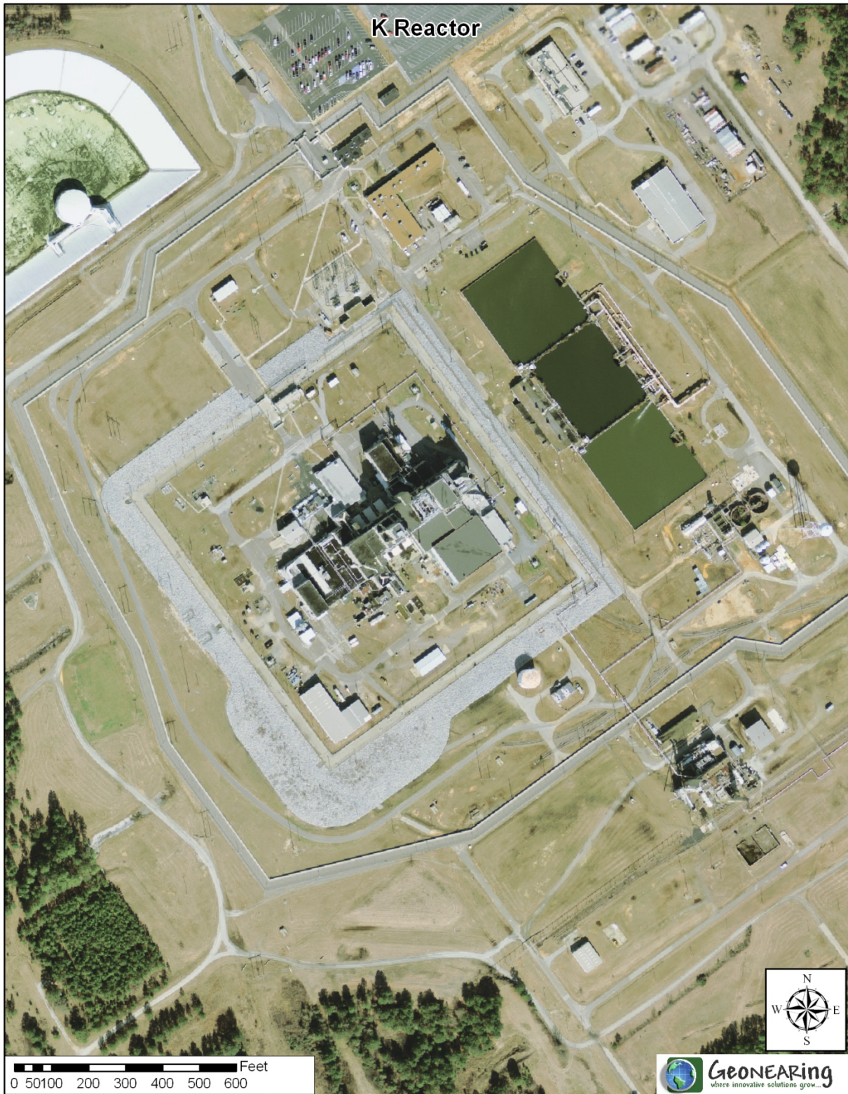
Figure D-5. Aerial View of the K-Reactor Complex (2010)
