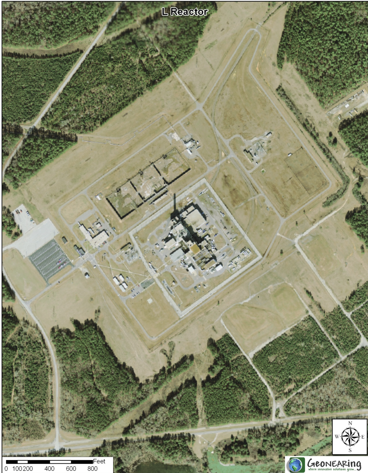
Figure D-6. Aerial View of the L-Reactor Complex (2010)
