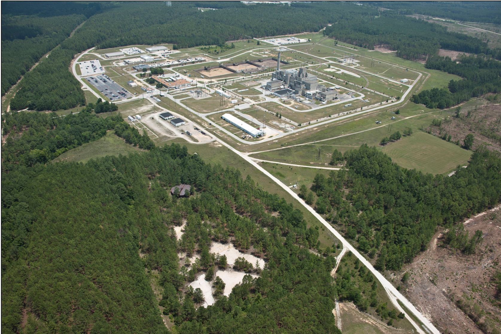
Figure C-2. Aerial Photograph of CAOU (2011)
