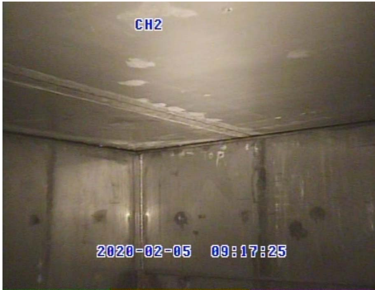
Walls and cell covers free of accumulated solids
