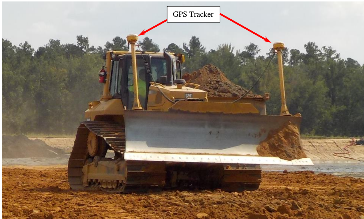
Photo 4. Dozer (Cat D-6)
