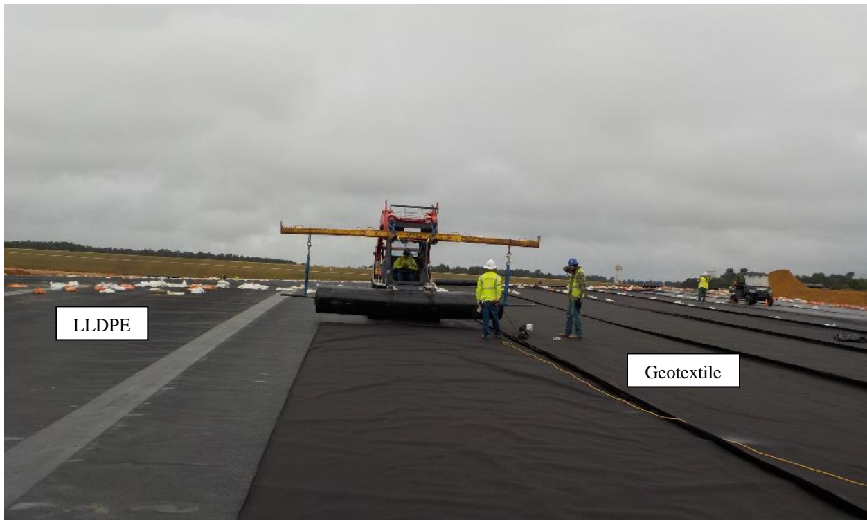
Photo 84. Geotextile Placement over the LLDPE Geomembrane (2)
