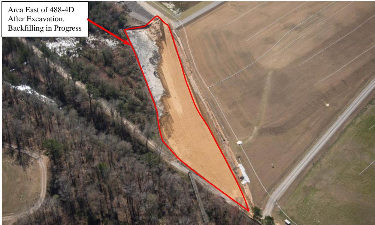
Photo 27. Area East of 488-4D Ash Landfill (February 2017)
