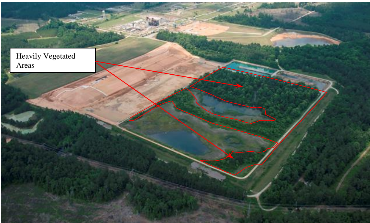
Photo 44. 488-1D Ash Basin Prior to Any Clearing of Trees (May 2016)
