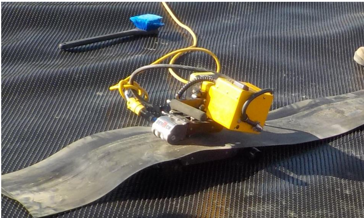
Photo 18. Hot Wedge Dual Track Welder
