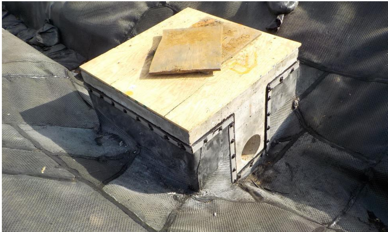
Photo 78. Typical LLDPE Tie into Catch Basin
