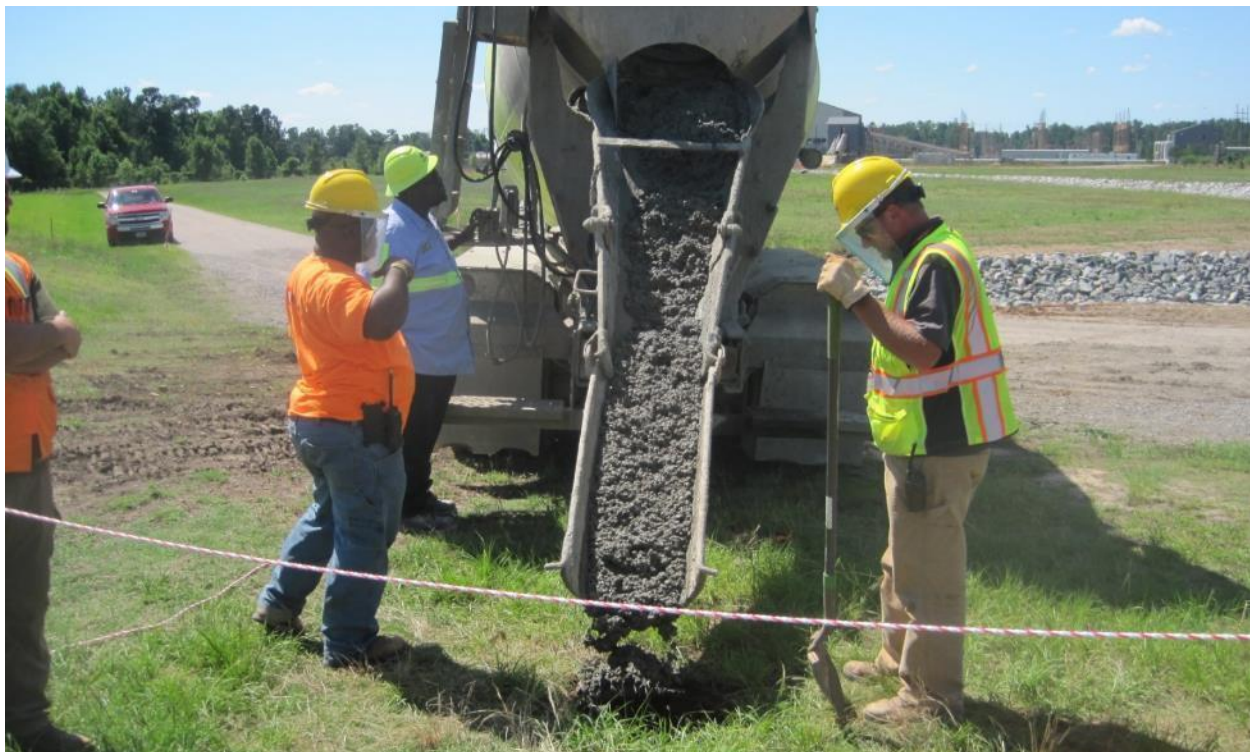
Photo 36. 489-D CPRB Plugging of Upgradient Manholes
