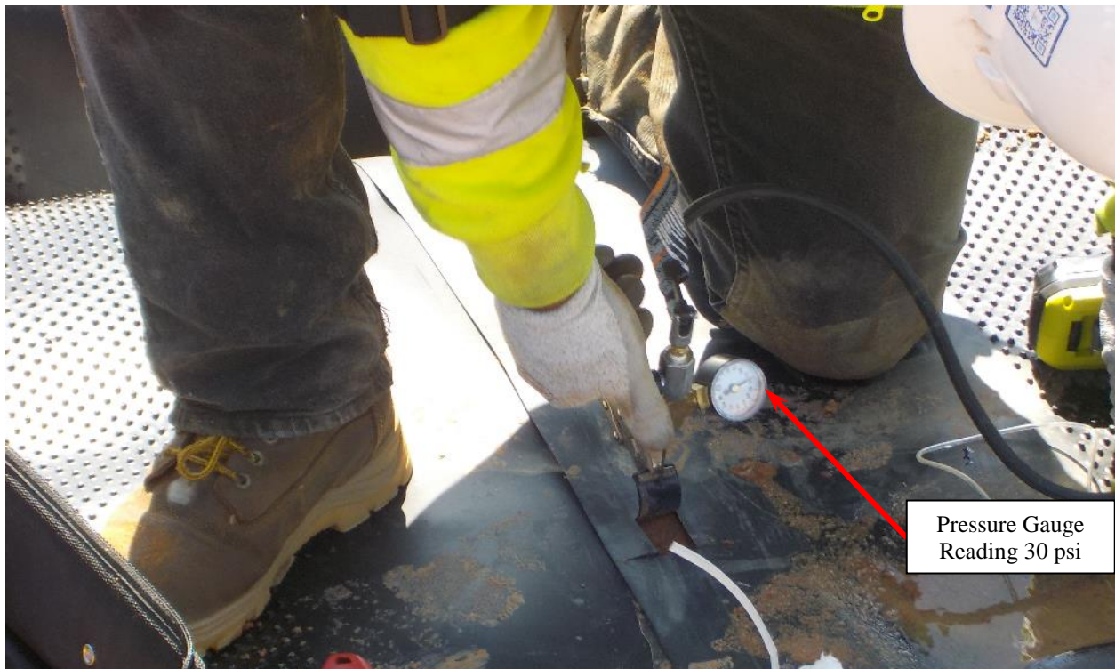
Photo 80. LLDPE Air Pressure Testing of Dual Hot Wedge Seam (Non-Destructive)
