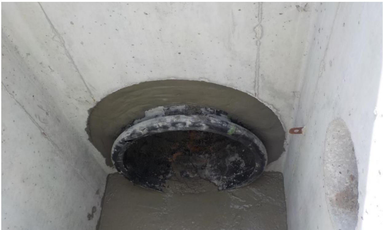
Photo 66. 488-1D Ash Basin Interior of Catch Basin Typical Grouted 24" Culvert
