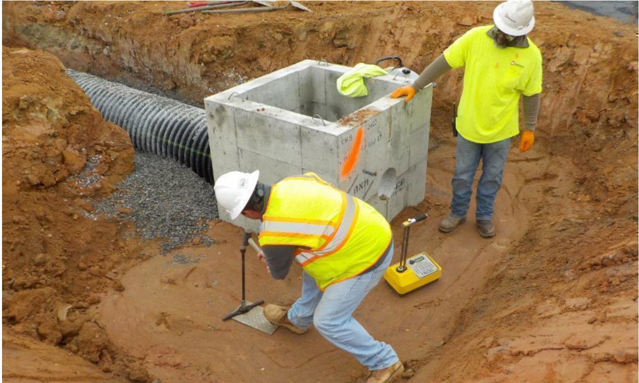
Photo 65. 488-1D Ash Basin Typical Compaction Testing around Utilities
