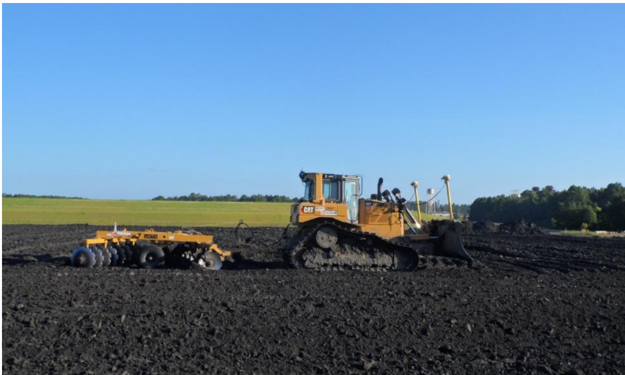
Photo 54. Disking of Ash to Allow for Additional Drying 488-1D Ash Basin (East End)
