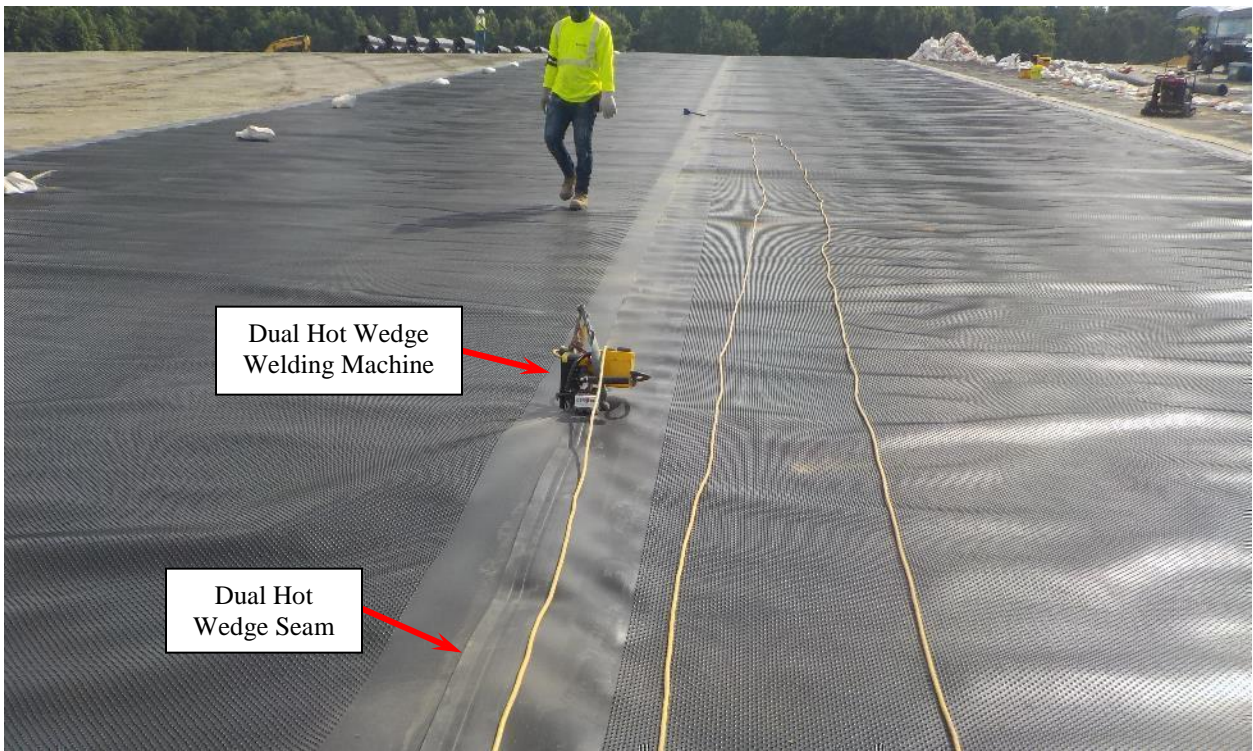
Photo 74. LLDPE Geomembrane Dual Hot Wedge Seaming (Production Seam)
