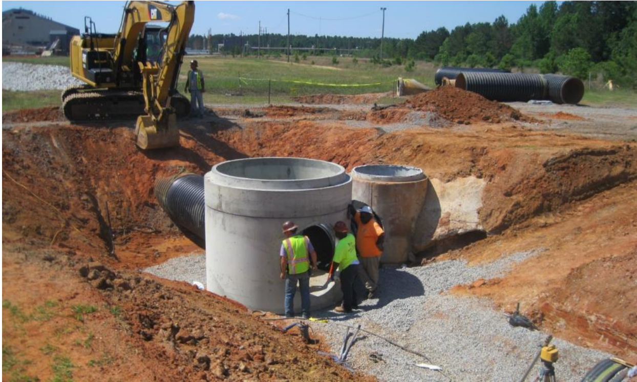
Photo 41. 489-D CPRB New Manhole in Place
