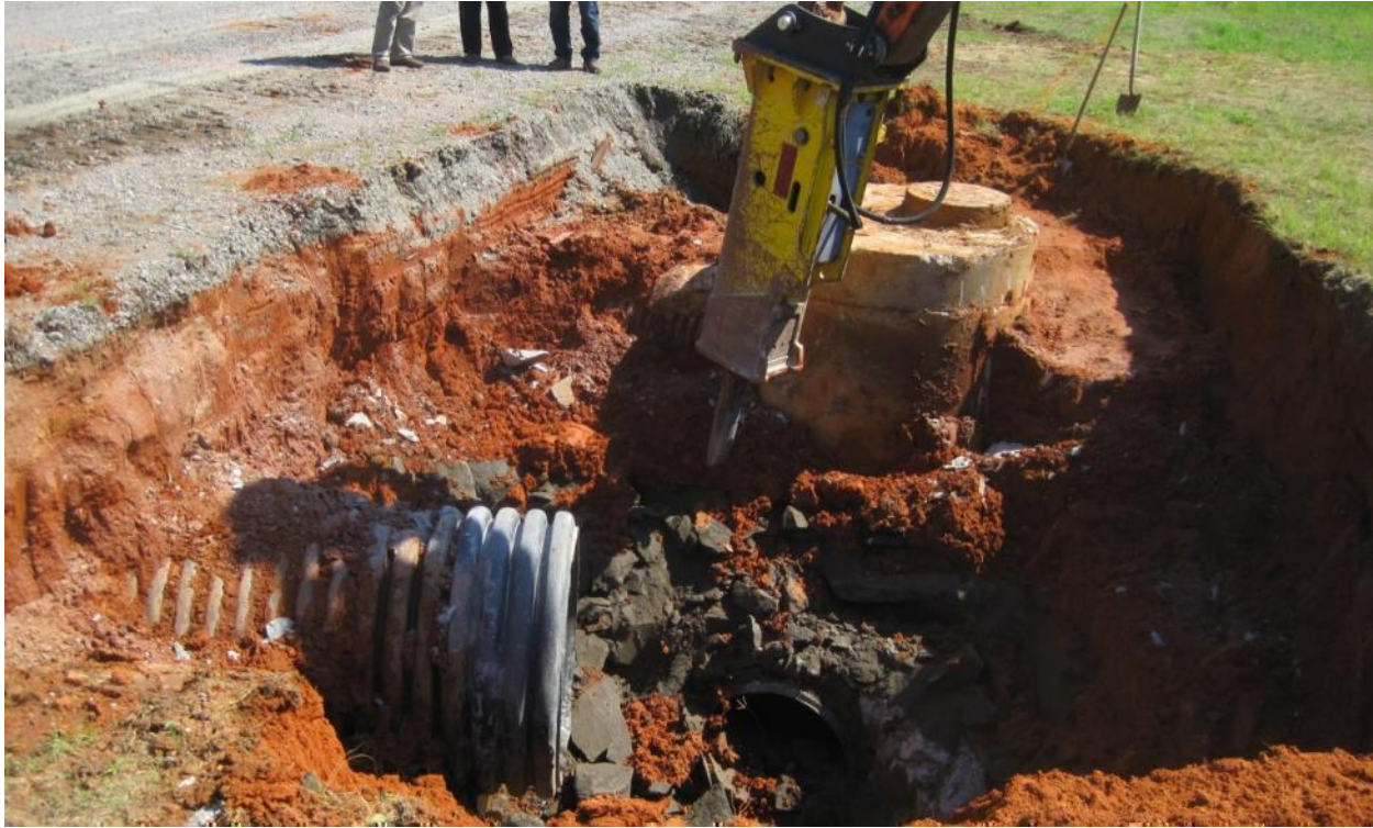
Photo 39. 489-D CPRB Removal of Existing Manhole
