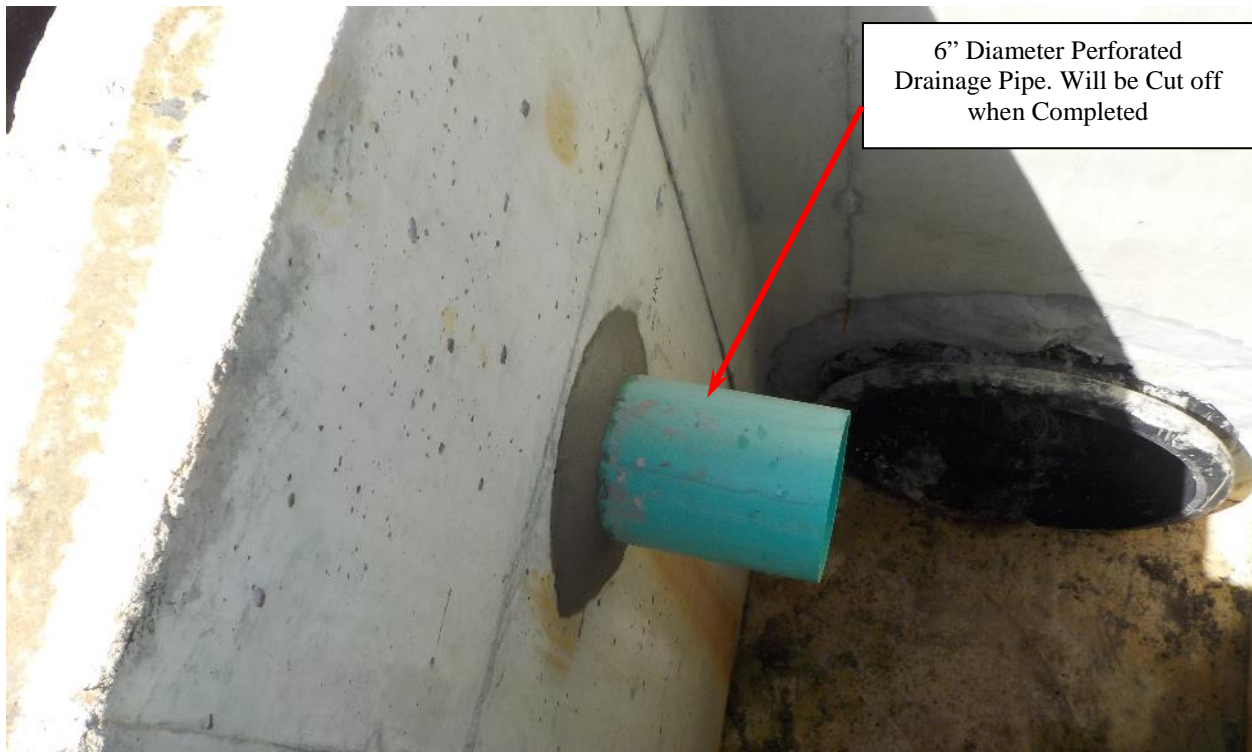
Photo 88. Grouted Subsurface Drainage Pipe in Catch Basin
