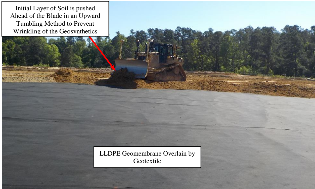
Photo 89. 488-1D Ash Basin East 20 Inch Soil Cover Placement
