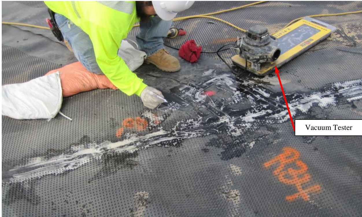
Photo 81. LLDPE Vacuum Testing of Extrusion Welds (Non- Destructive)
