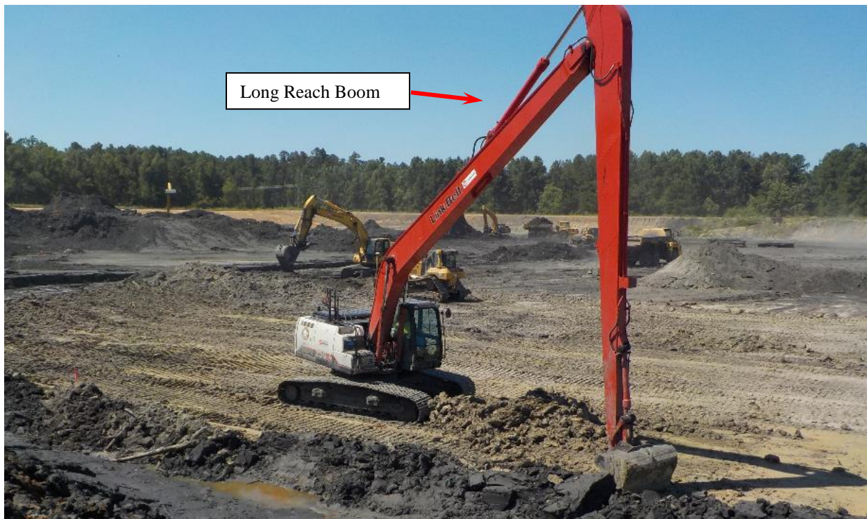
Photo 6. Long Reach Excavator
