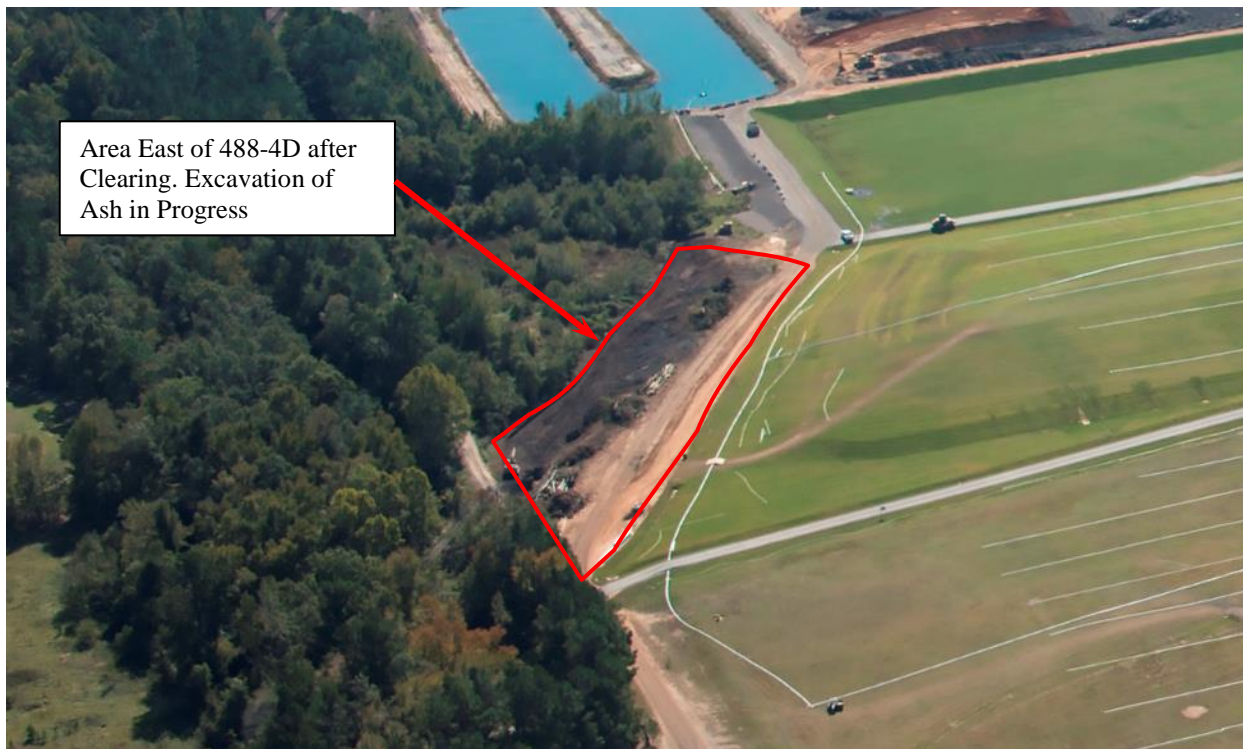
Photo 26. Area East of 488-4D Ash Landfill (October 2016)
