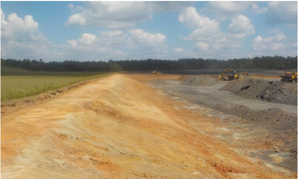
Photo 52. 488-1D Ash Basin Northern Berm Face Visually Clean of Ash
