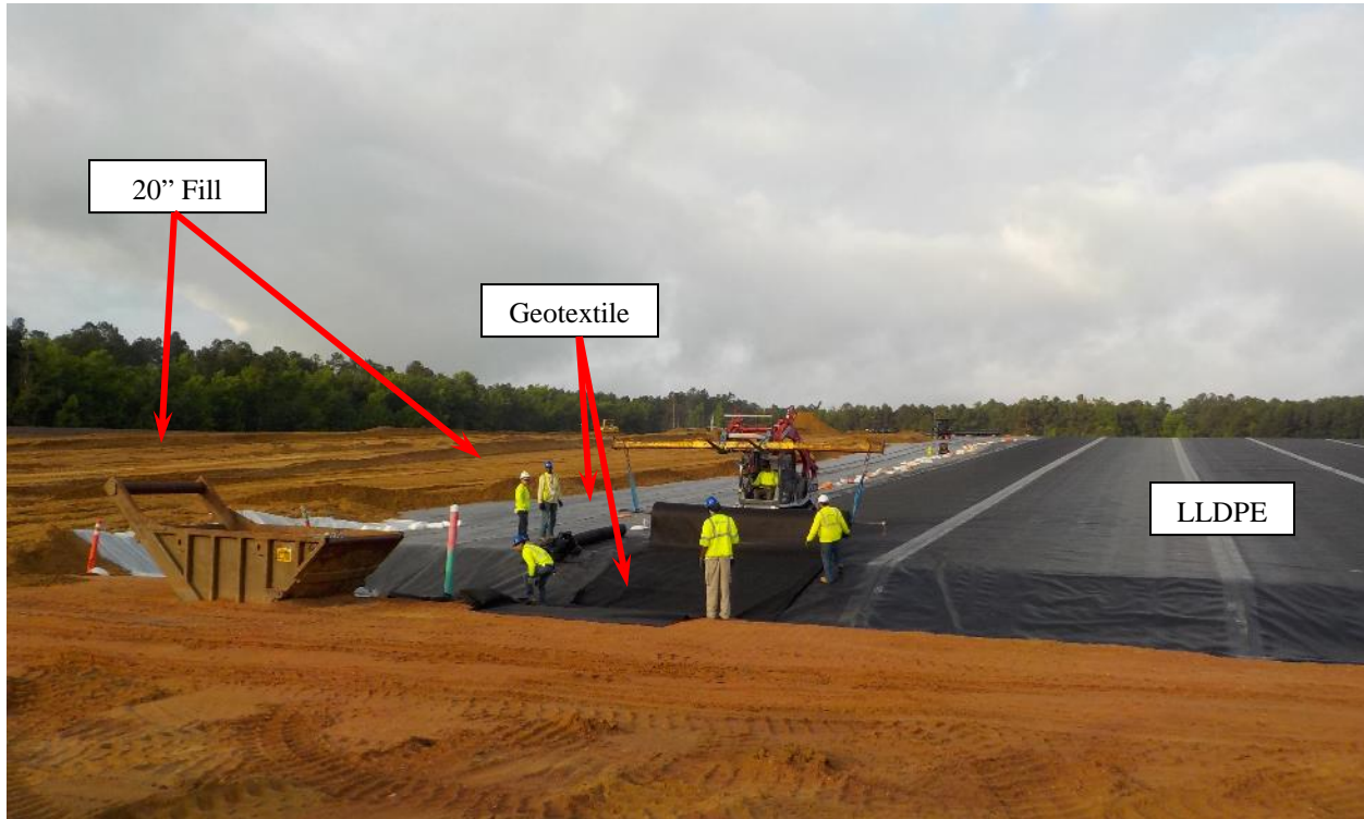
Photo 83. Geotextile Placement over the LLDPE Geomembrane (1)
