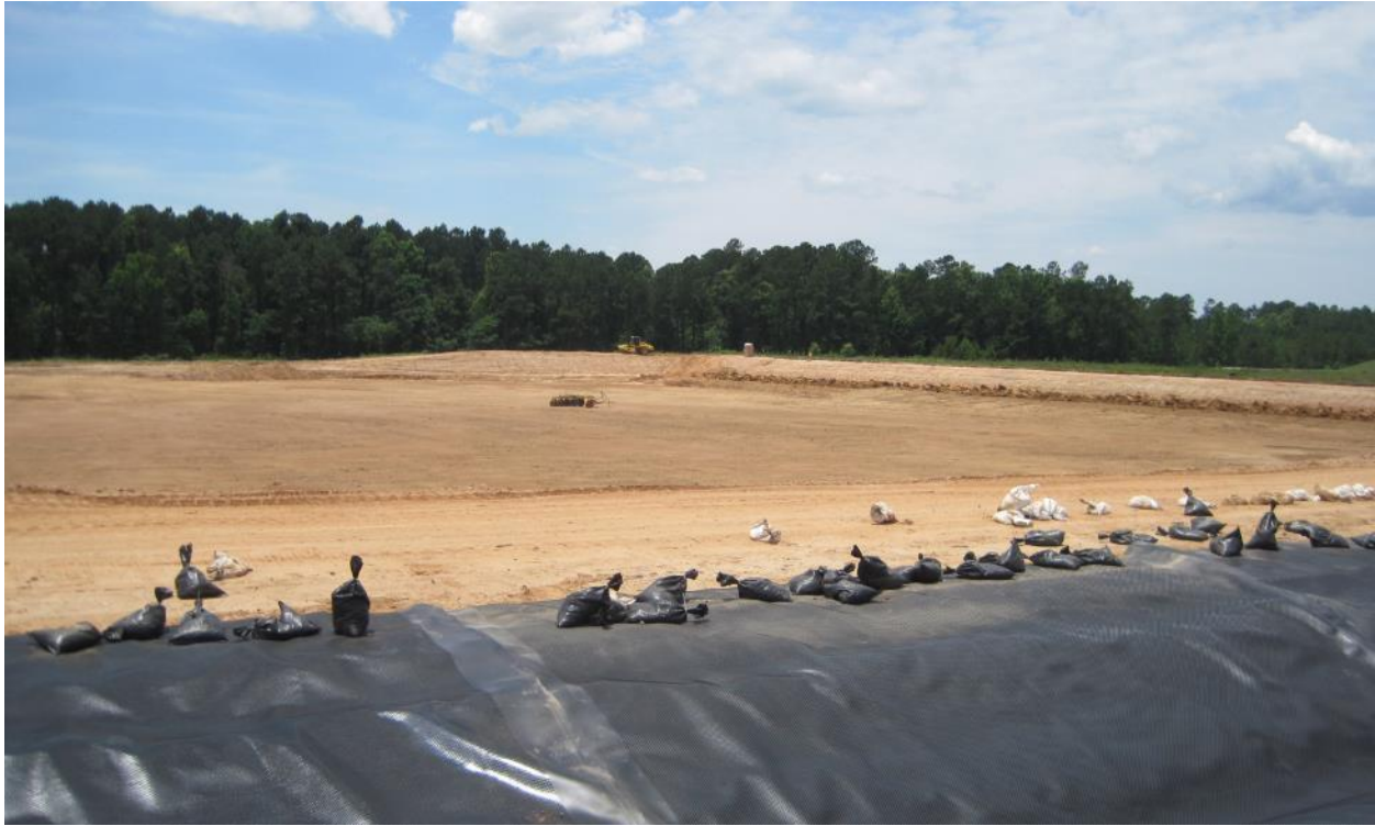
Photo 61. Backfill 488-1D Ash Basin West
