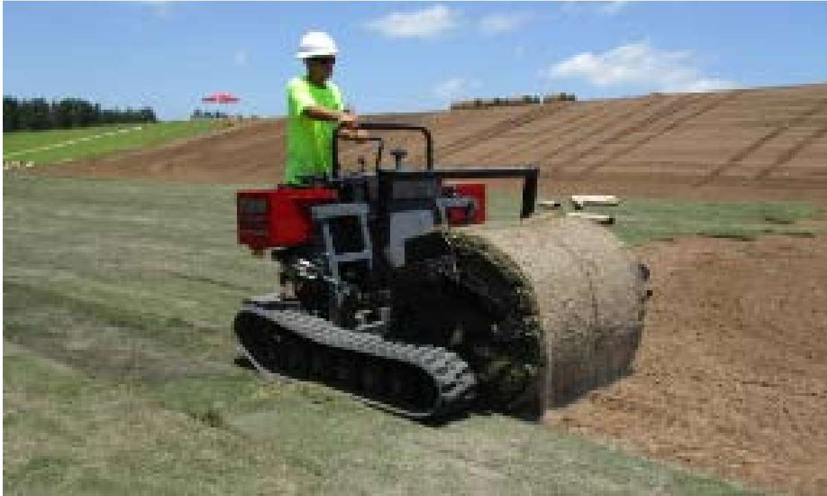
Photo 17. Tracked Sod Installer
