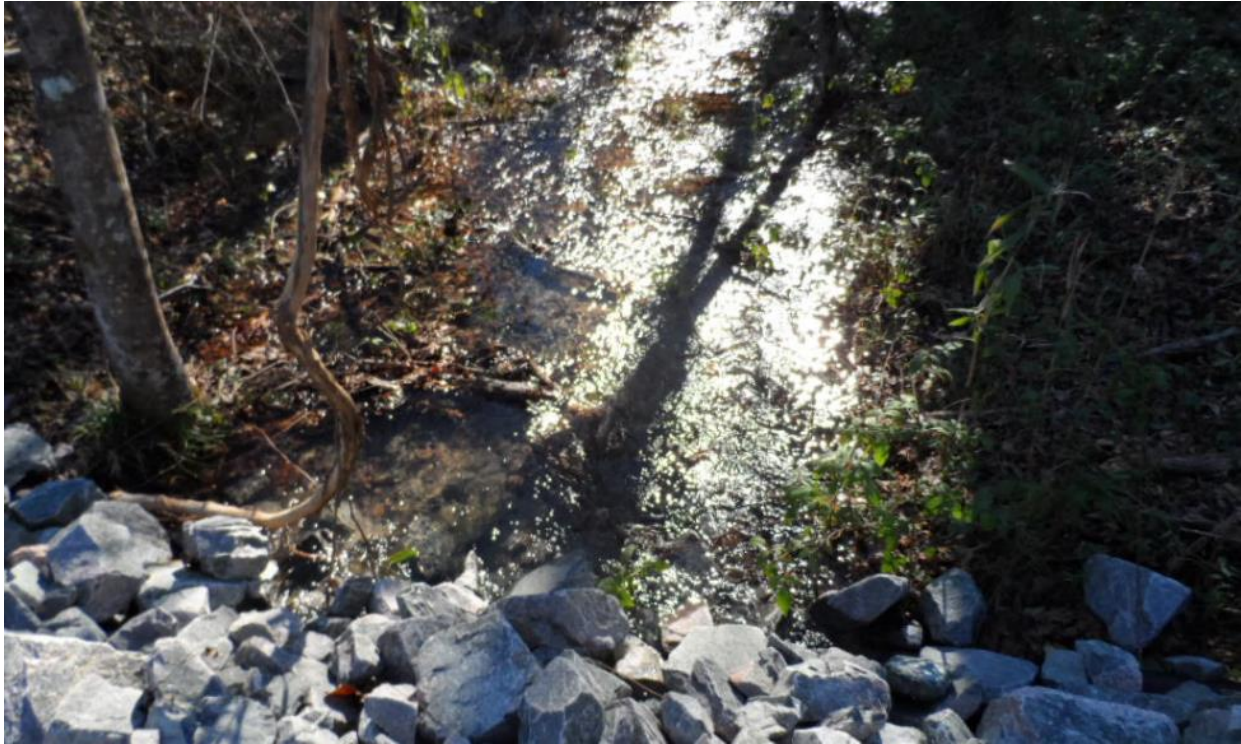
Photo 23. Stormwater Discharge through Check Dam
