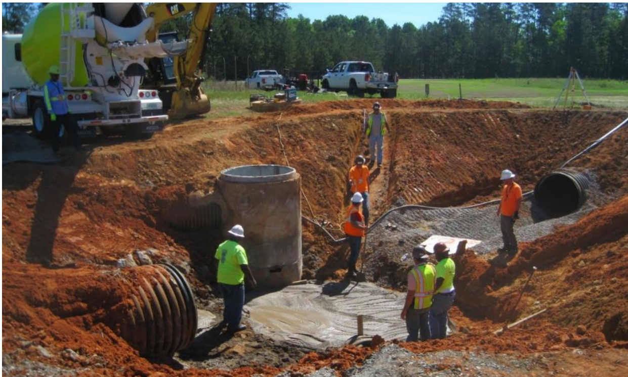
Photo 40. 489-D CPRB Prepping for Placement of New Manhole
