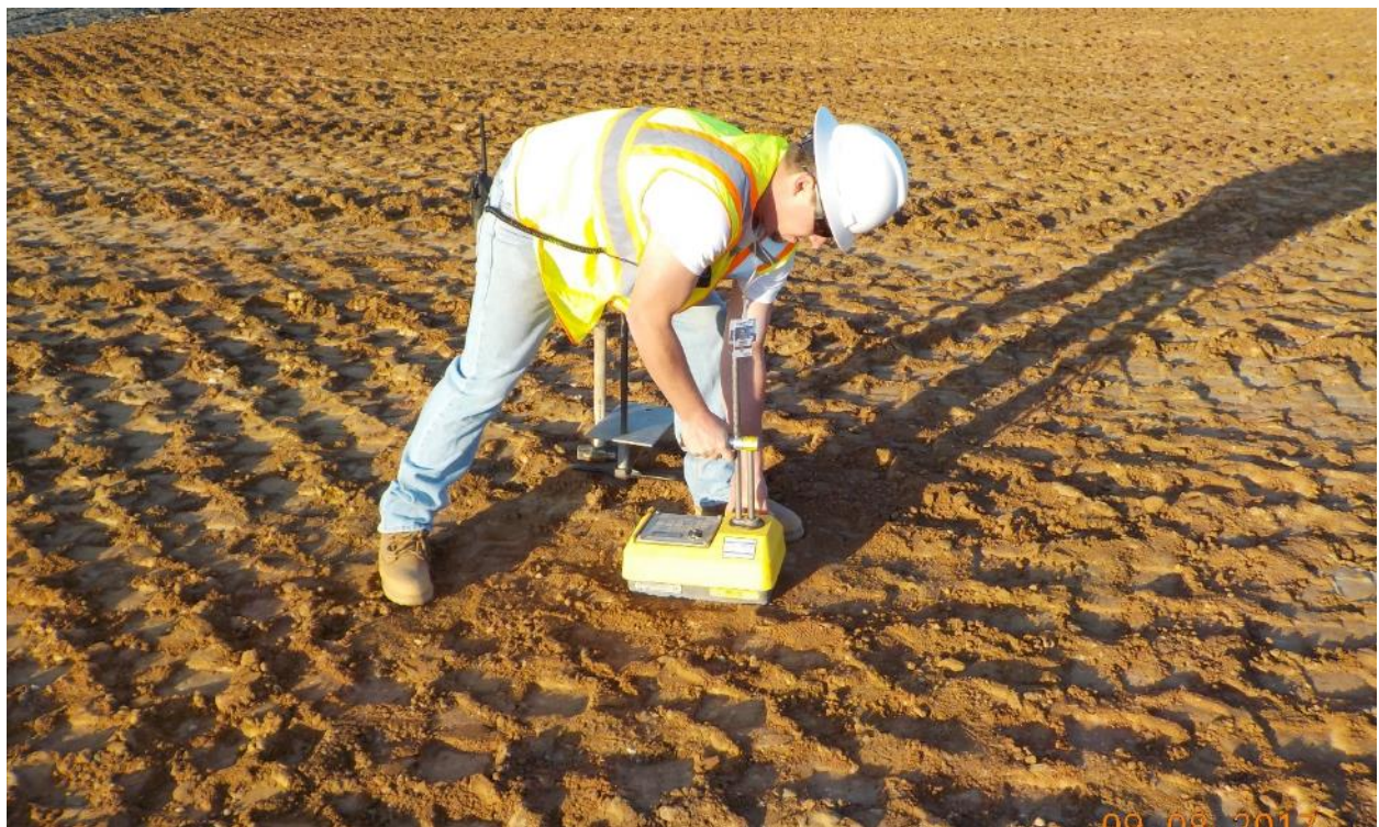
Photo 60. 488-1D Ash Basin Compaction Testing New Western Berm
