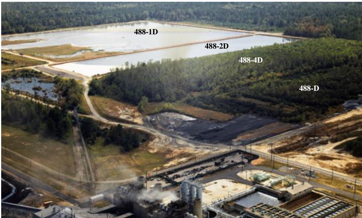
Photo 2. Historical Photo of D-Area (1984)
