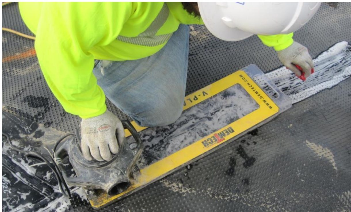
Photo 21. Vacuum Testing of Extrusion Weld
