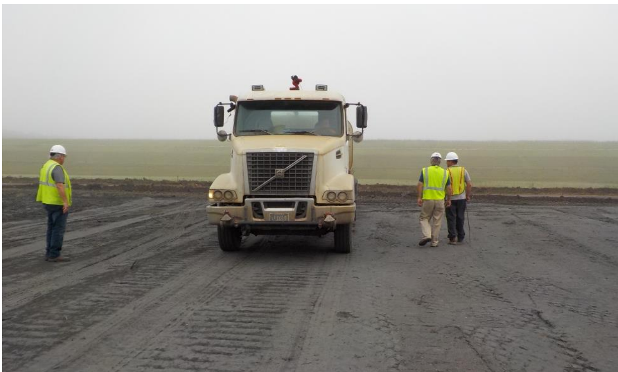
Photo 56. Proof Roll Inspection
