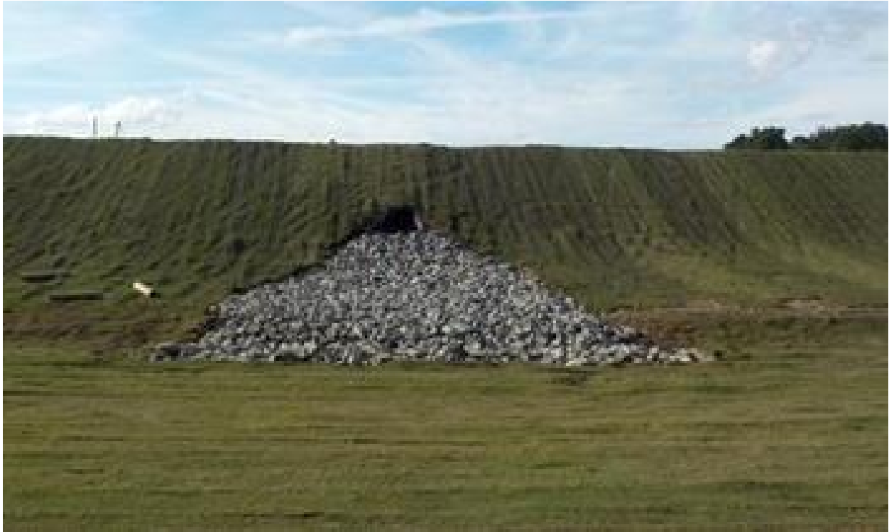
Photo 67. Typical RipRap Apron
