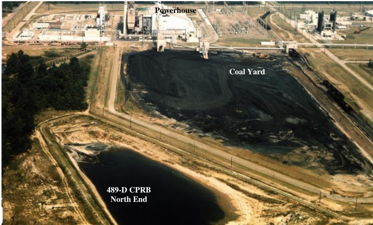
Photo 1. Historical Photo of D-Area (1982)
