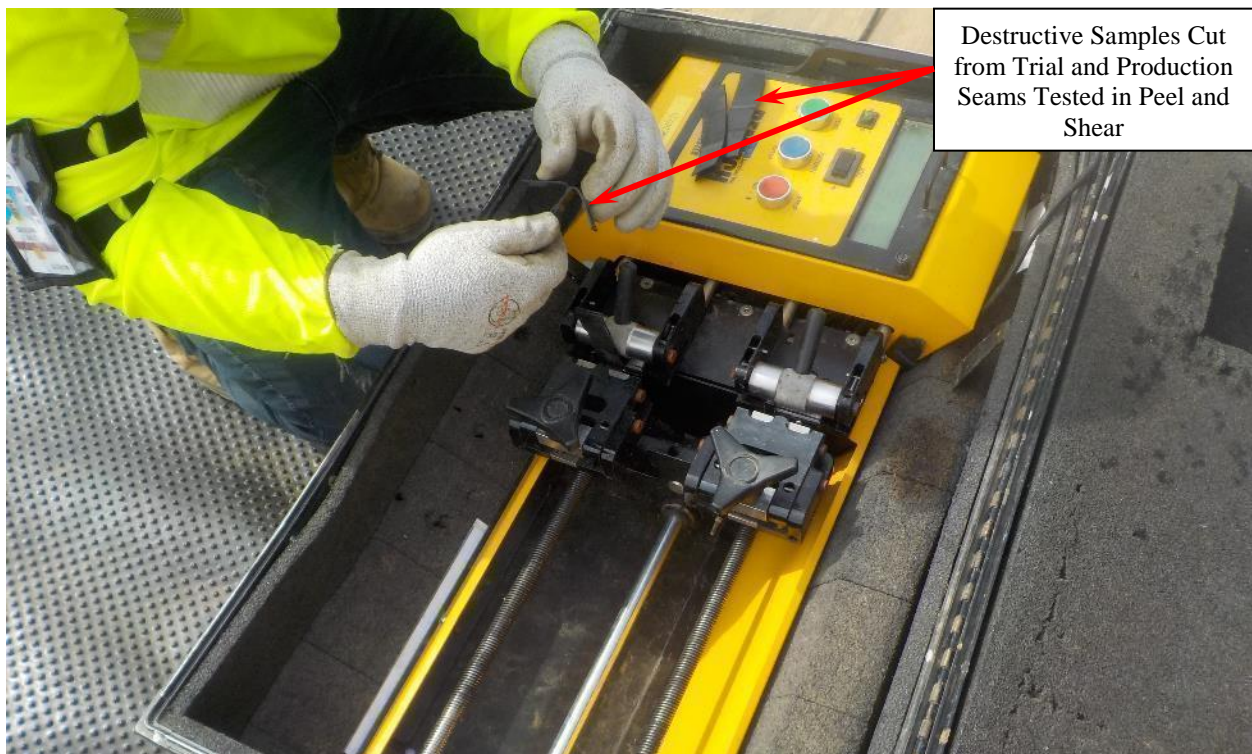
Photo 82. LLDPE Field Peel and Shear Testing (Destructive)
