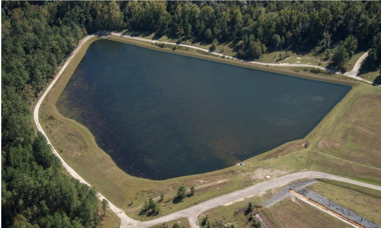
Photo 43. 489-D CPRB Aerial After Completion
