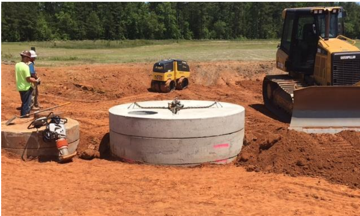
Photo 42. 489-D CPRB Backfilling in Progress
